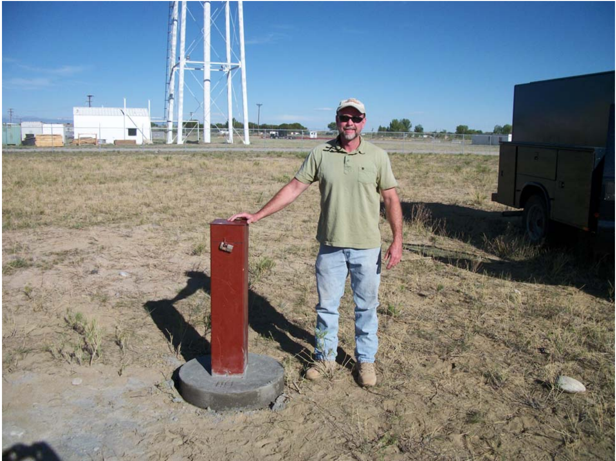
Upgrade of Monitoring Well 0110
