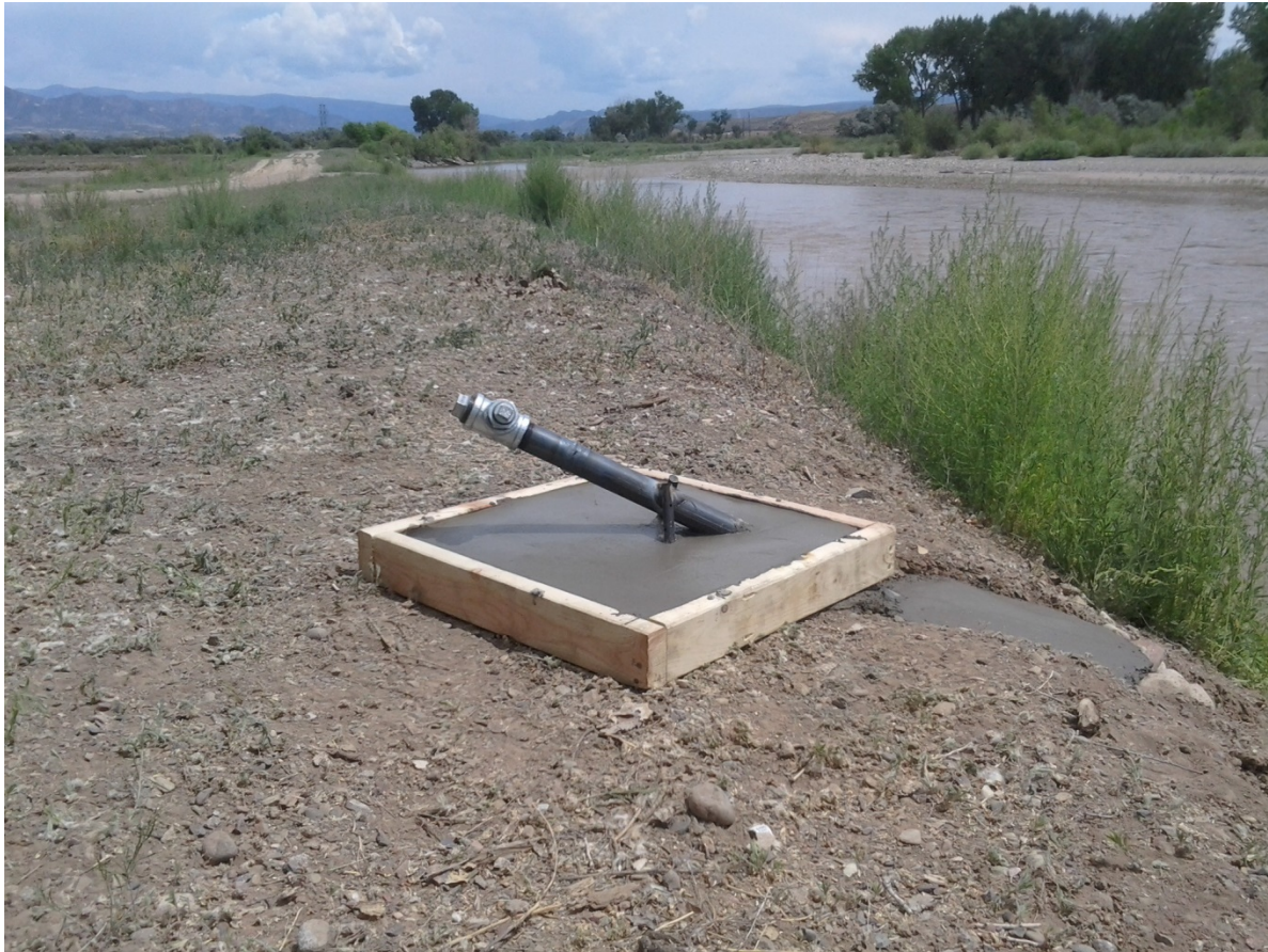
Figure 2. Example of Stilling Well Construction
