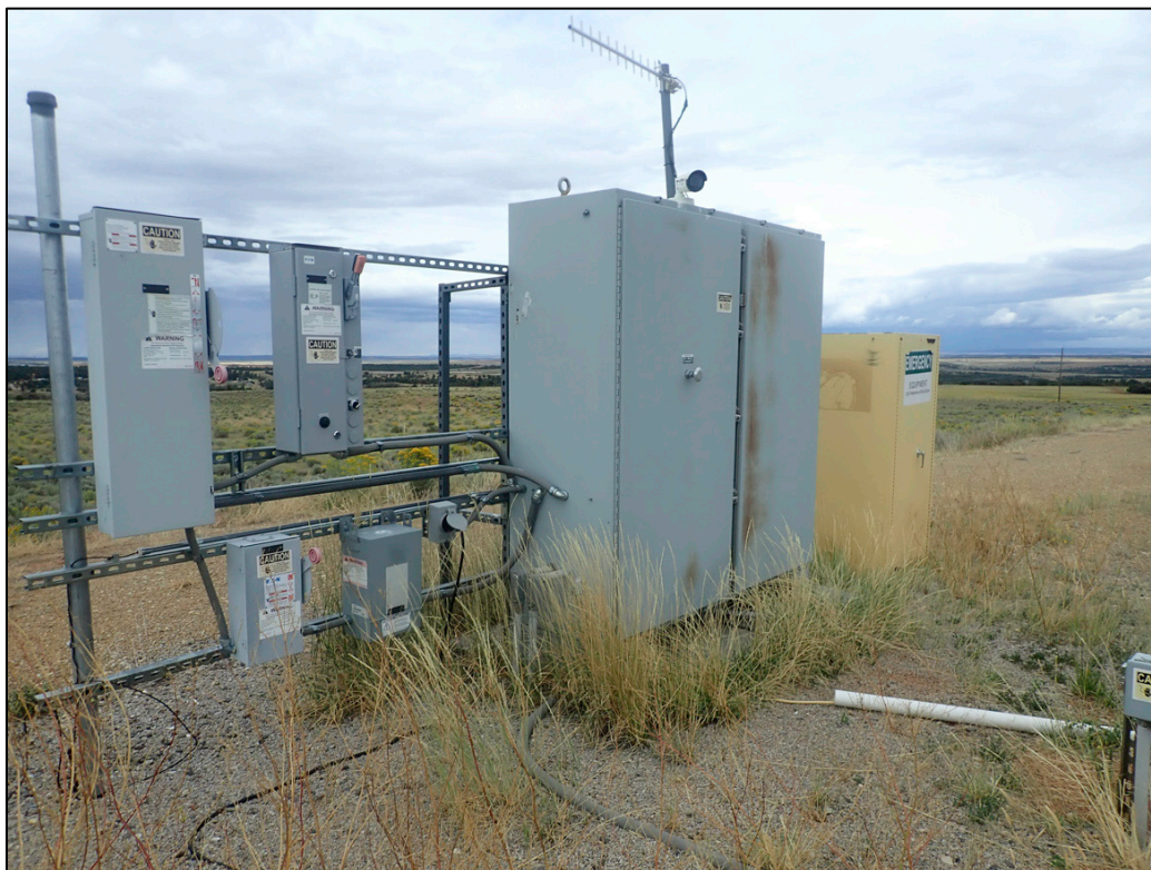
PL-15. Pond 4 LCRS and LDS Control Cabinet
