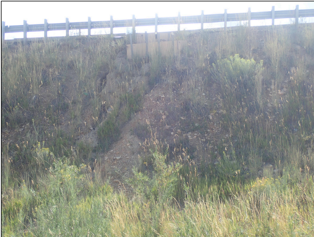
PL-30. UDOT Highway 191 Embankment Erosion
