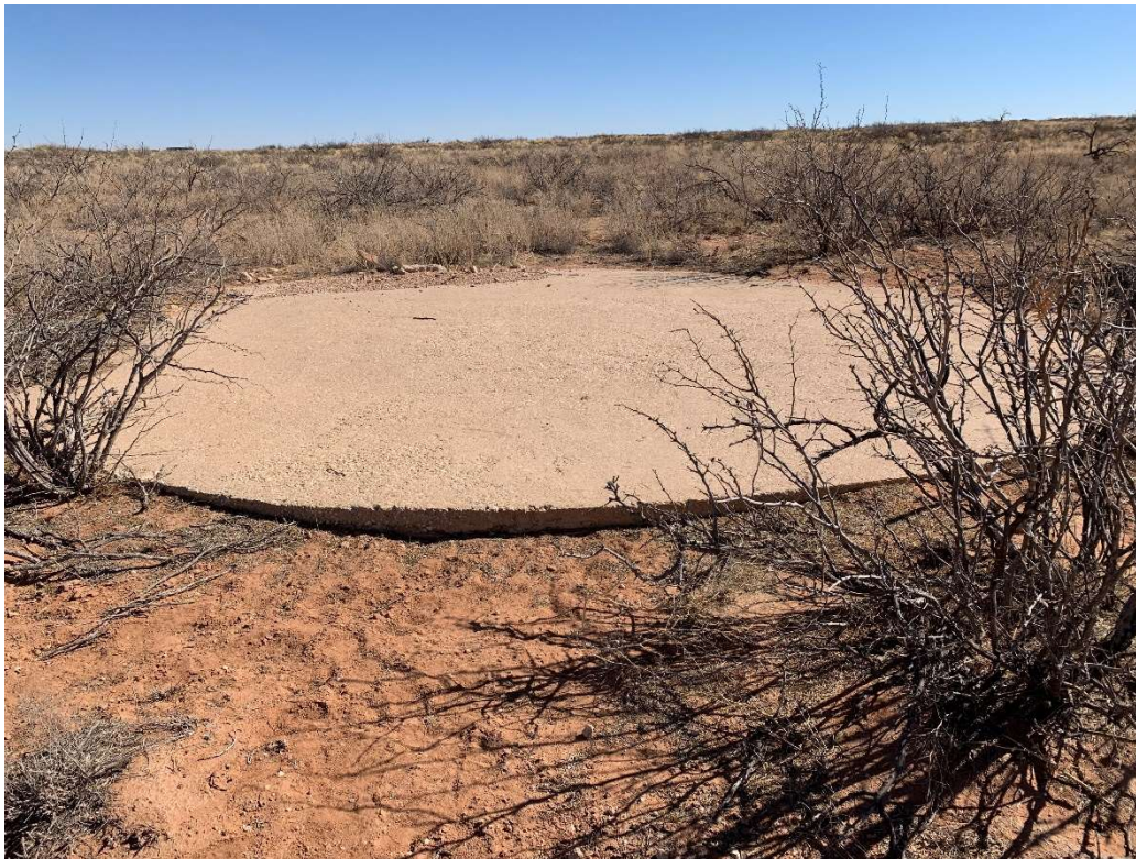
Photograph A-3. Looking East at the Concrete Cap That Covers the Project Gnome Emplacement Shaft
