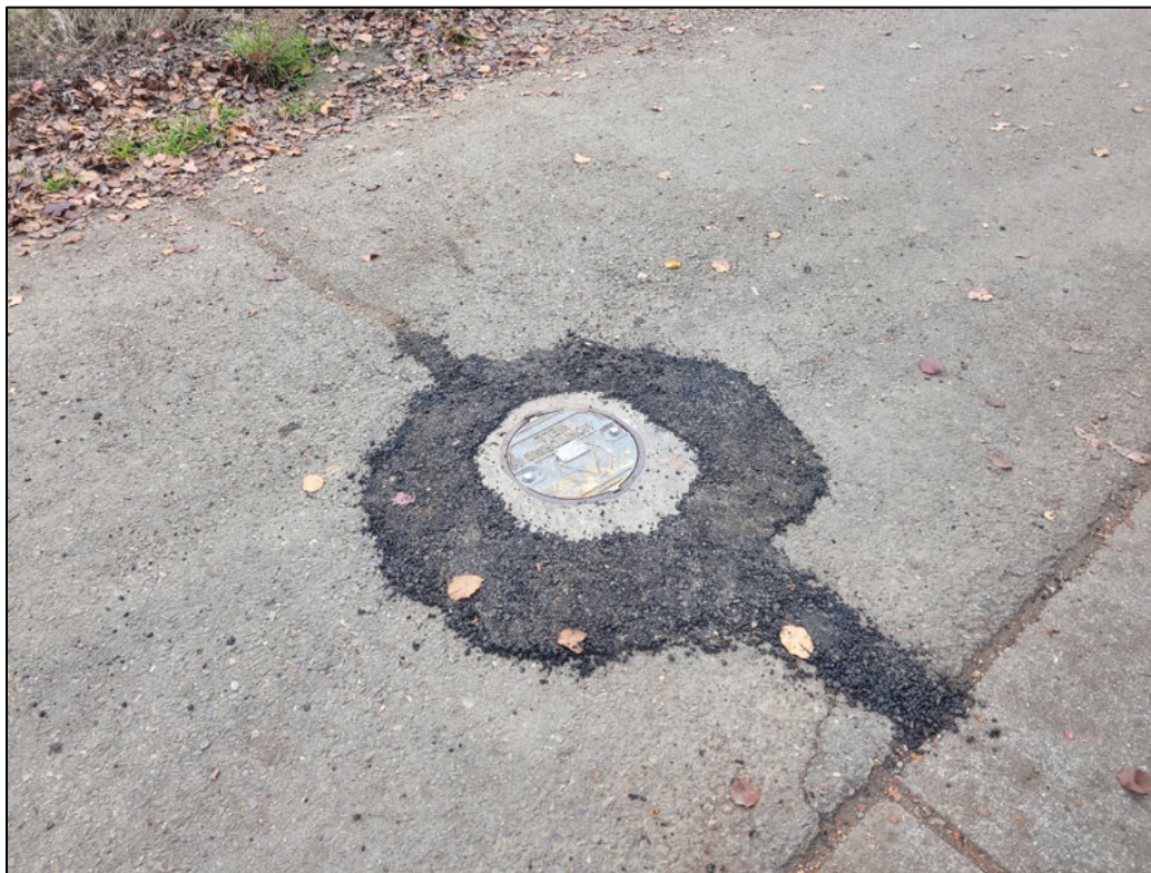
Photo F-5. Well UCD1-021: New Asphalt Patch Installed Surrounding Concrete Apron (UCD1-021 #1)
