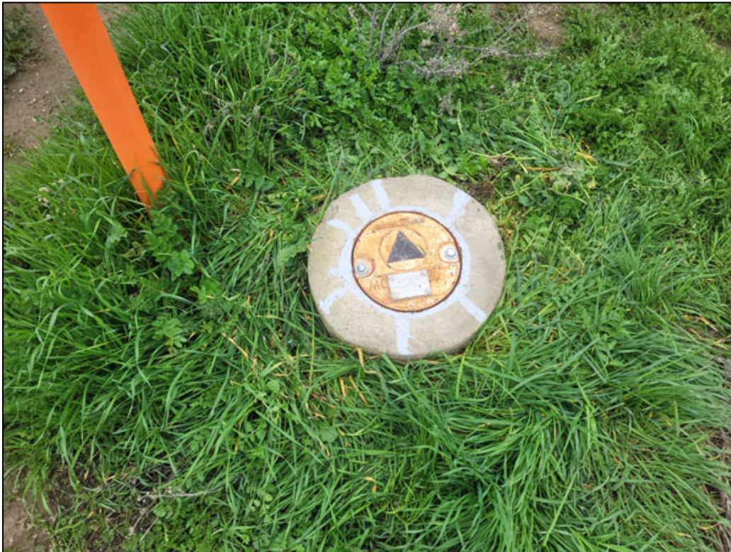
Photo F-6. Well UCD1-068: Cracks Patched in Concrete Apron (UCD1-068 #1)
