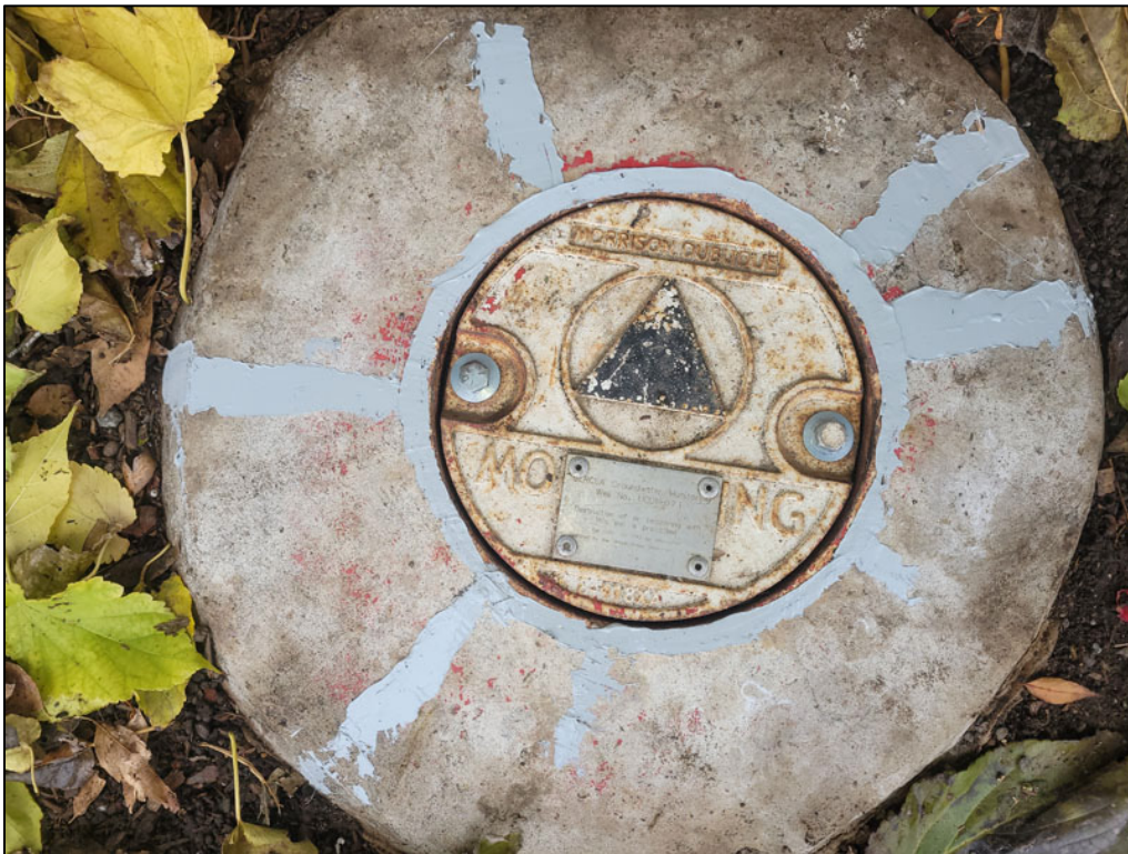
Photo F-11. Well UCD1-071: Seal Surfaces Cleaned, Seals Replaced, and Washers and Seals Installed on Bolts to Prevent Storm Water Entry (UCD1-071 #2)
