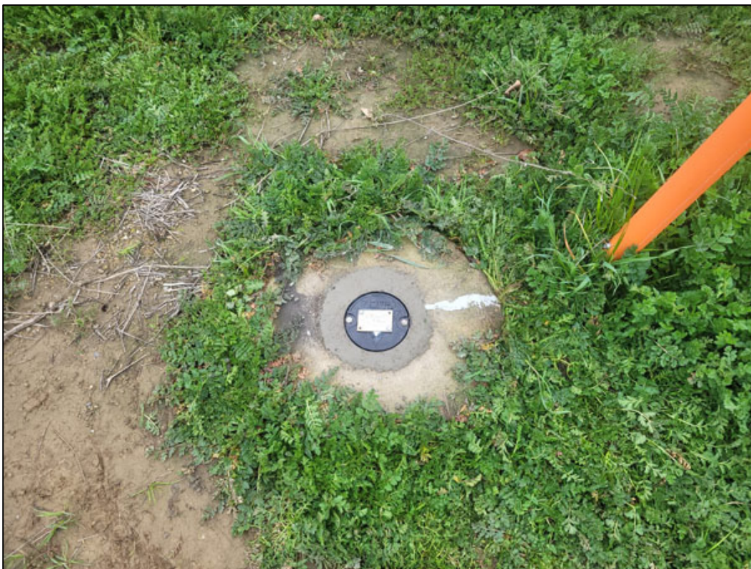
Photo F-4. Well UCD1-072: New Well Vault Installed (UCD1-072 #1)
