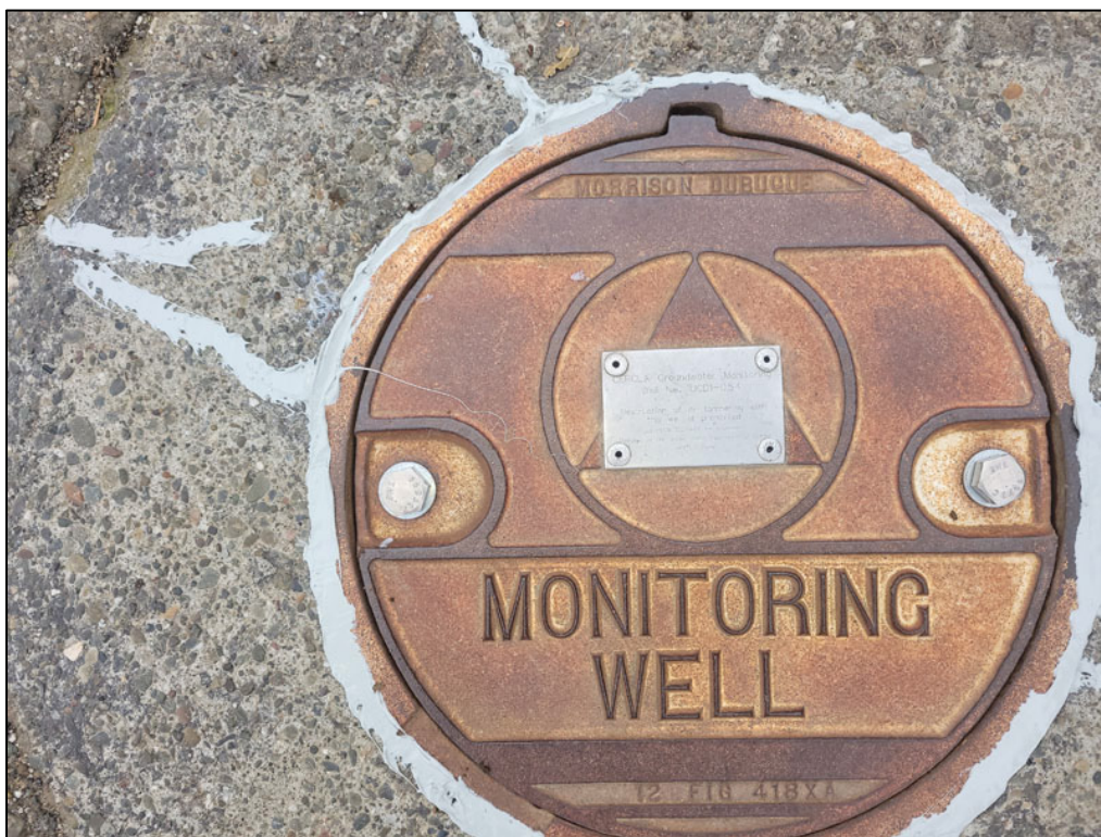
Photo F-8. Well UCD1-054: Seal Surfaces Cleaned, Seals Replaced, and Washers and Seals Installed on Bolts to Prevent Storm Water Entry (UCD1-054 #2)
