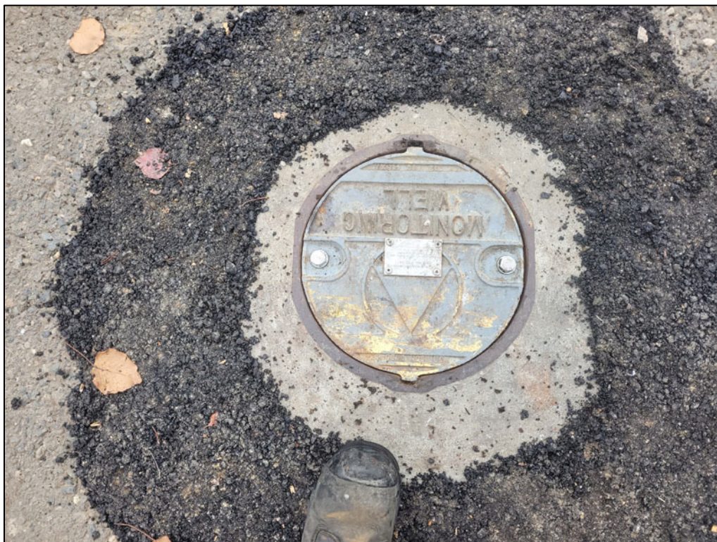
Photo F-7. Well UCD1-021: Seal Surfaces Cleaned, Seals Replaced, and Washers and Seals Installed on Bolts to Prevent Storm Water Entry (UCD1-021 #2)
