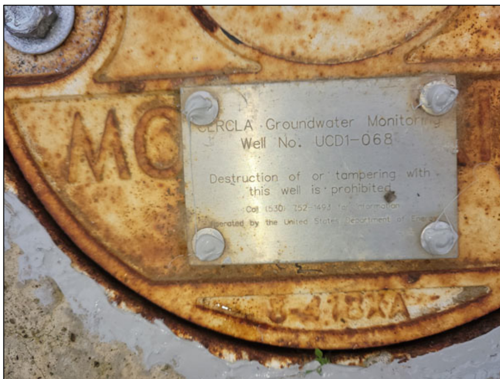
Photo F-9. Well UCD1-068: Seal Surfaces Cleaned, Seals Replaced, and Washers and Seals Installed on Bolts to Prevent Storm Water Entry (UCD1-068 #2)
