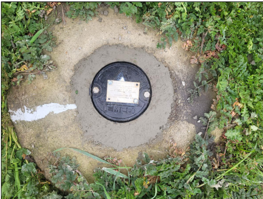
Photo F-12. Well UCD1-072: Seal Surfaces Cleaned, Seals Replaced, and Washers and Seals Installed on Bolts to Prevent Storm Water Entry (UCD1-072 #2)
