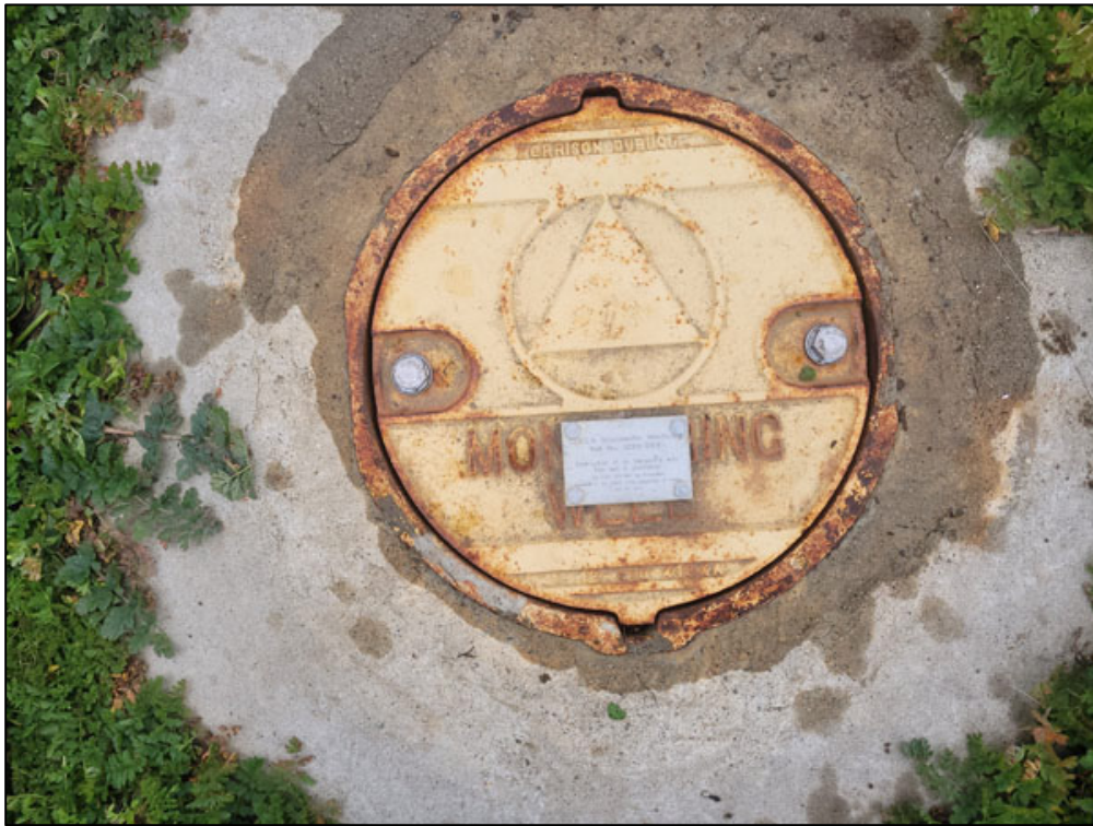
Photo F-10. Well UCD1-069: Seal Surfaces Cleaned, Seals Replaced, and Washers and Seals Installed on Bolts to Prevent Storm Water Entry (UCD1-069 #2)
