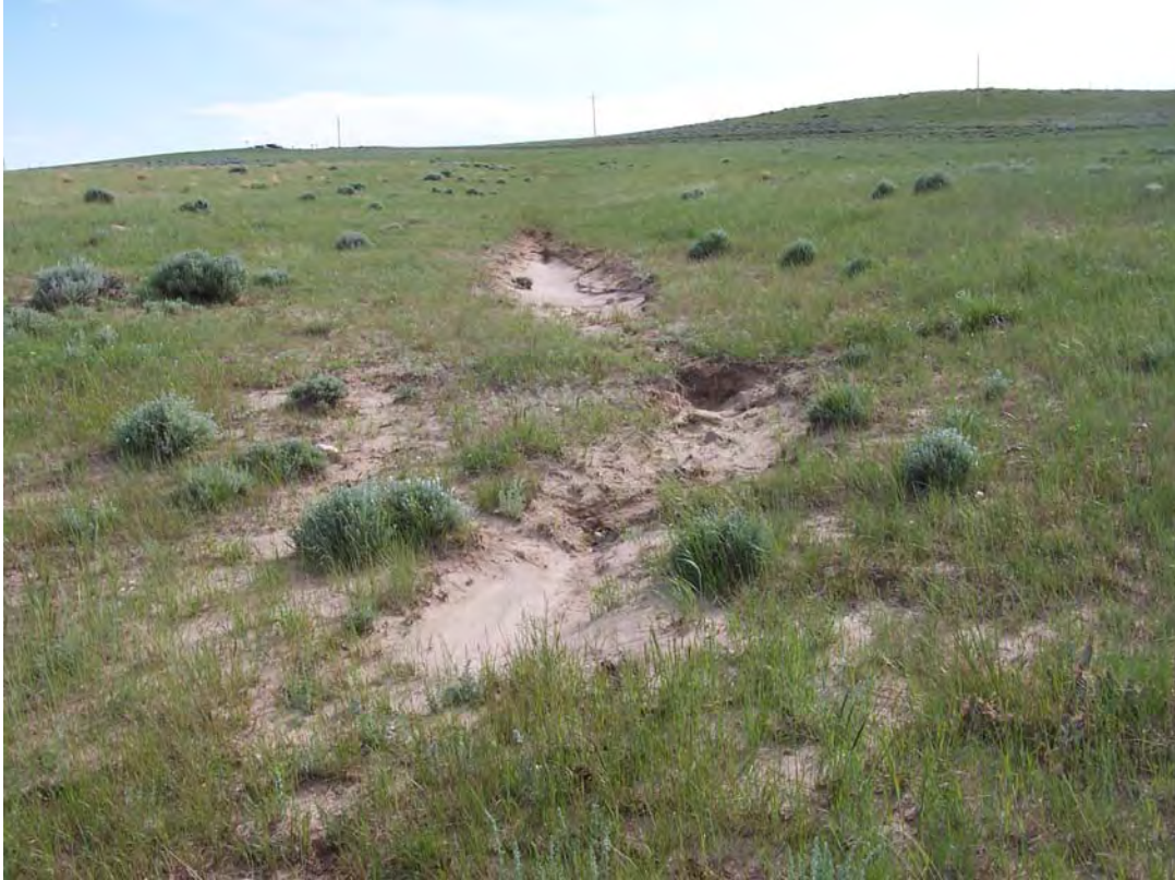
SPK 6/2008. PL-3. Stable erosion area near the northwest edge of the disposal cell.
