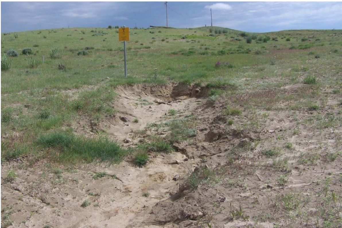
SPK 6/2007. PL-4. Gully adjacent to perimeter sign P4; minor change from 2006.
