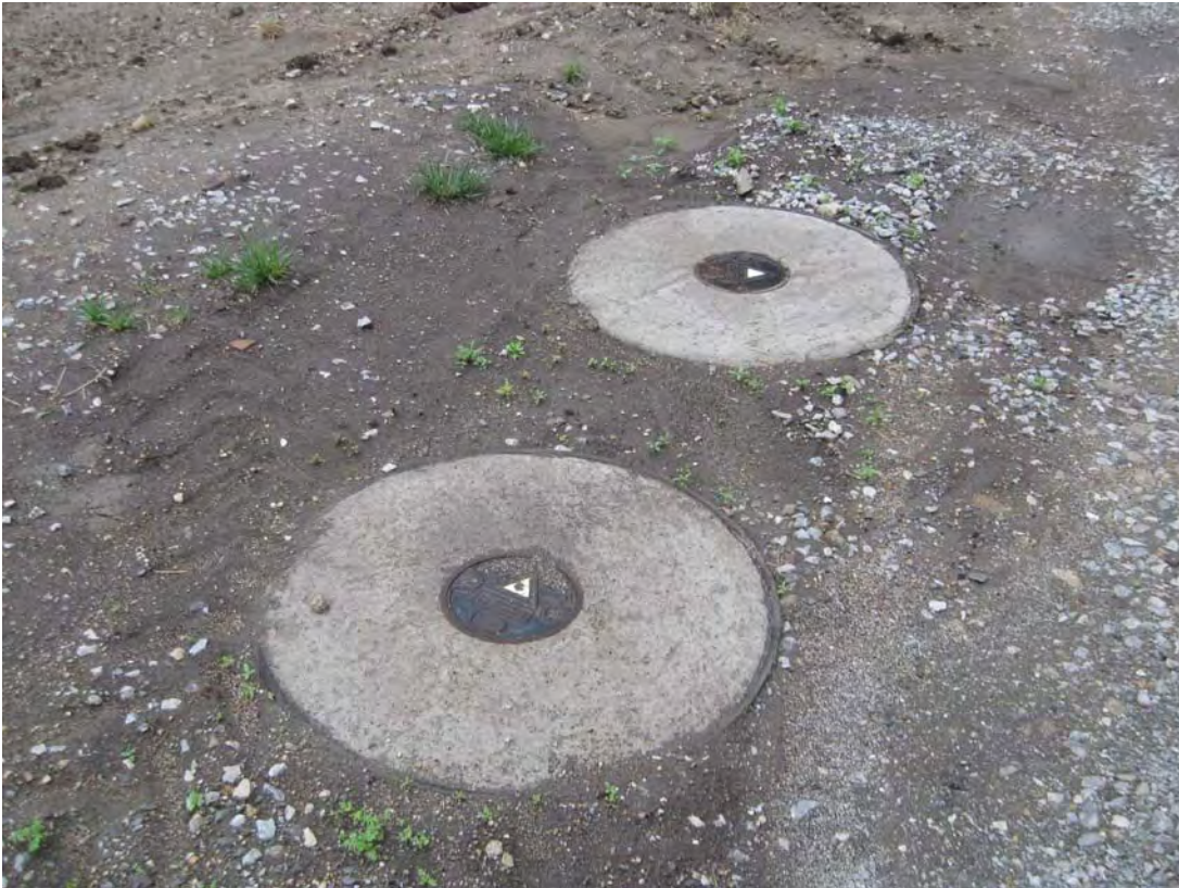
HAL 4/2009. PL-9. Newly installed flush mount wells 1A and 1B.
