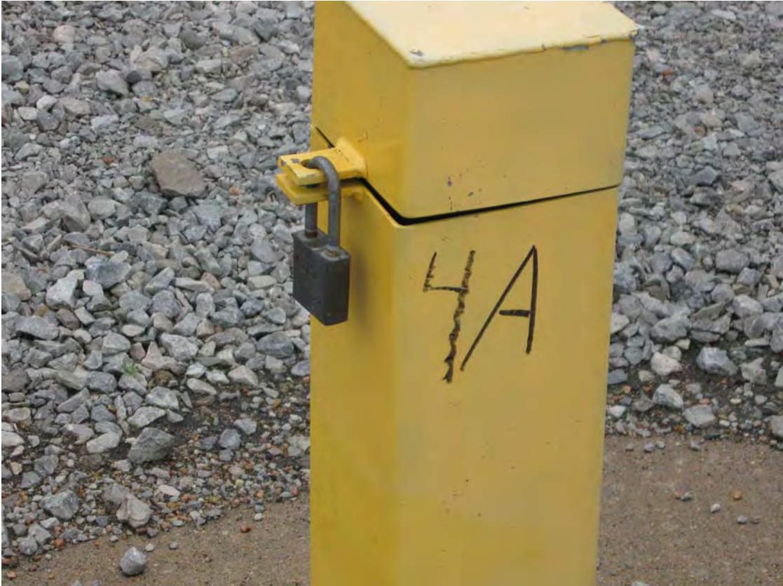
HAL 4/2009. PL-8. Monitor well 4-A clearly labeled on outside of protective casing.
