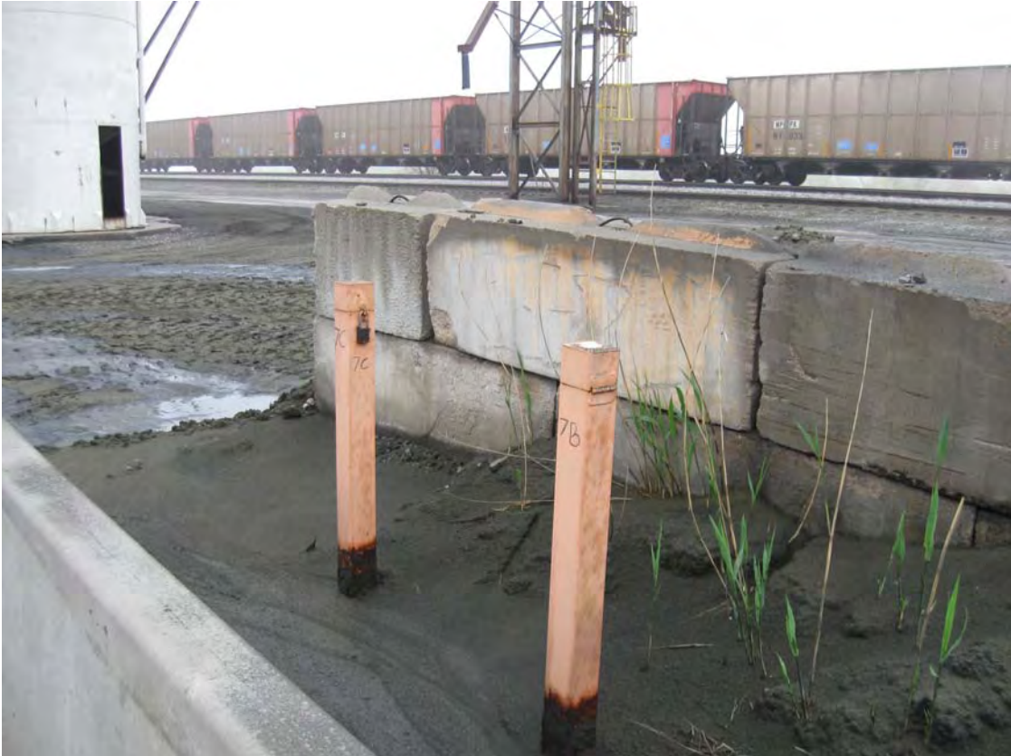
HAL 4/2009. PL-14. New concrete barriers around well cluster 7.
