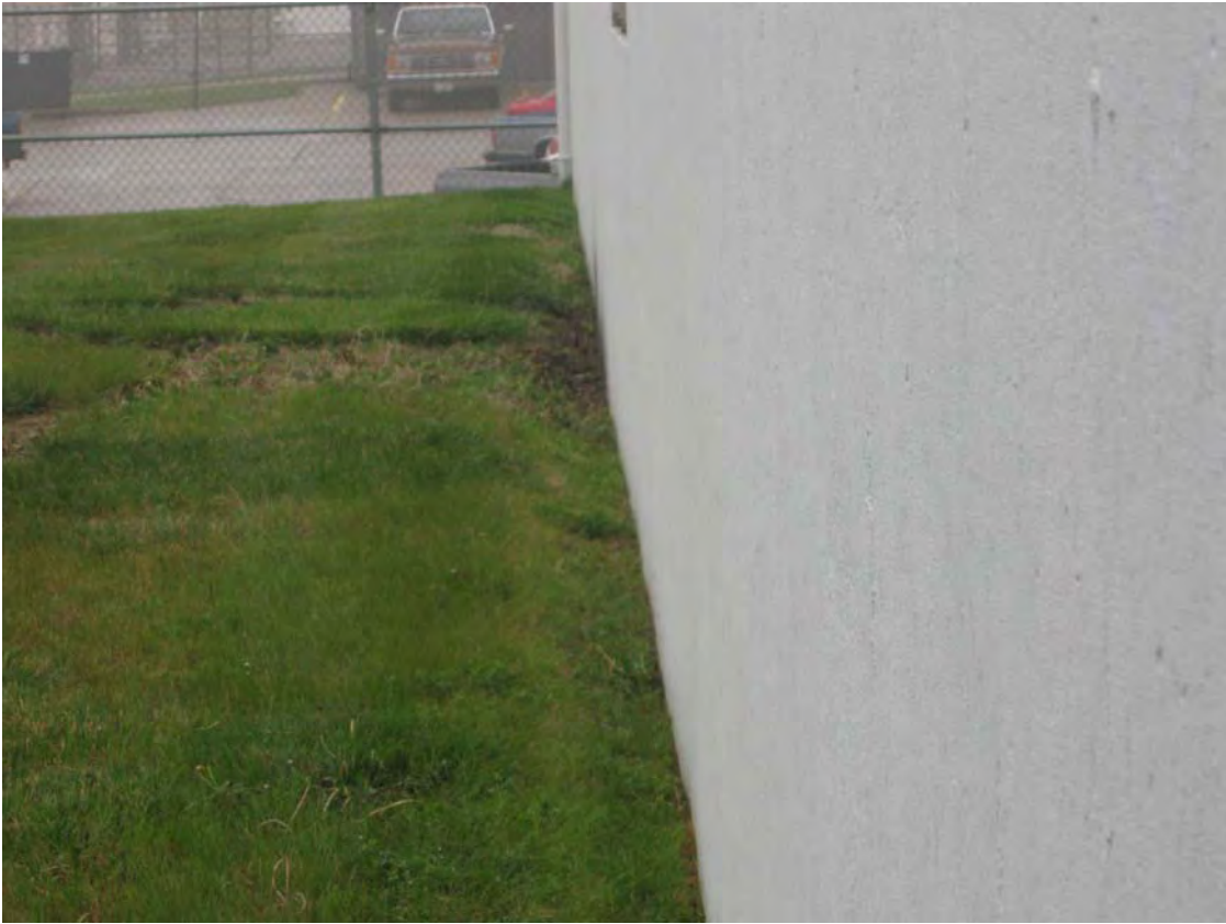
HAL 4/2009. PL-5. Soil at the base of the south wall of the IHX is sloped toward the building.
