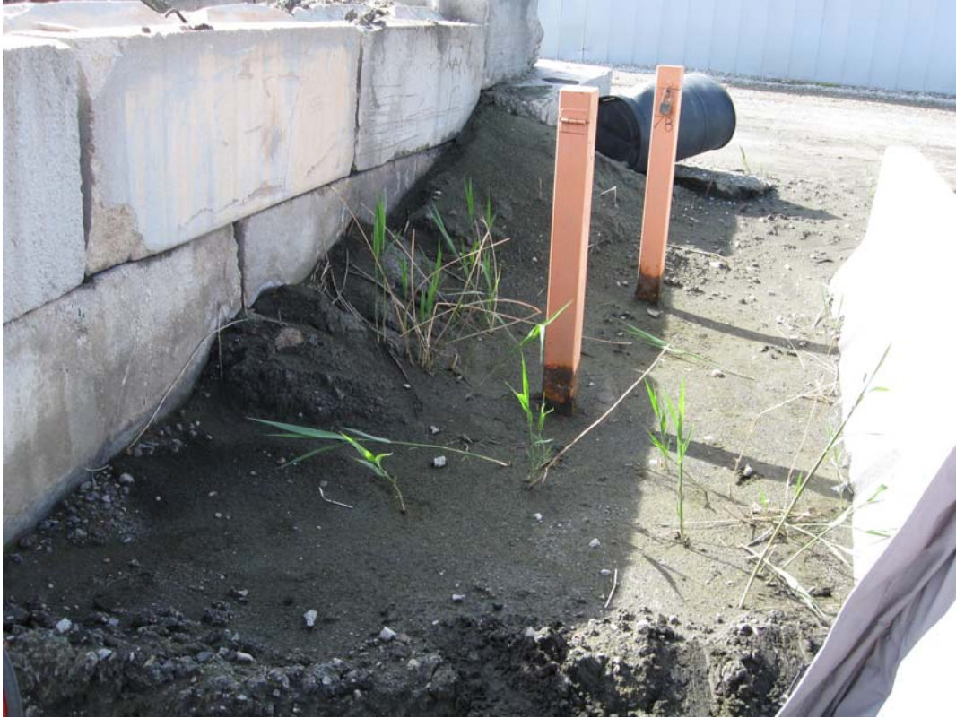
HAL 4/2010. PL-11. Monitoring wells OBS-7B and OBS-7C. Protected on east and west by concrete barriers. Well pad covered by coal dust.
