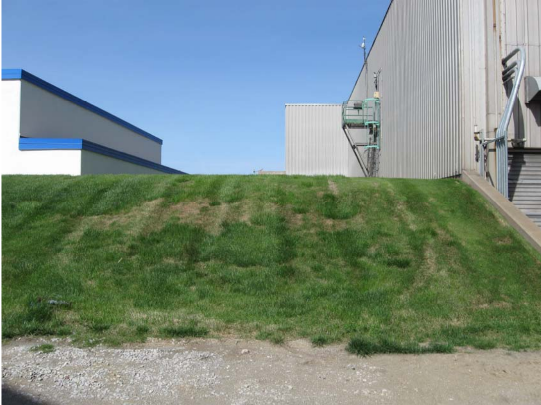
HAL 4/2010. PL-5. Grass-covered mound east of the IHX building.
