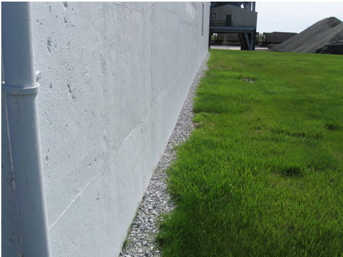
HAL 4/2010. PL-2. Gravel along the base of the south side of the IHX building.
