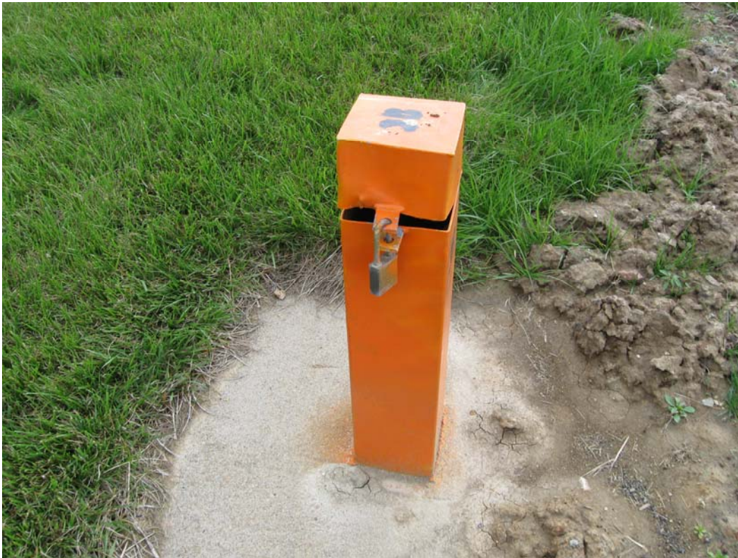
HAL 4/2011. PL-8. Monitoring Well OBS-3B.
