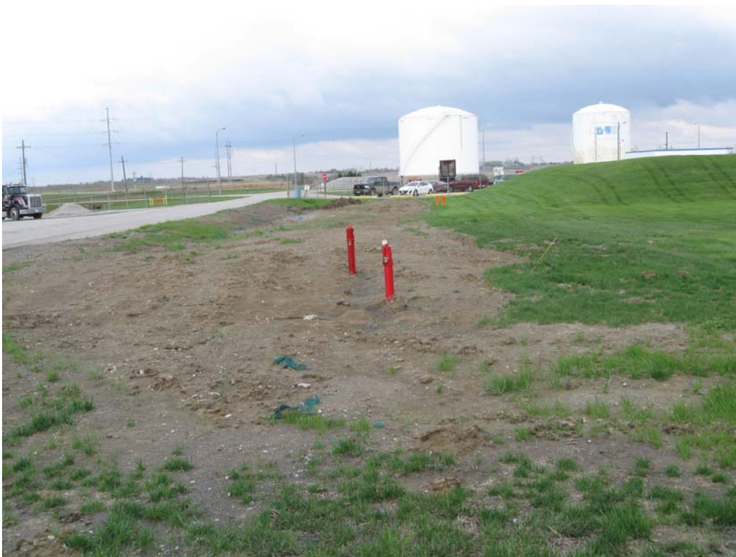
HAL 4/2011. PL-3. South end of grass covered mound. New grass seeding needed.
