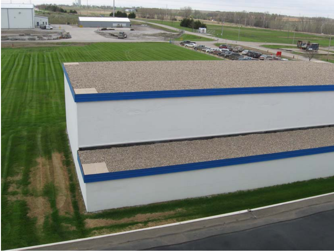
HAL 4/2011. PL-1. Roof of IHX building.
