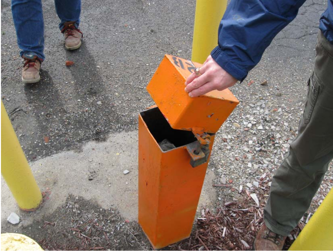
HAL 4/2011. PL-7. Monitoring Well OBS-2B. Hinge placement allows well cap to partially open when locked.
