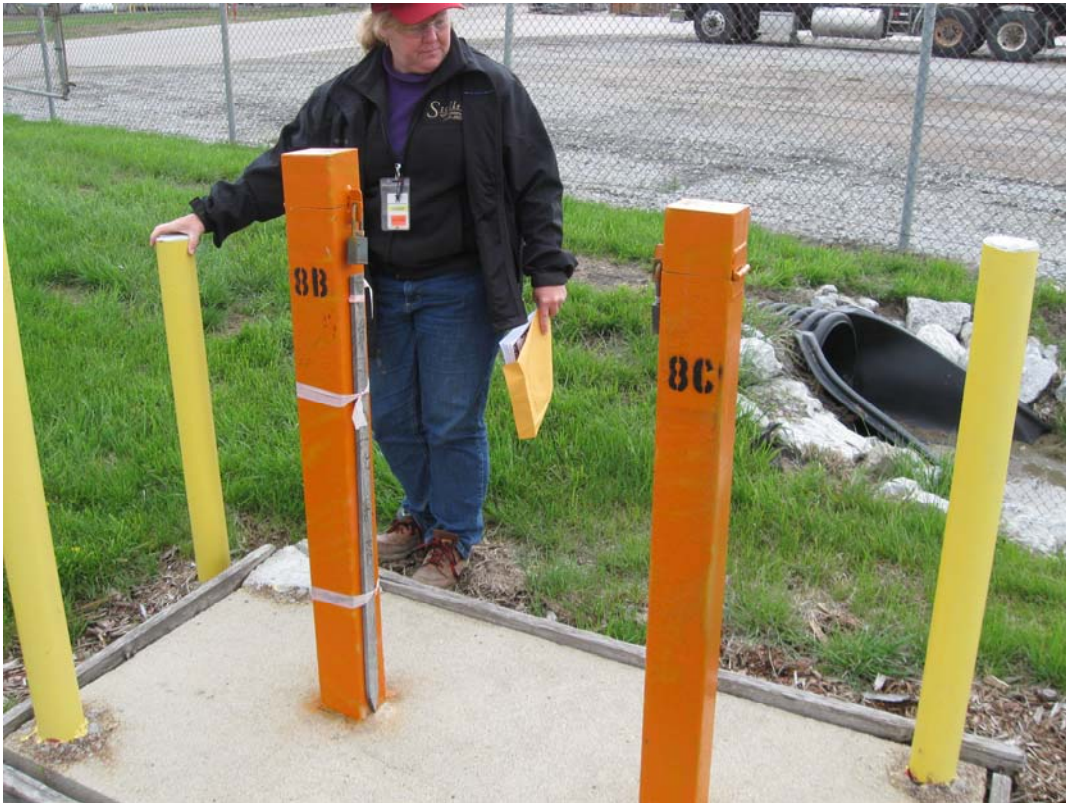
HAL 4/2011. PL-6. Monitoring Wells OBS-8B and OBS-8C.
