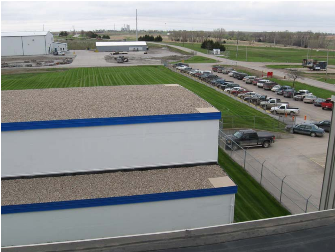
HAL 4/2011. PL-2. Roof of IHX building.
