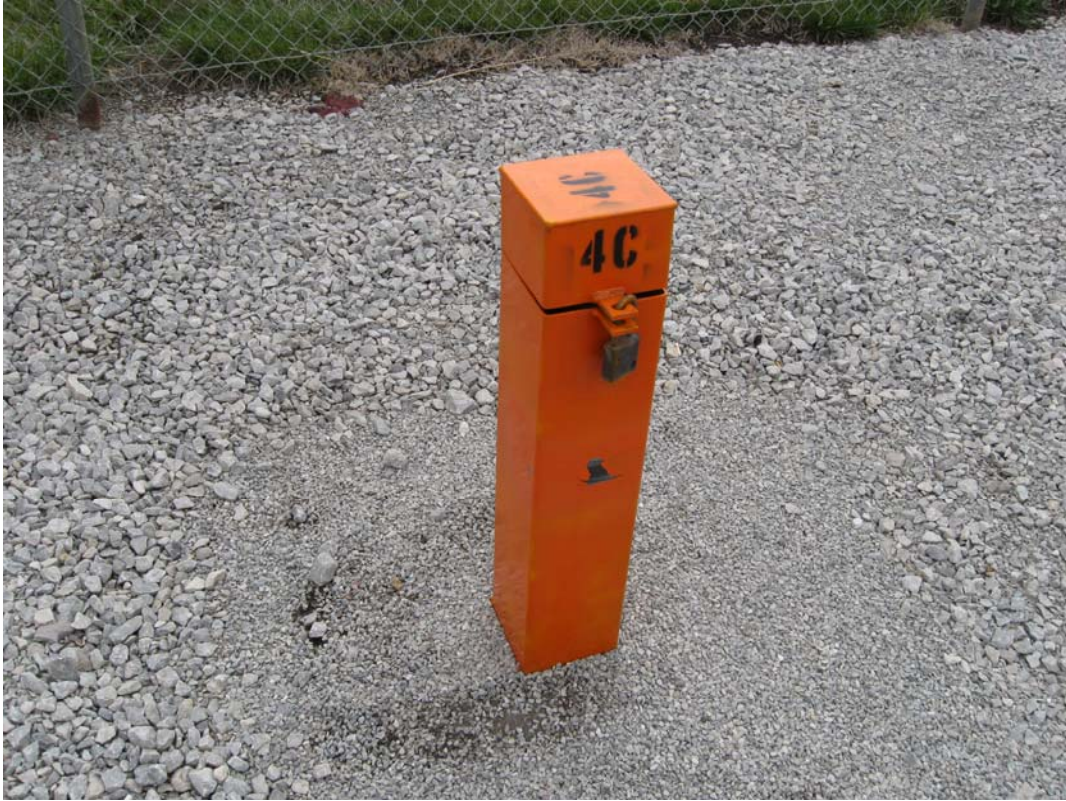
HAL 4/2011. PL-5. Monitoring Well OBS-4C.
