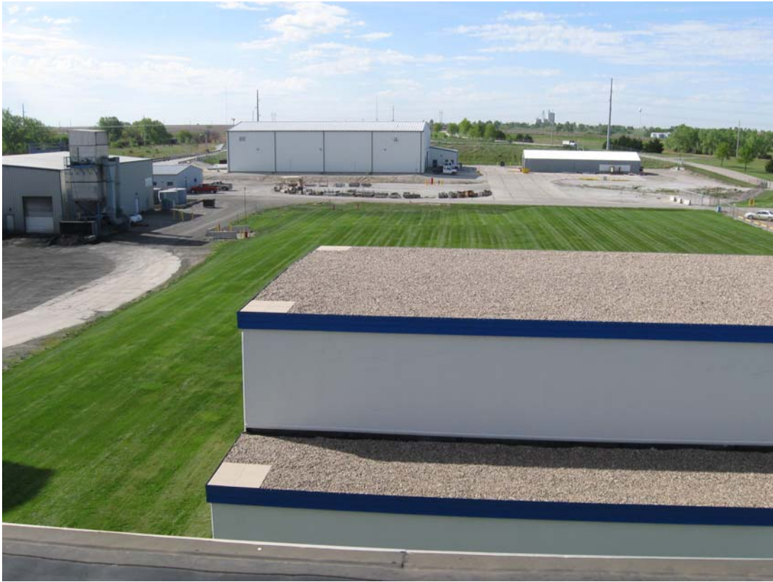
HAL 4/2012. PL-1. Northeast corner of IHX roof.
