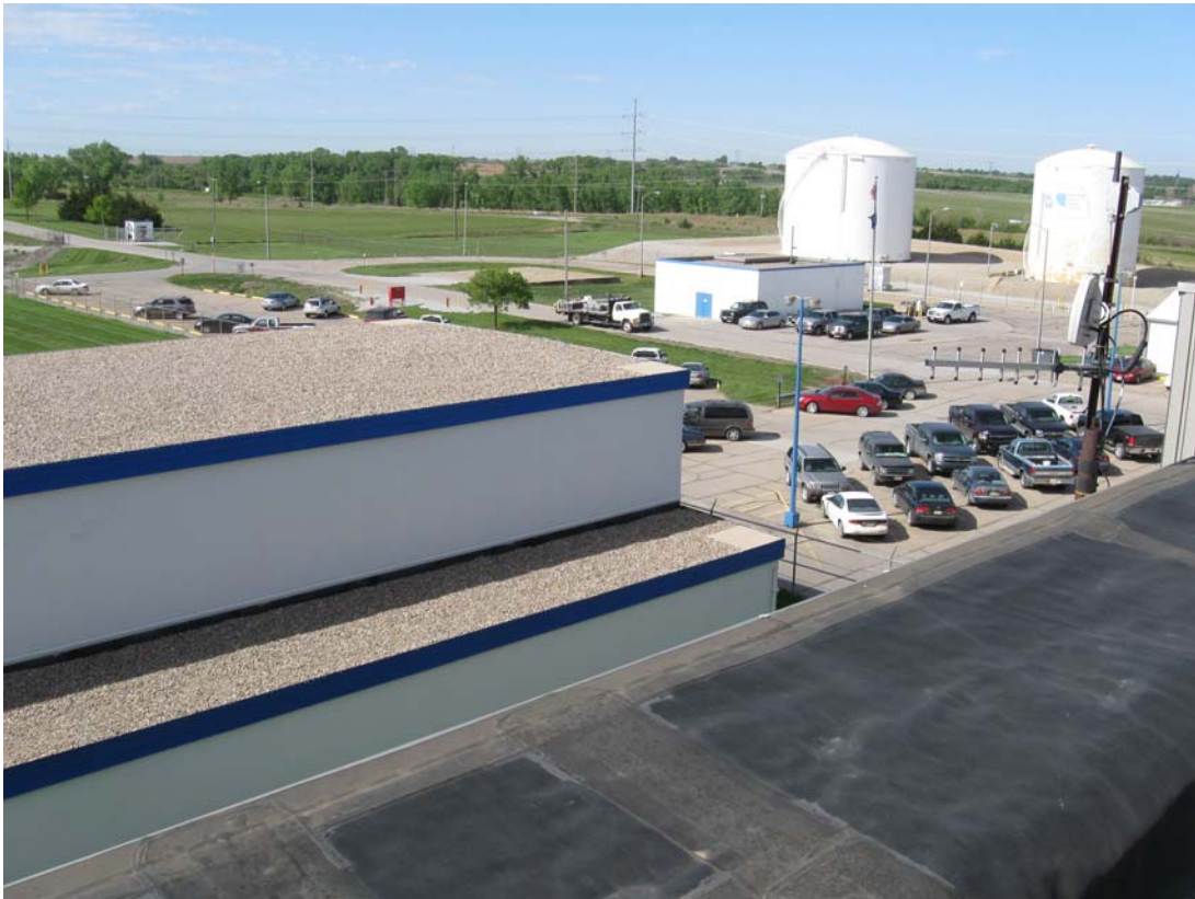
HAL 4/2012. PL-2. West end of IHX roof.
