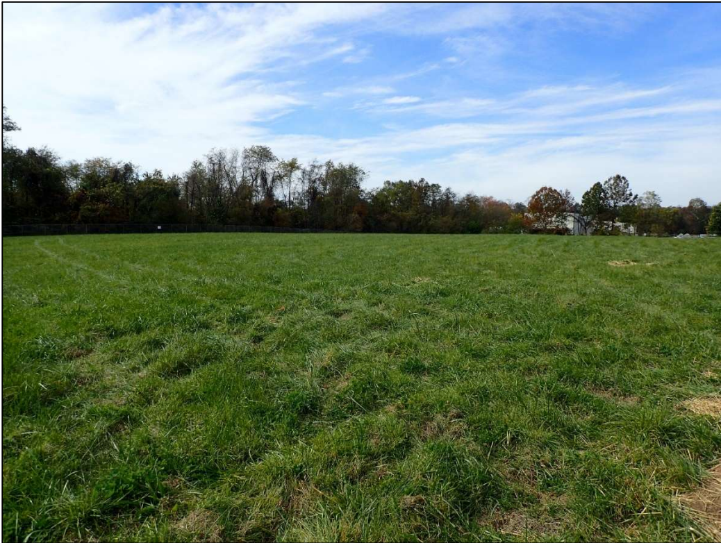
PL-6. Top of Disposal Cell
