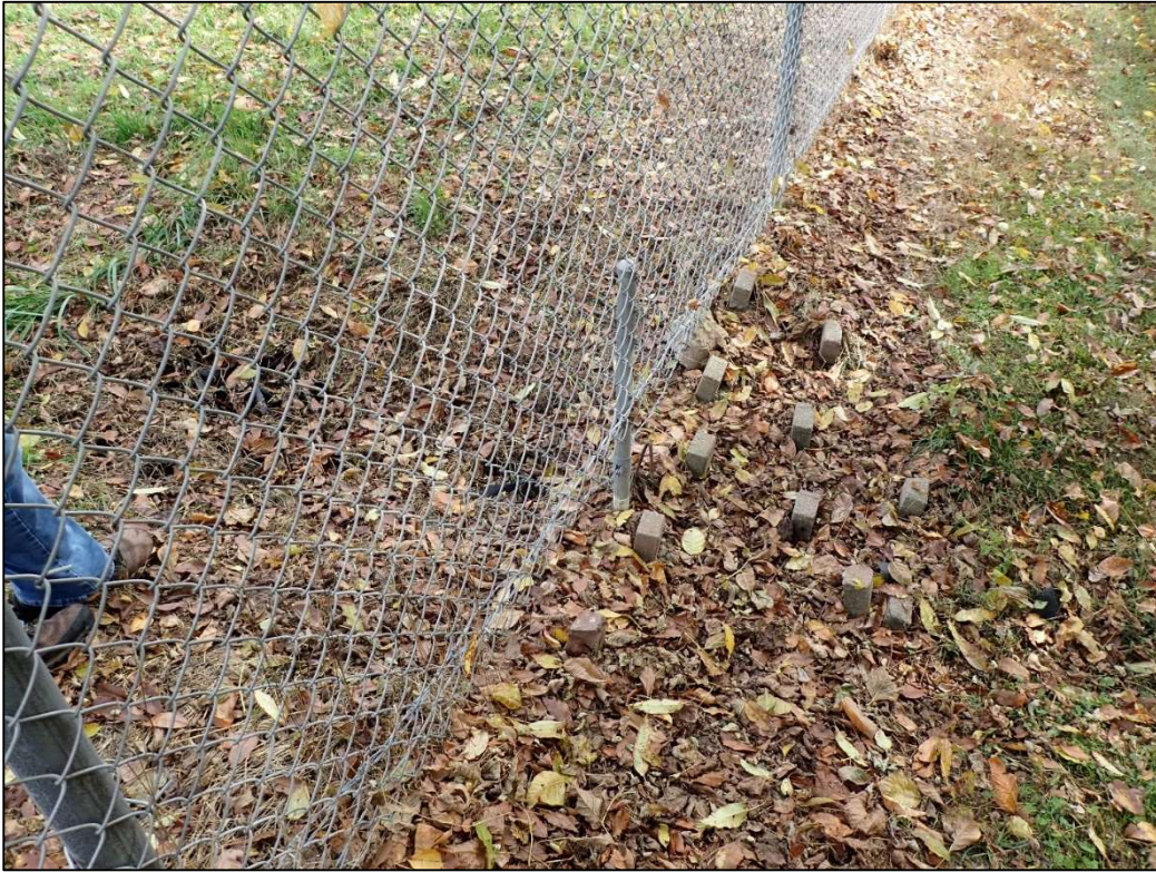
PL-9. Erosion Control Area
