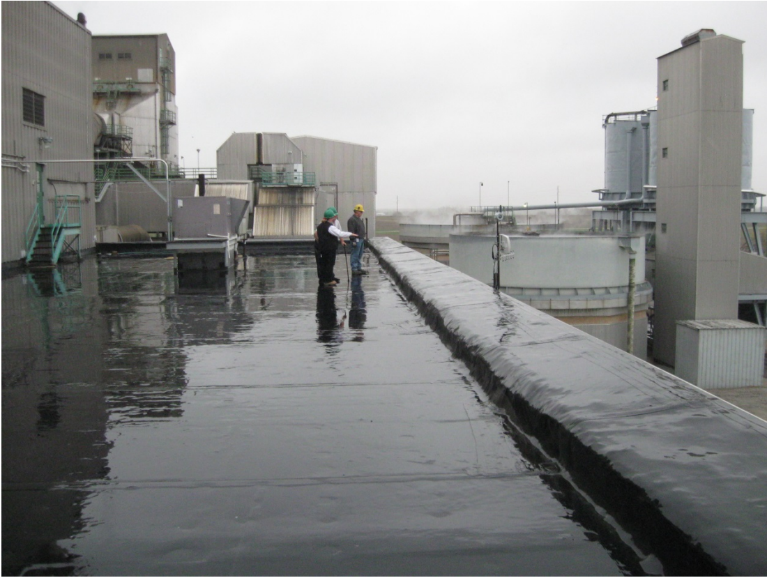
HAL 4/2013. PL-1. Roof of Power Plant building.
