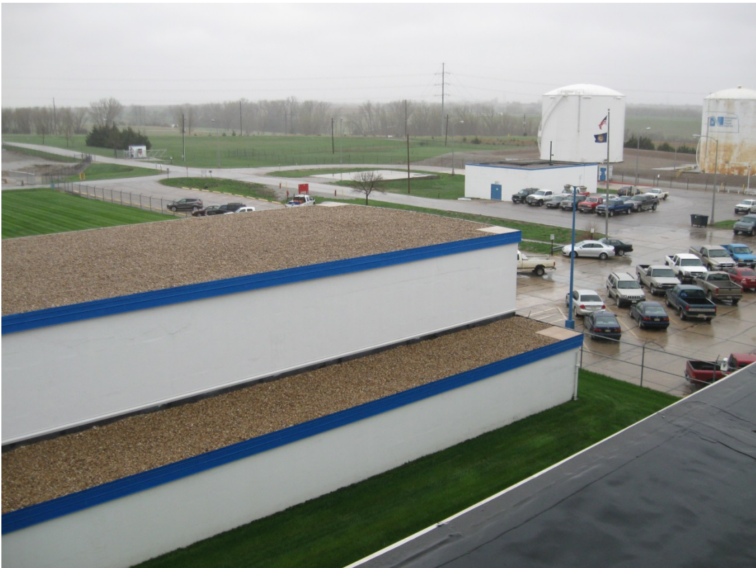
HAL 4/2013. PL-2. Roof of IHX building.
