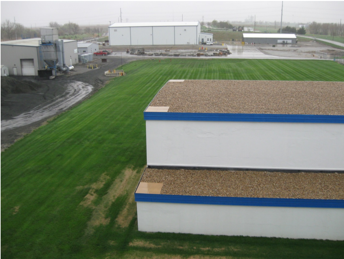
HAL 4/2013. PL-3. Roof, east half of IHX building.
