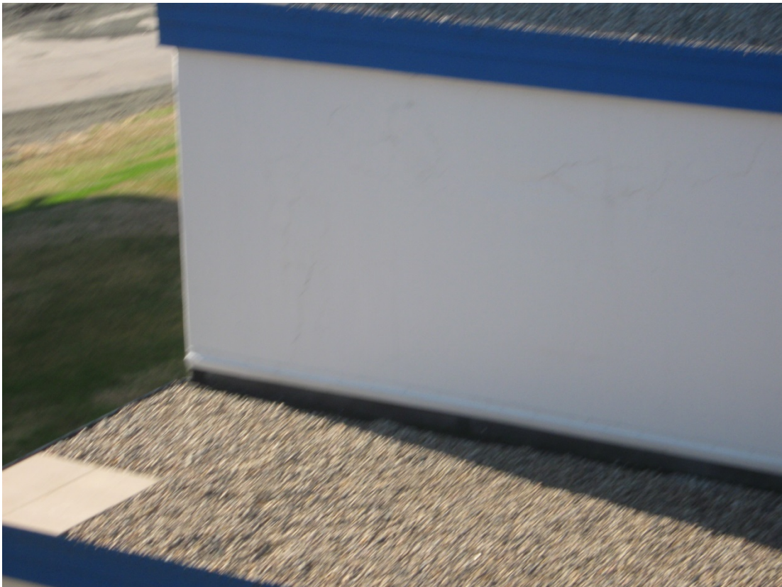
HAL 4/2014. PL-2. Northeast corner of lower IHX Building.
