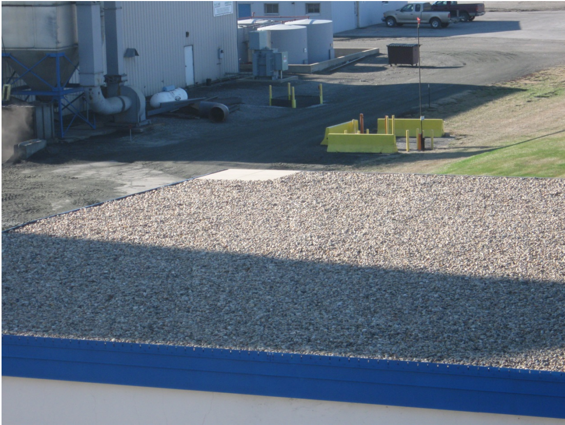
HAL 4/2014. PL-3. Southeast corner of upper IHX Building.
