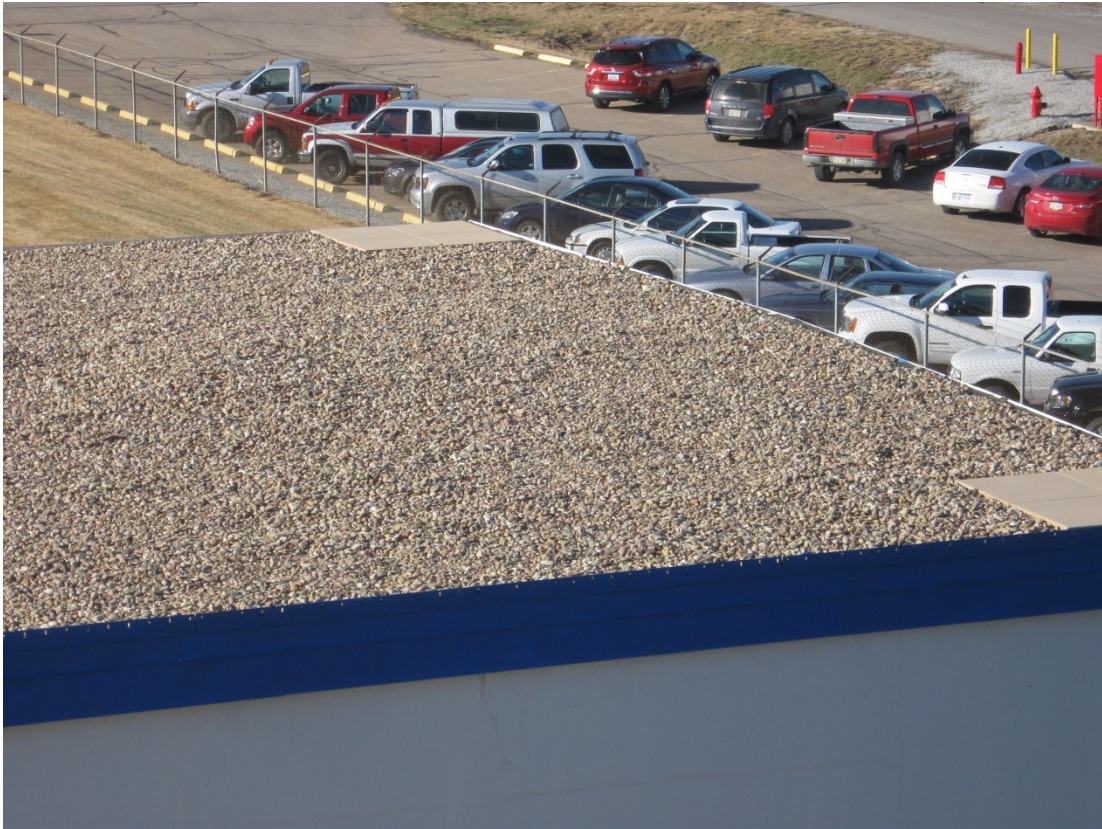
HAL 4/2014. PL-1. West Edge of Upper IHX building roof.
