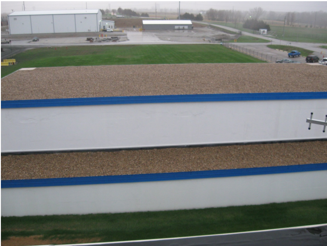
HAL 4/2015. PL-2. IHX building roof.
