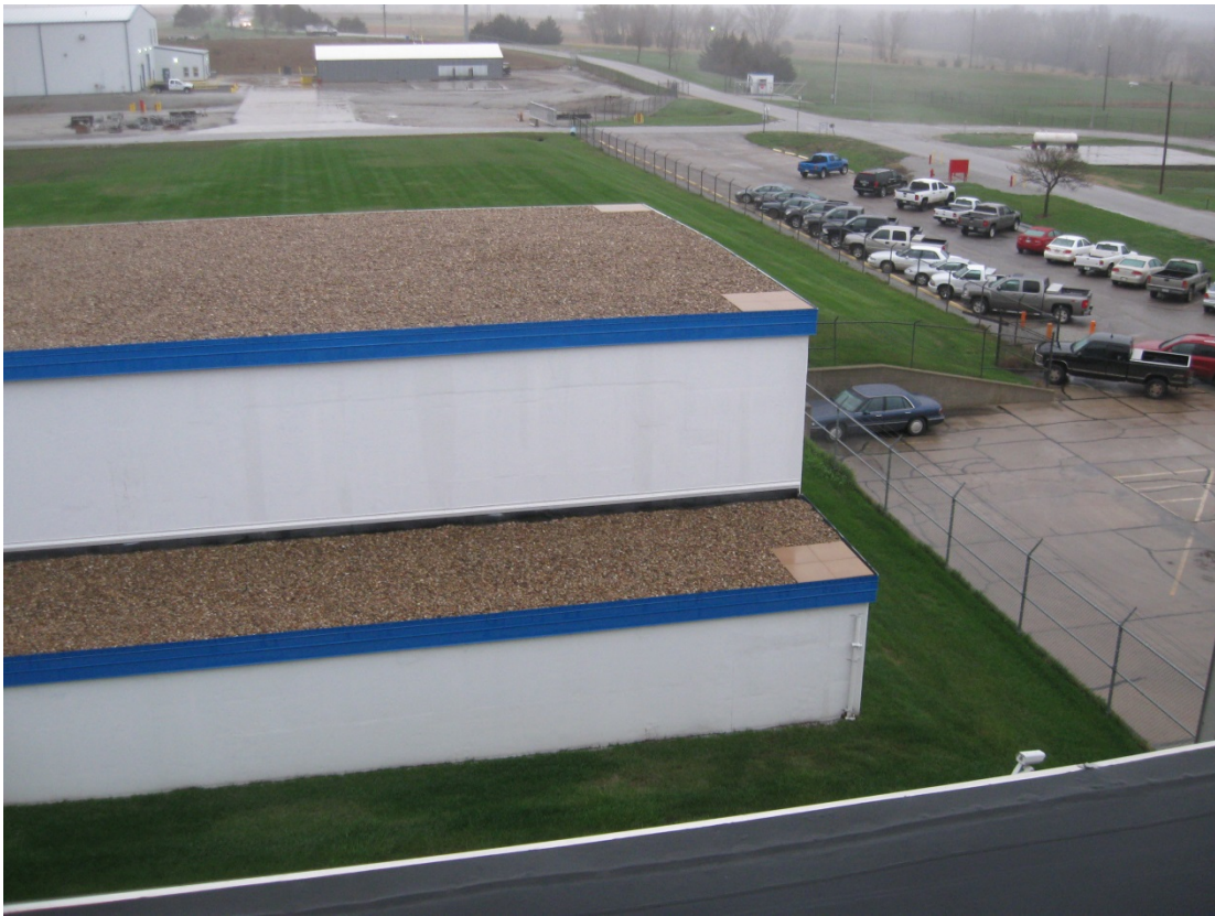
HAL 4/2015. PL-3. West end of IHX building roof.
