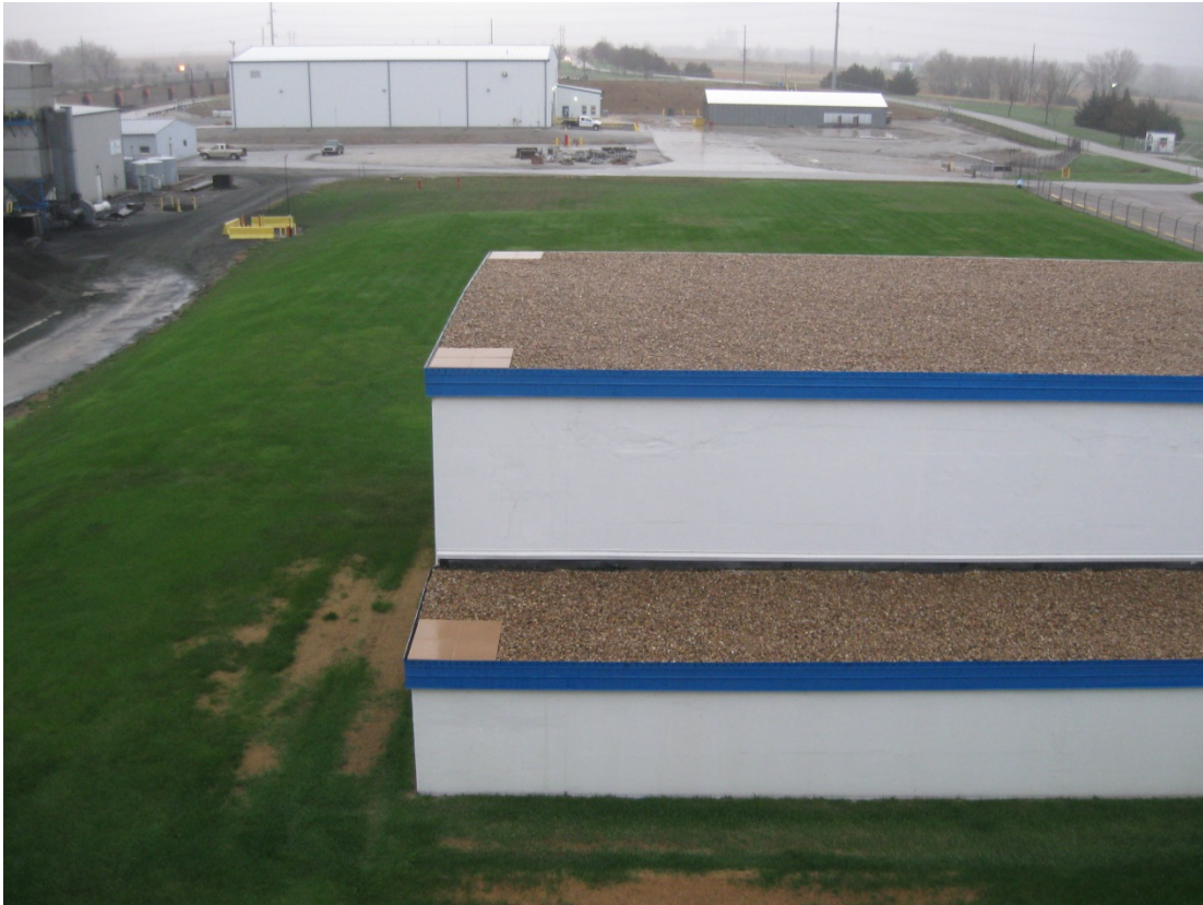
HAL 4/2015. PL-1. East end of IHX Building roof.
