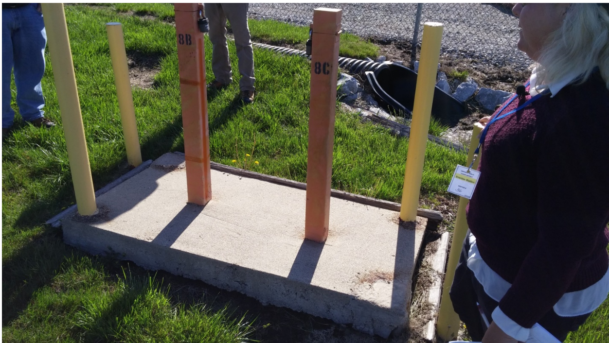
HAL 4/2016. PL-8. Slight erosion around base of OBS-8 well pad.
