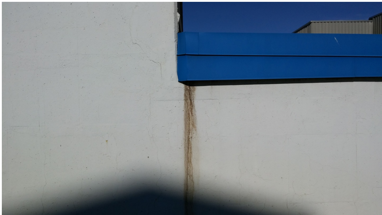
HAL 4/2016. PL-3. Water staining on east wall of IHX building.
