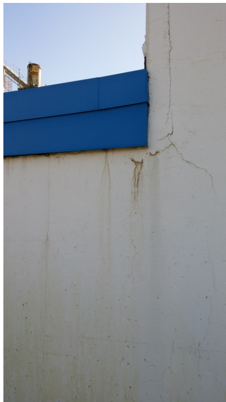
HAL 4/2016. PL-4. Surface cracks on west wall of IHX building.
