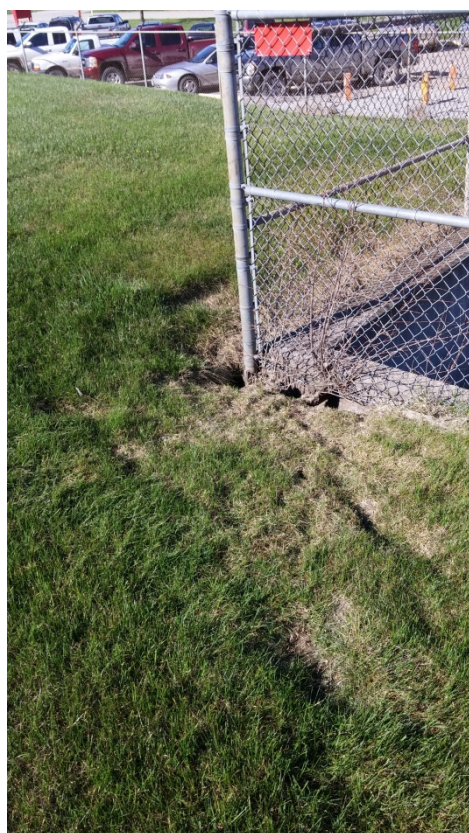
HAL 4/2016. PL-6. Erosion at base of fence.
