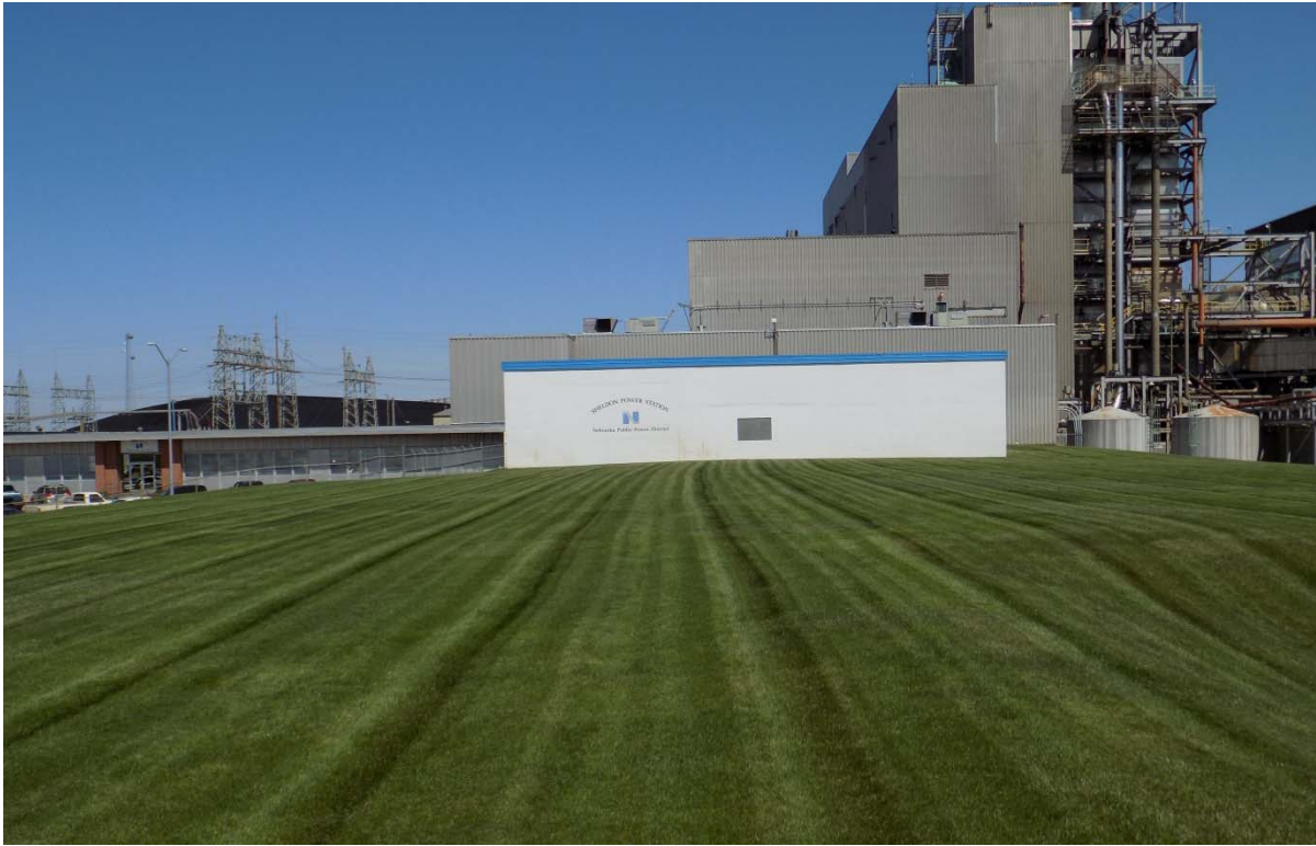
PL-7. View North from South Edge of Grass-Covered Mound
