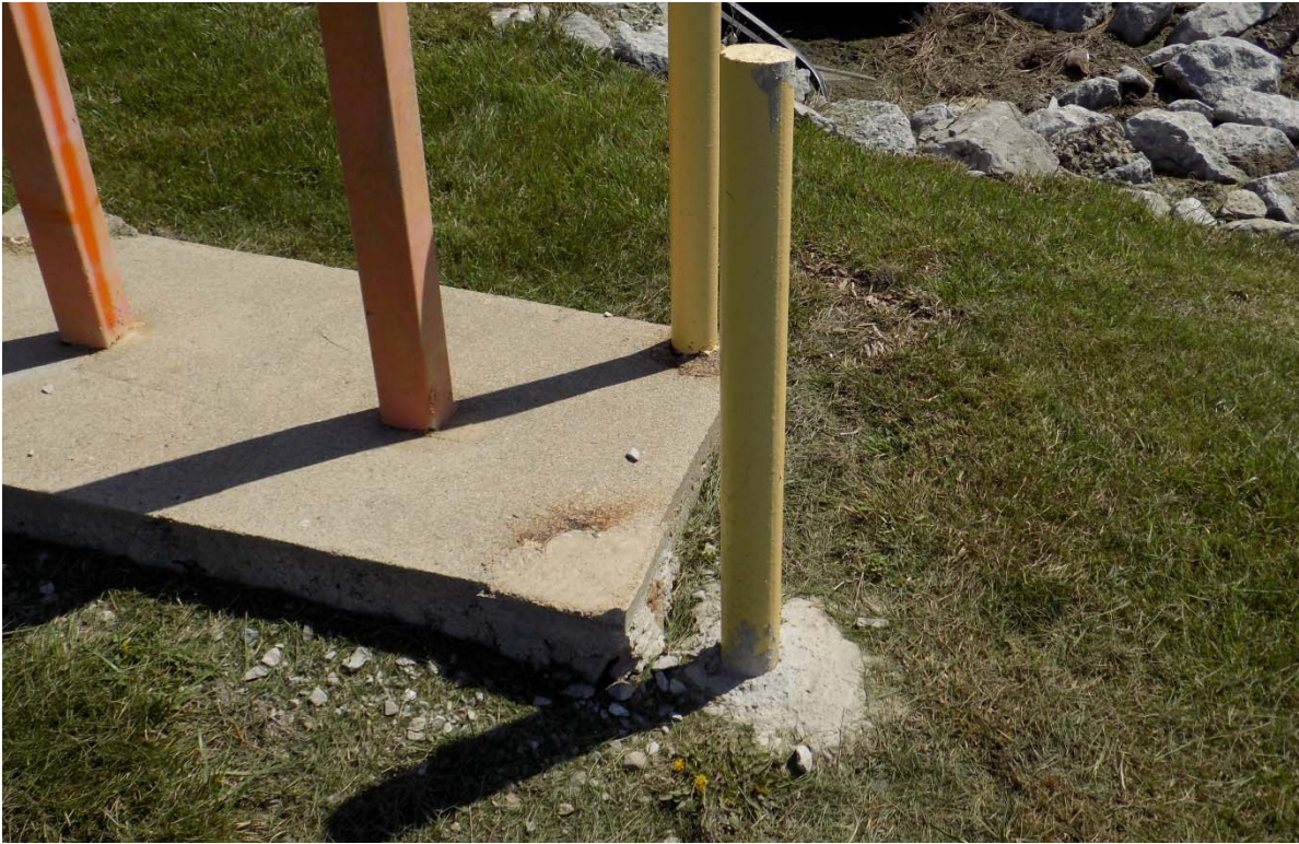
PL-11. Southwest Corner of OBS-8 Well Pad
