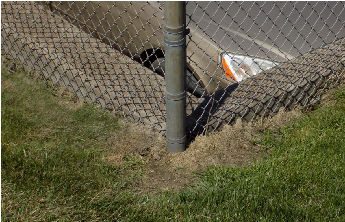
PL-8. Repaired Erosion Around Retaining Wall
