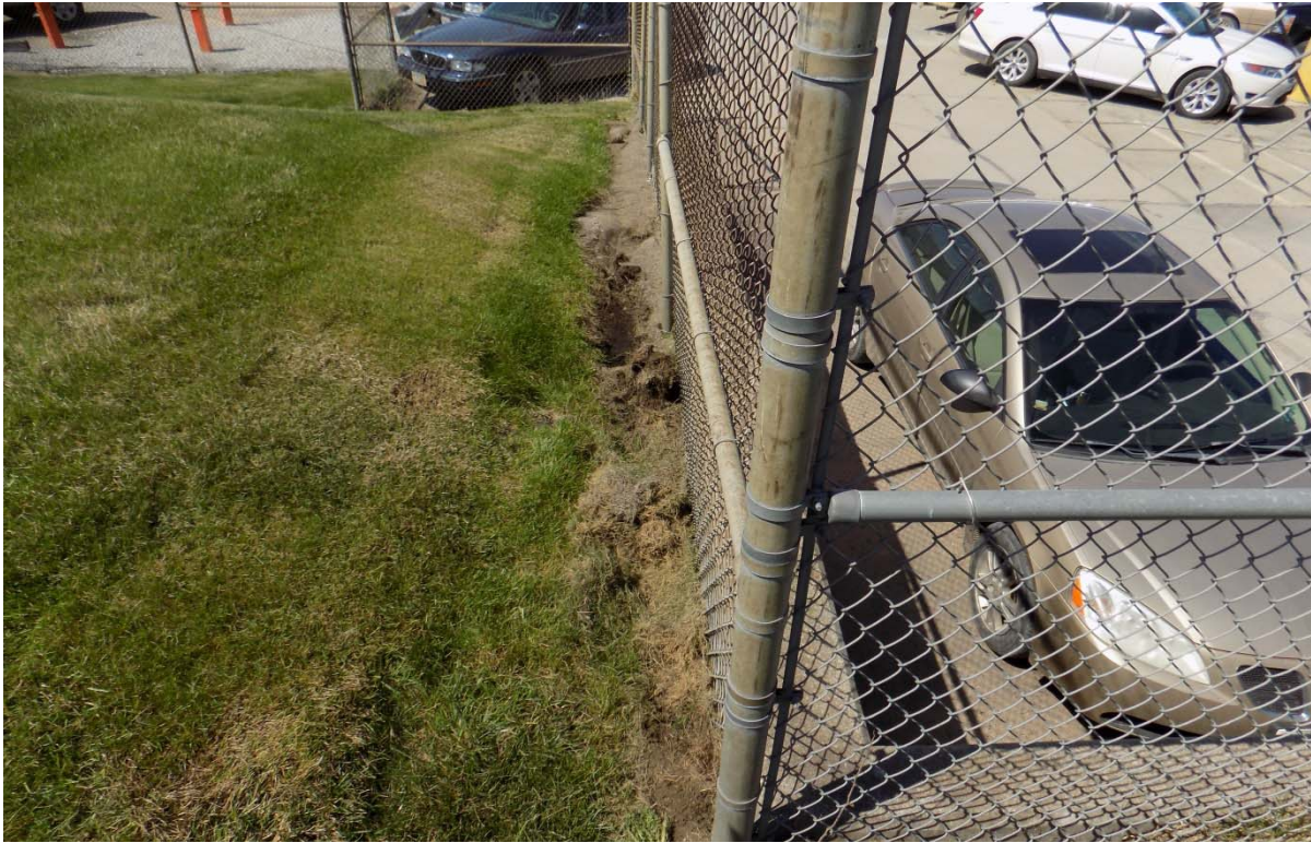
PL-9. Repaired Erosion Around Retaining Wall
