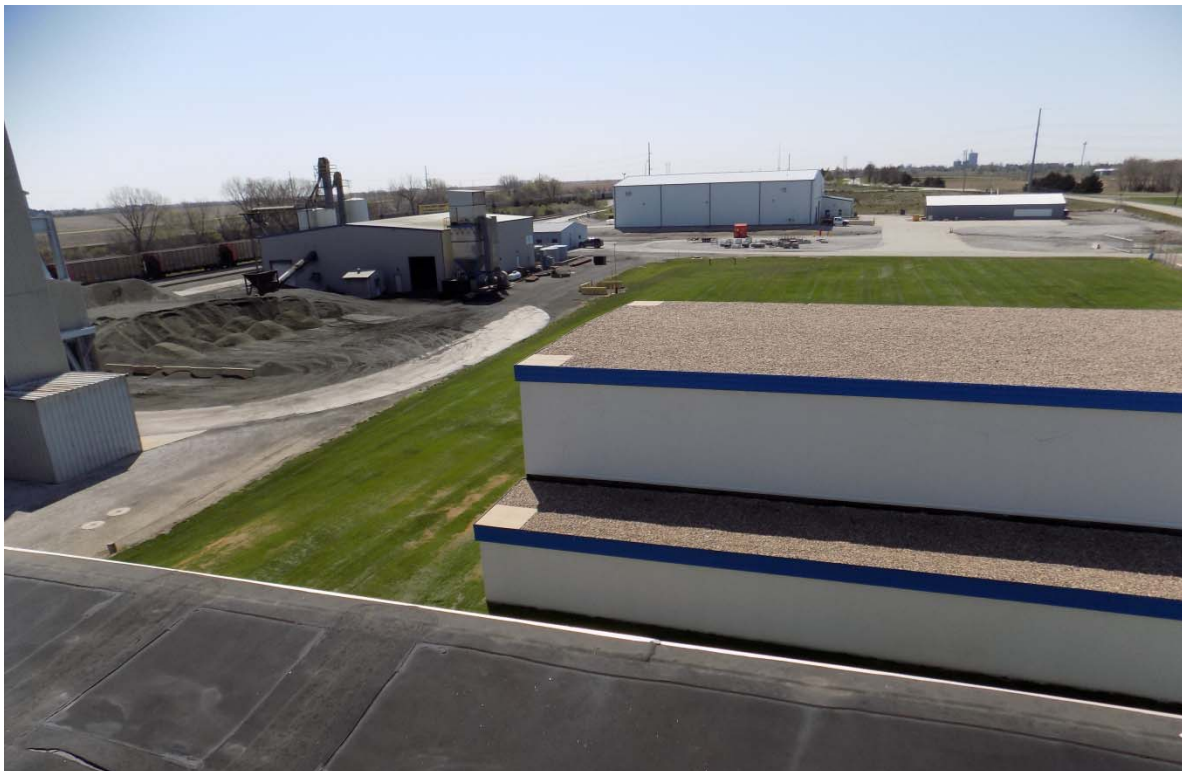
PL-2. East End of IHX Roof
