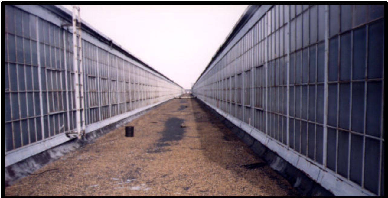
Figure 3-1. Overhead Beam Area Shown from Below and from Roof Above
