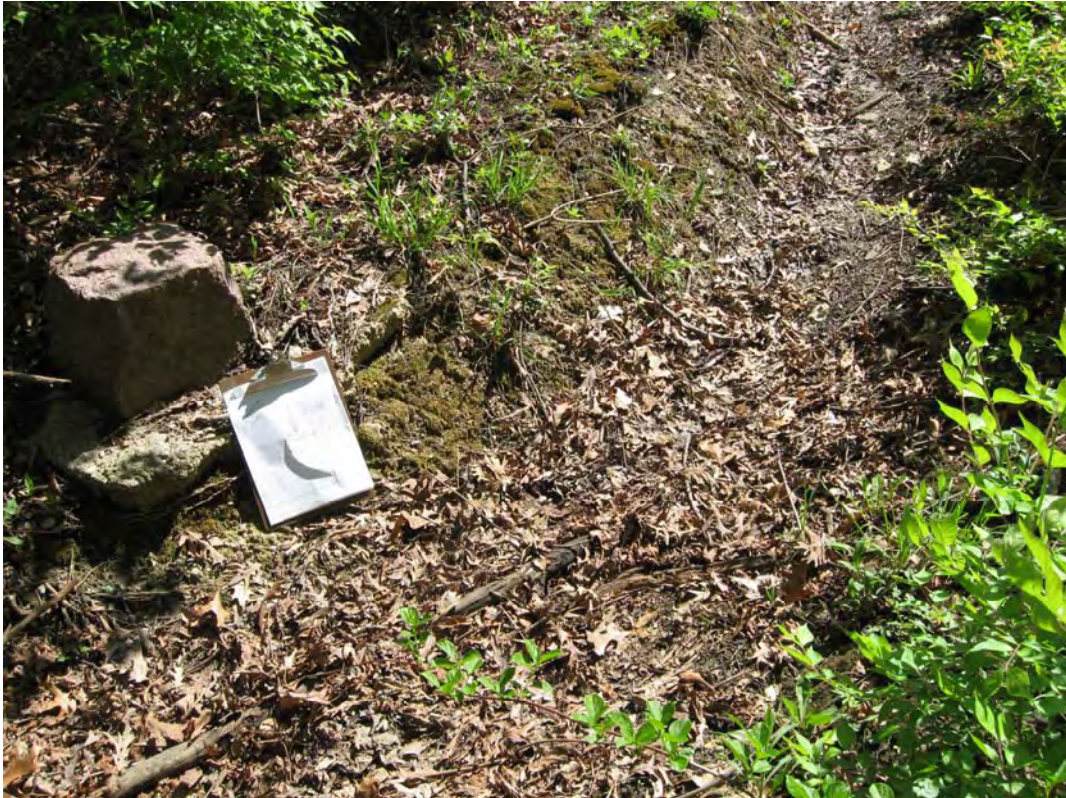
SAM 4/2010. PL-10. Erosion at Plot M west of the site marker.
