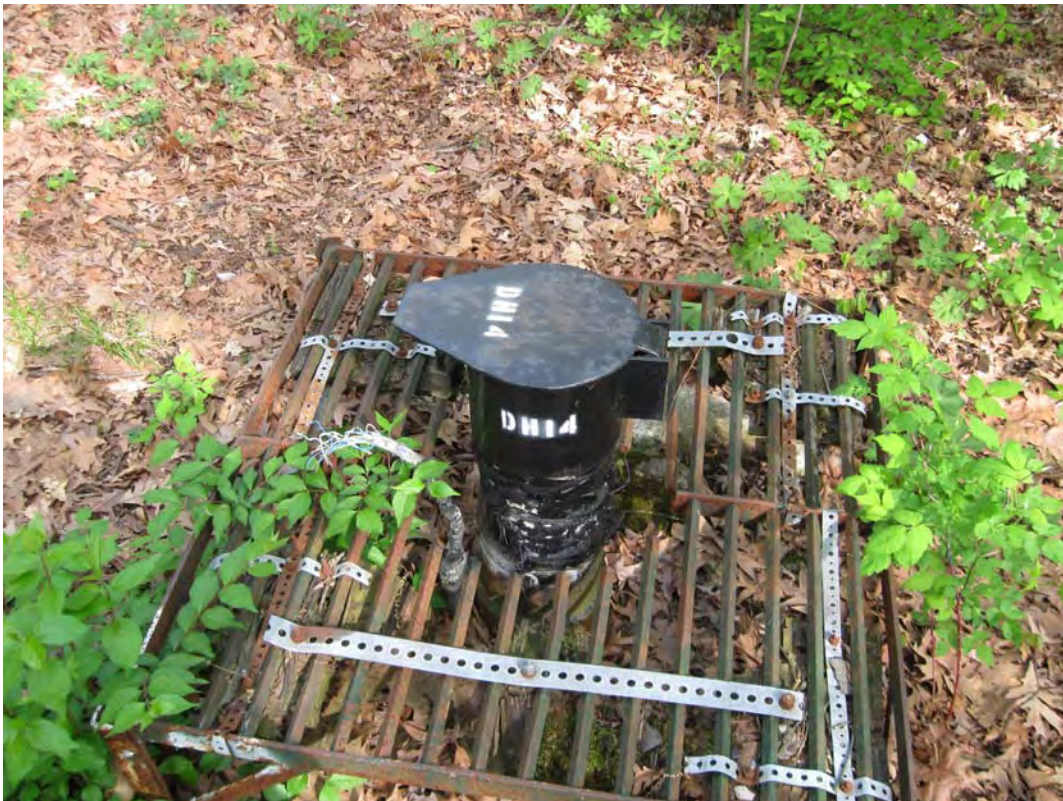
SAM 4/2010. PL-12. Grate around monitoring well DH-14.
