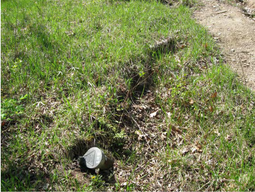
SAM 4/2010. PL-7. Monitoring well BH-9 impacted by erosion north of the Plot M site marker.
