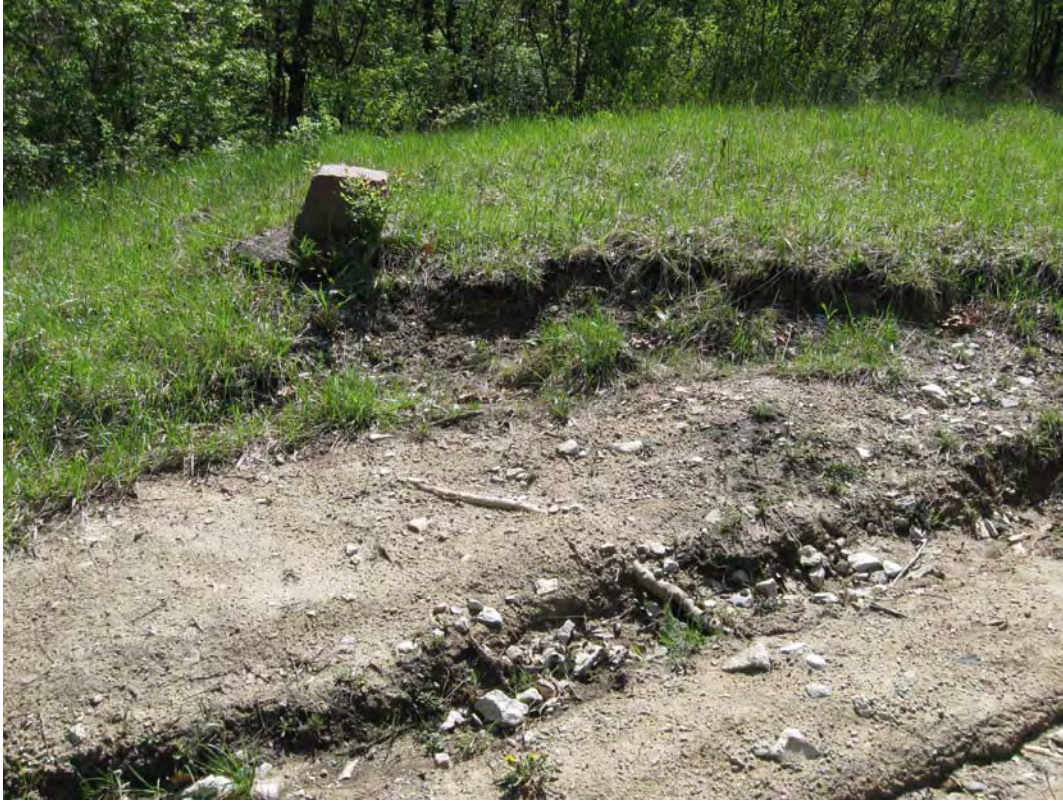
SAM 4/2010. PL-5. Erosion at Plot M, north of site marker.
