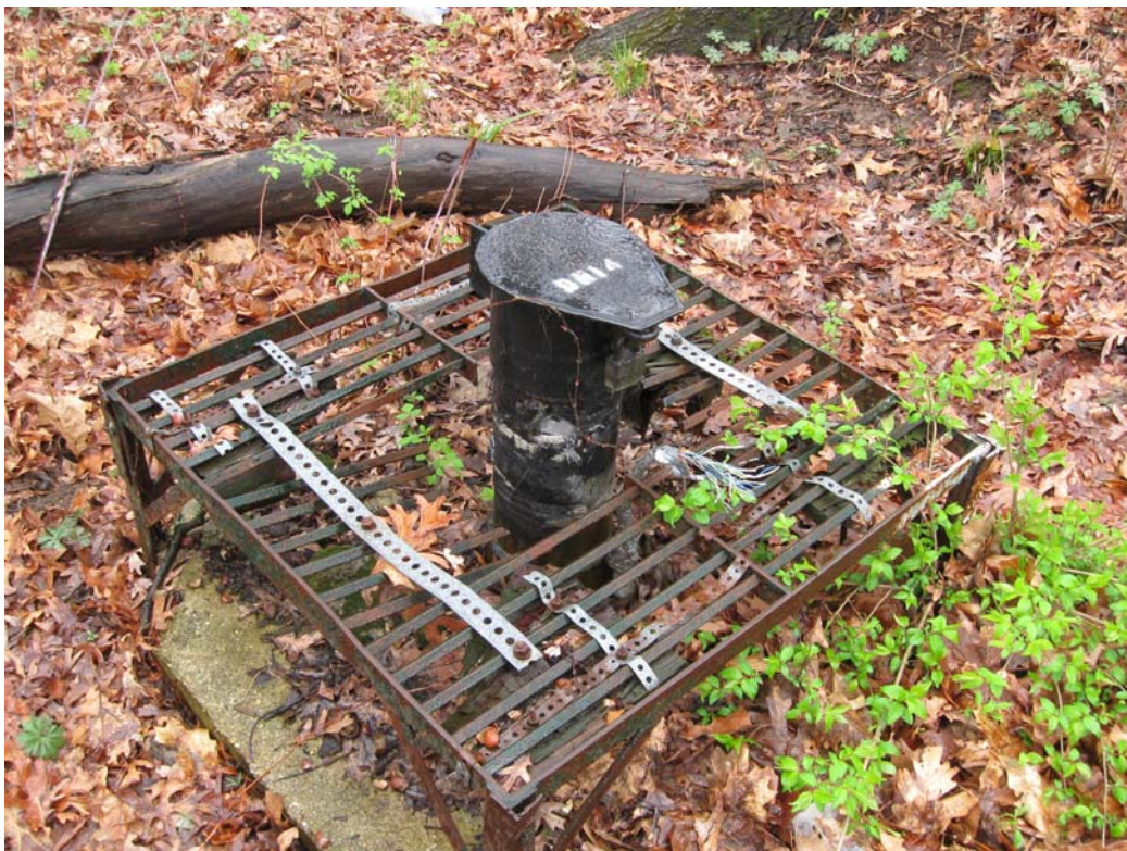
SAM 4/2011. PL-4. Wires and grate at monitoring well DH14.
