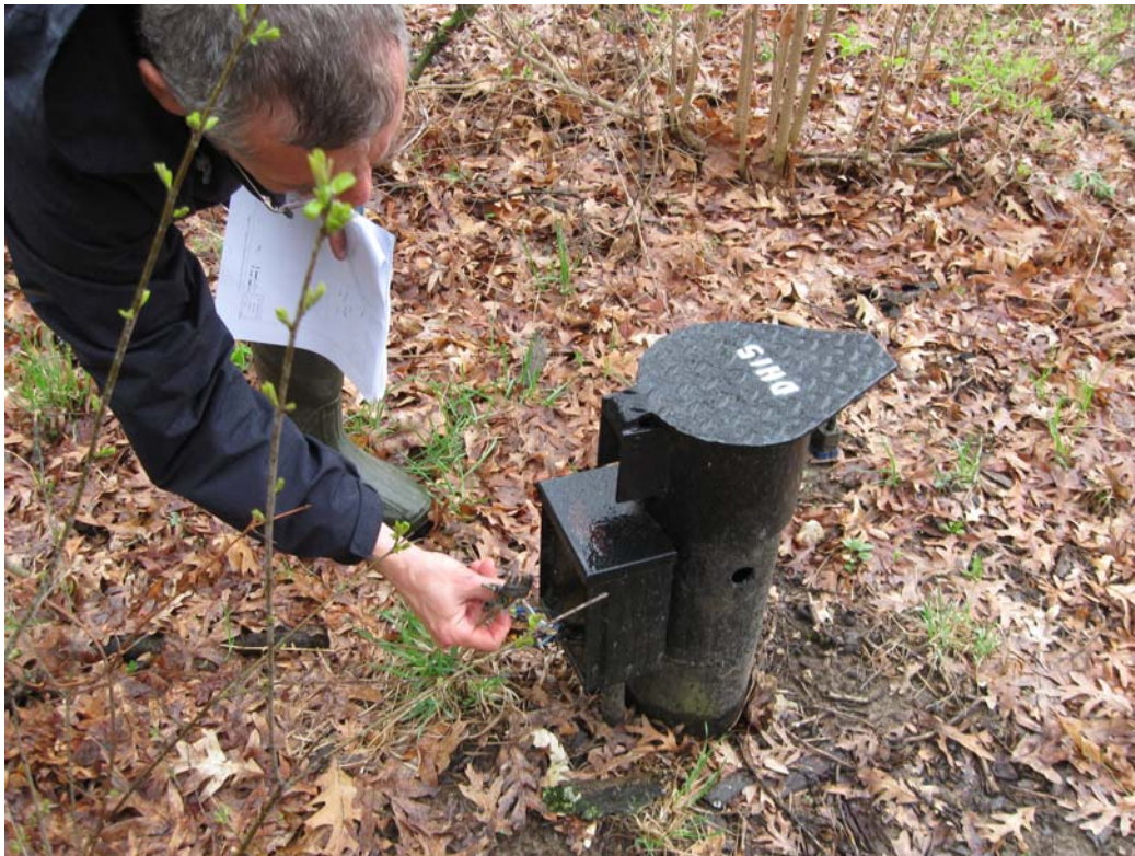
SAM 4/2011. PL-3. Wires protruding from monitoring well DH15.
