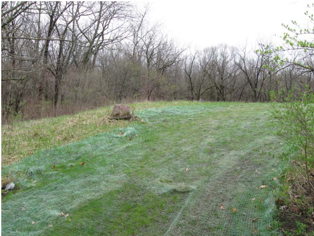
SAM 4/2011. PL-2. Erosion repair at Plot M.
