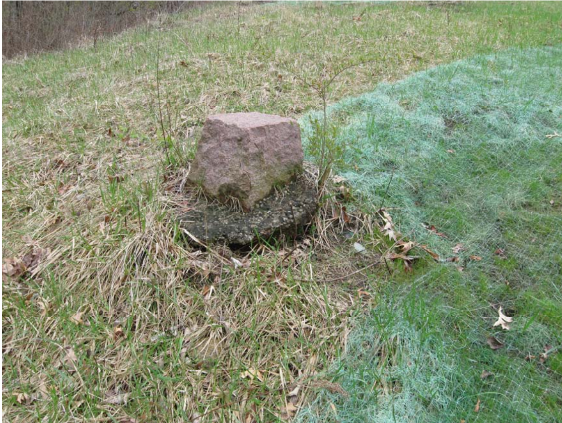
SAM 4/2011. PL-9. Erosion repair next to corner marker at Plot M.
