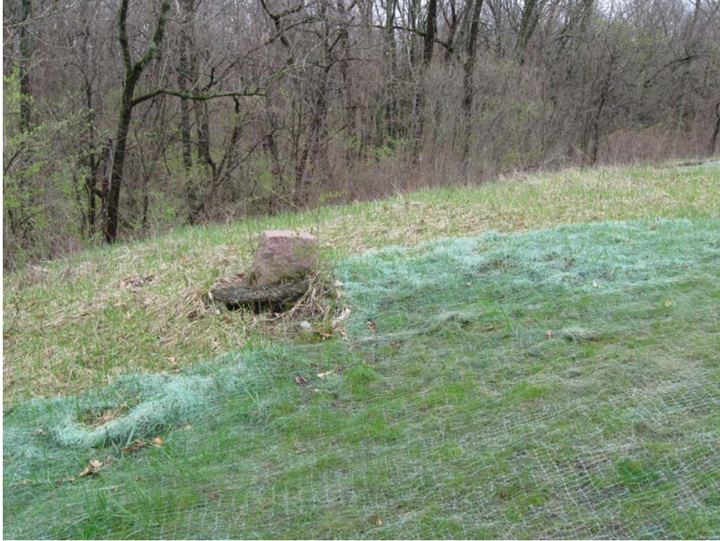
SAM 4/2011. PL-1. Erosion repair at Plot M.
