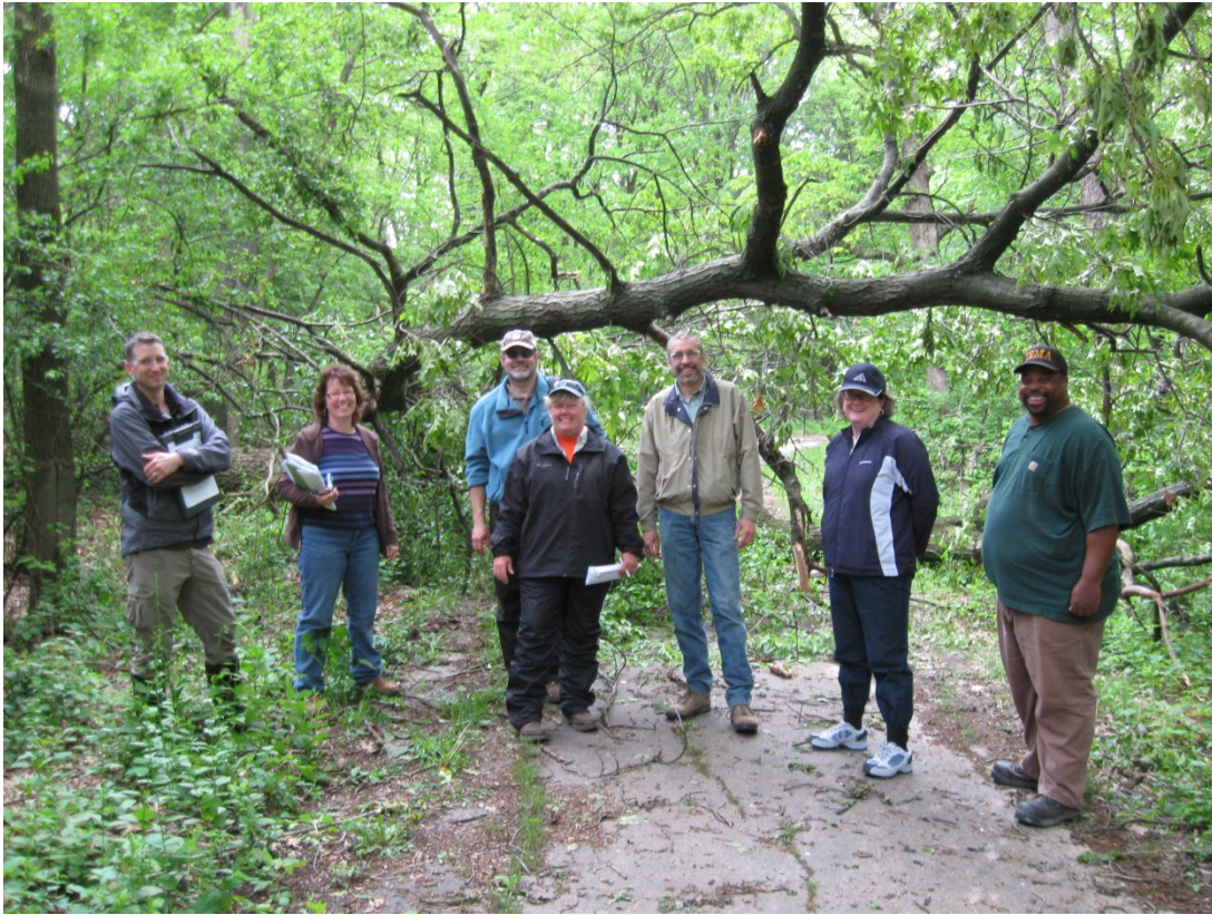
SAM 5/2012. PL-3. Fallen tree blocking access road to Site A.
