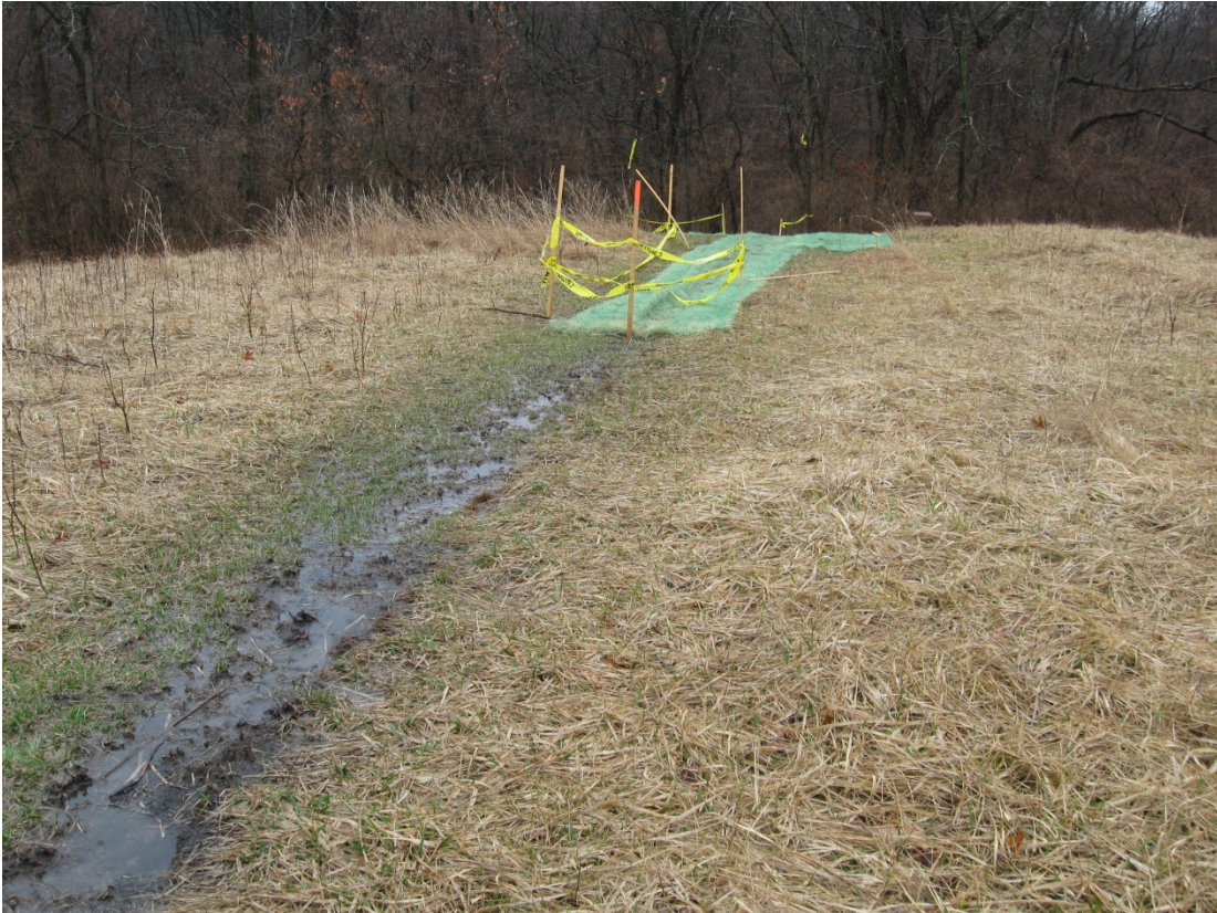
SAM 4/2013. PL-6. Recent rut repair work on top of Plot M.
