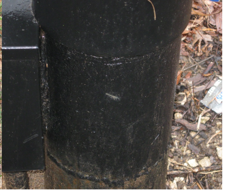
SAM 4/2013. PL-11. Repair on monitoring well BH-13.
