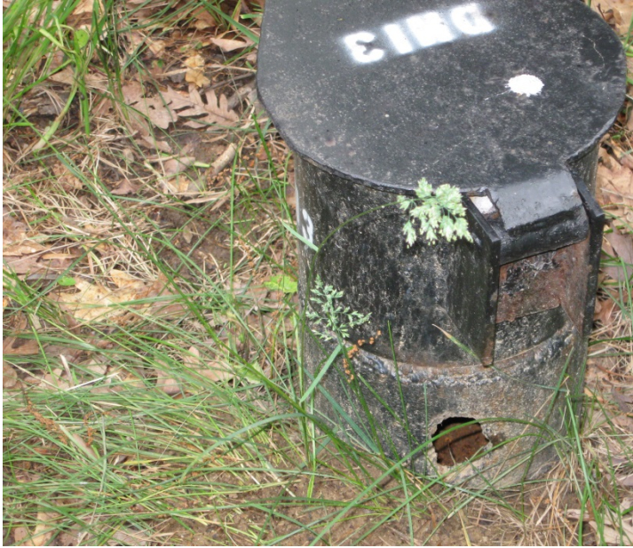
SAM 4/2013. PL-10. 2012 photo of monitoring well BH-13.
