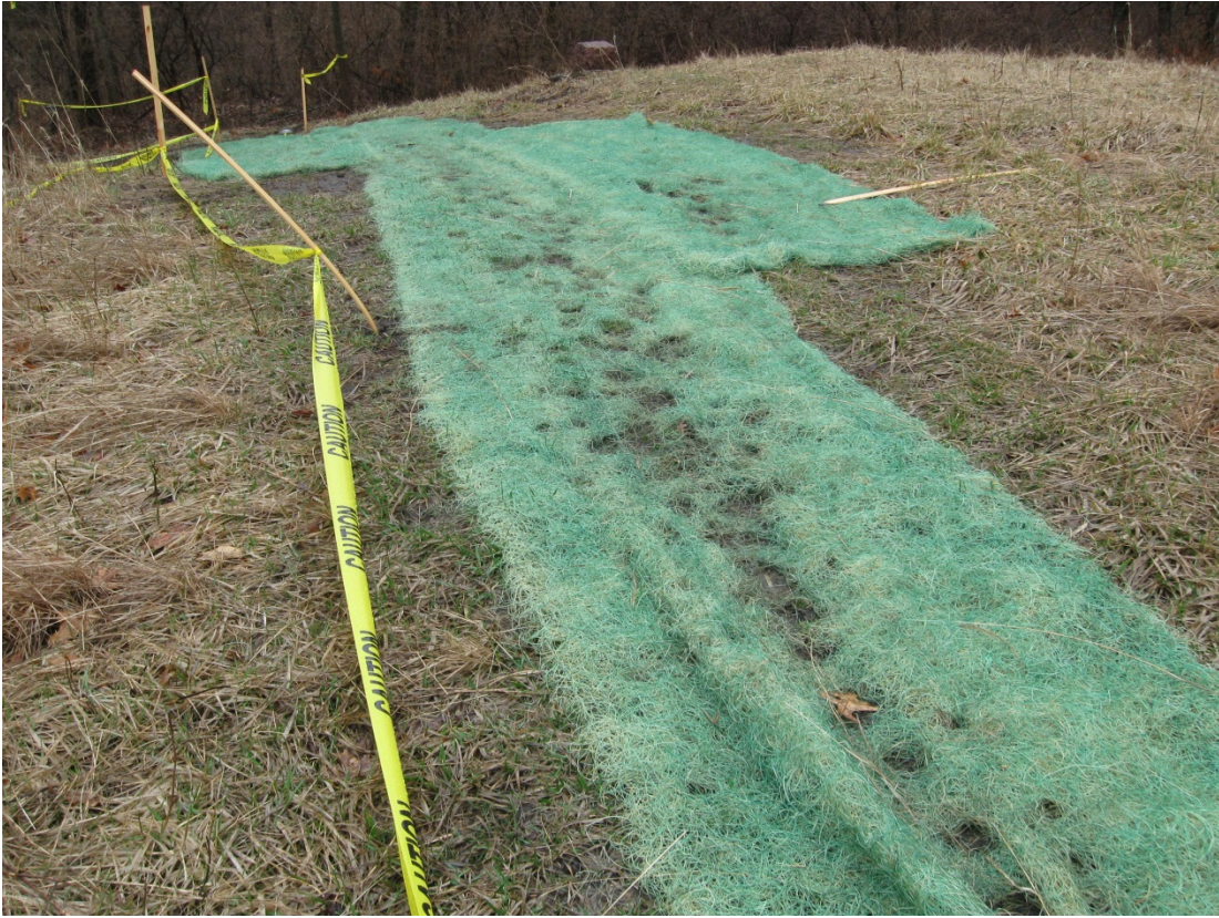
SAM 4/2013. PL-7. Recent rut repair work on top of Plot M.
