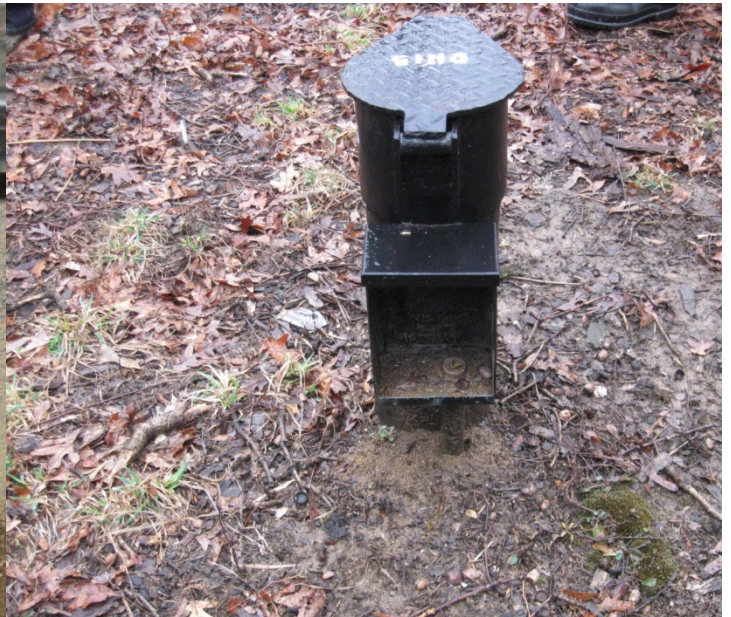
SAM 4/2013. PL-13. Repair on monitoring well BH-15.
