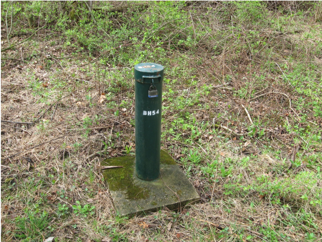
SAM 4/2014. PL-3. Monitoring well BH-54.
