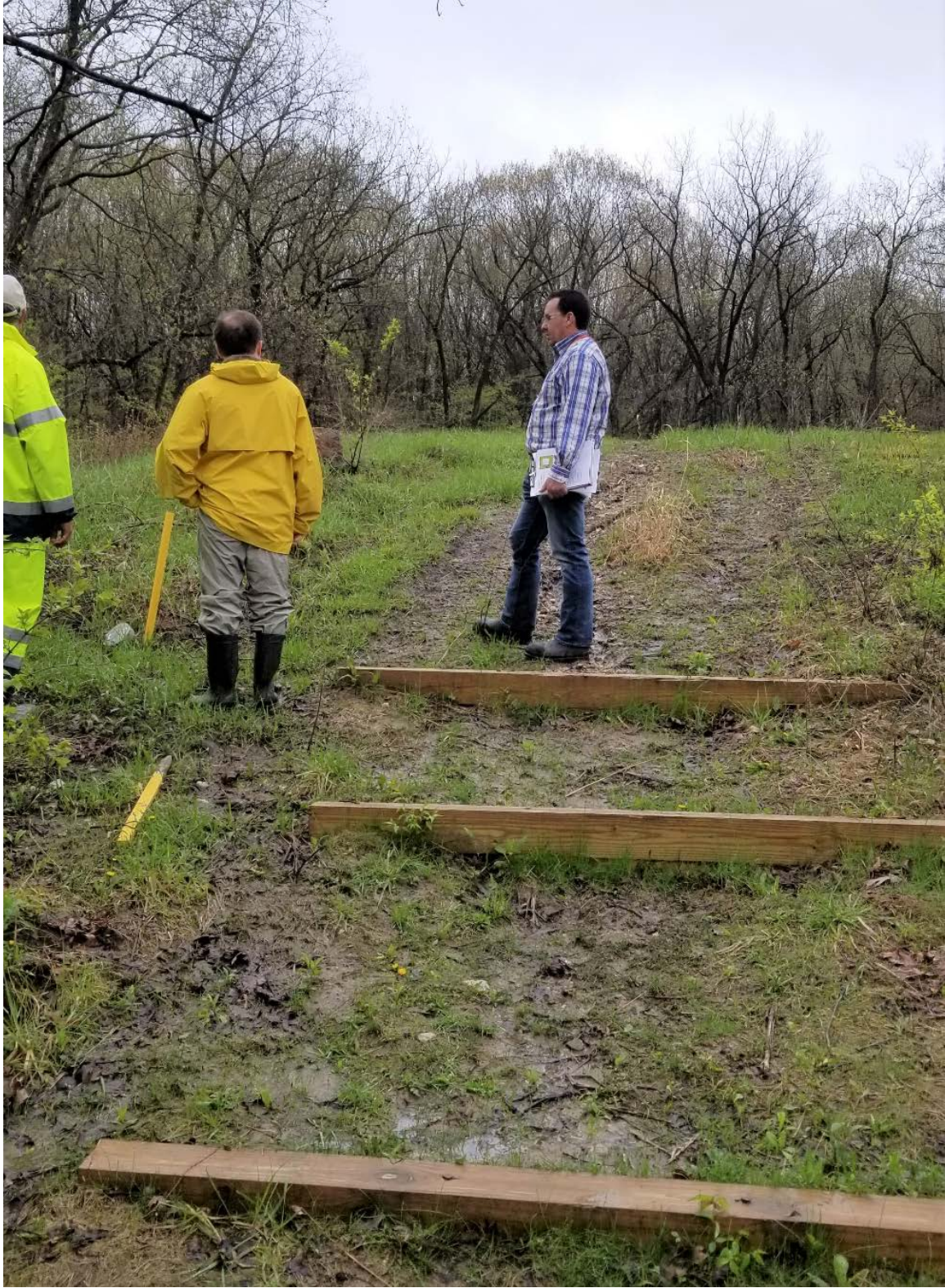
Figure 1.1 View of timber steps installed along northeast path at Plot M.
