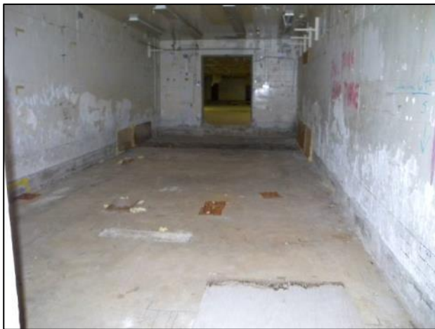
Figure C-34. T Building Room 58 View C
