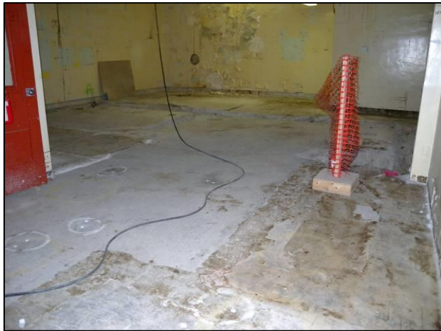
Figure C-20. T Building Room 63 View A
