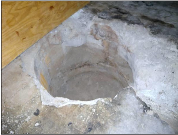
Figure C-6. T Building Room 16 View E
