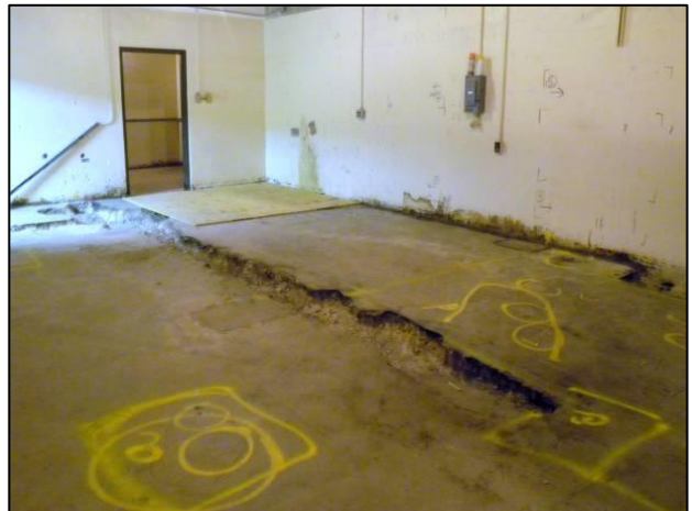
Figure C-11. T Building Room 16 View J
