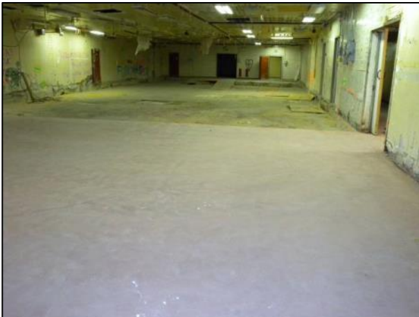
Figure C-38. T Building Rooms 39-44 and 48-50 View A
