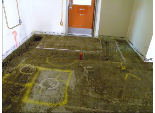
Figure C-17. T Building Room 61 View F
