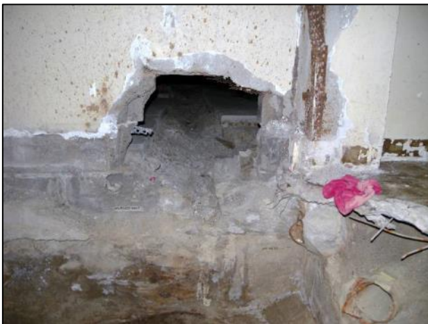
Figure C-28. T Building Room 63 View I
