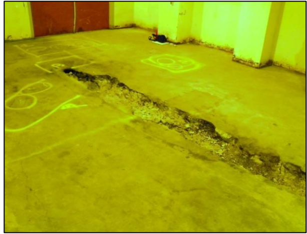
Figure C-7. T Building Room 16 View F
