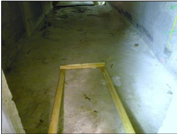
Figure C-32. T Building Room 57 View A
