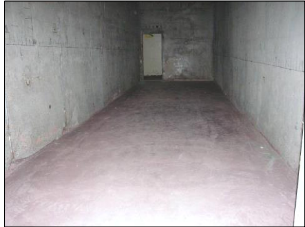
Figure C-37. T Building Room 59 View F
