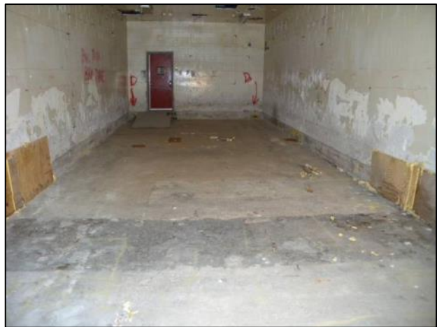
Figure C-35. T Building Room 58 View D
