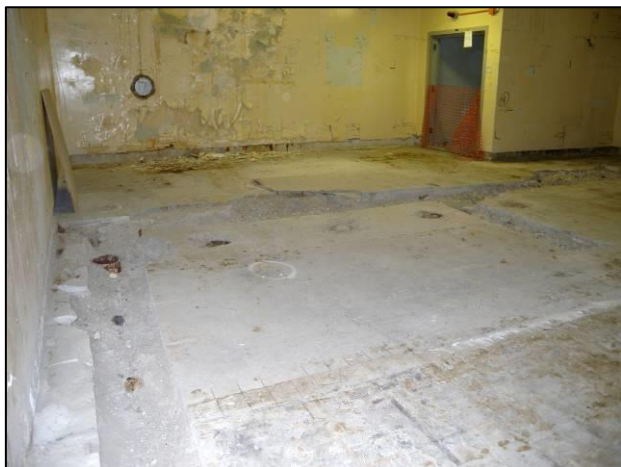
Figure C-22. T Building Room 63 View C
