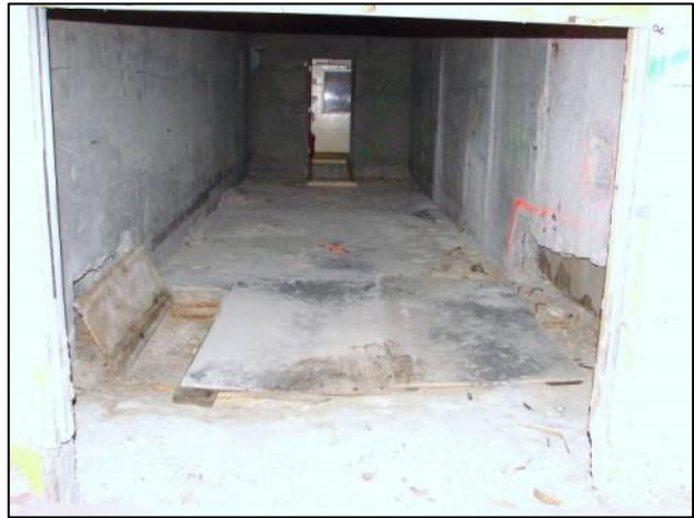
Figure C-33. T Building Room 57 View B
