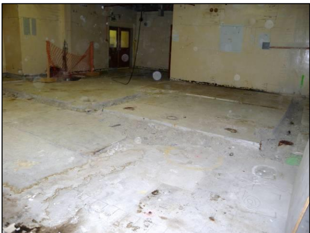
Figure C-23. T Building Room 63 View D
