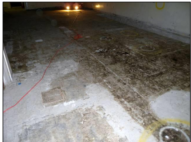
Figure C-15. T Building Room 61 View D
