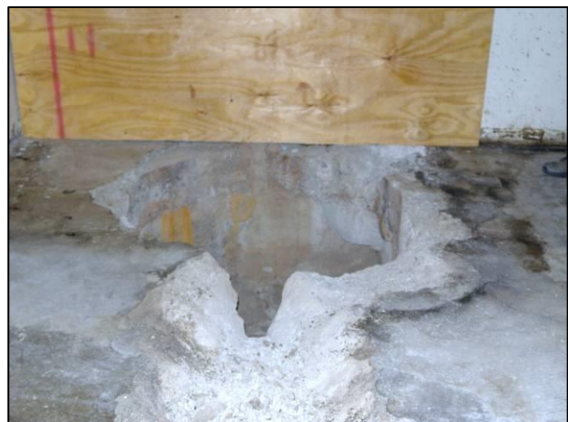
Figure C-5. T Building Room 16 View D
