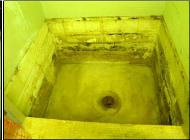
Figure C-31. T Building Room 62 View L
