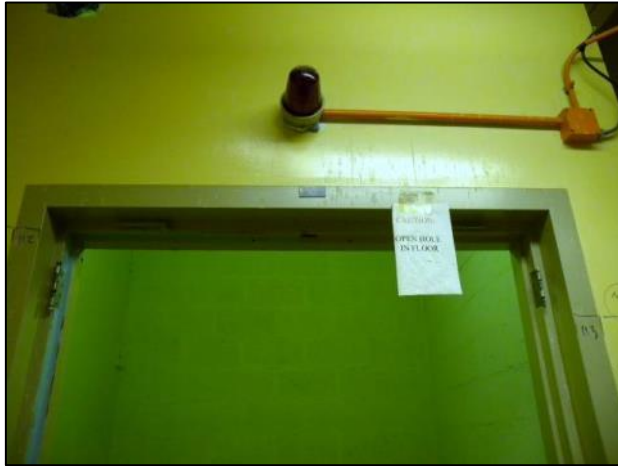
Figure C-30. T Building Room 62 View K
