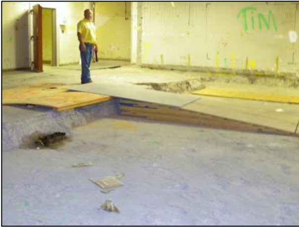
Figure C-42. T Building Rooms 39-44 and 48-50 View E
