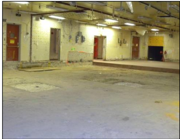
Figure C-45. T Building Rooms 39-44 and 48-50 View H
