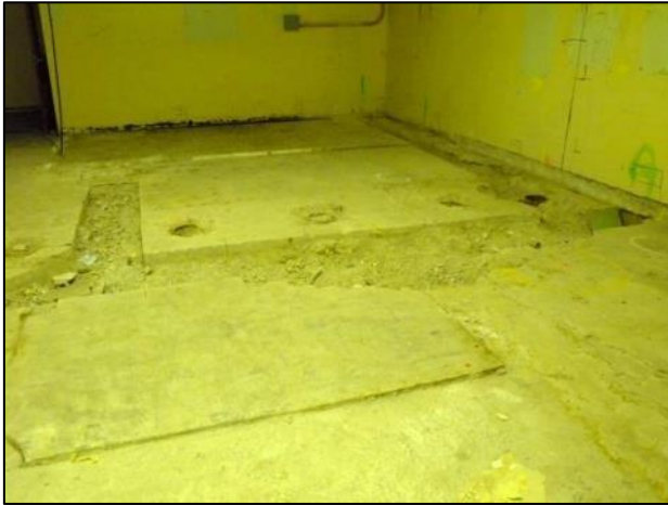
Figure C-24. T Building Room 63 View E
