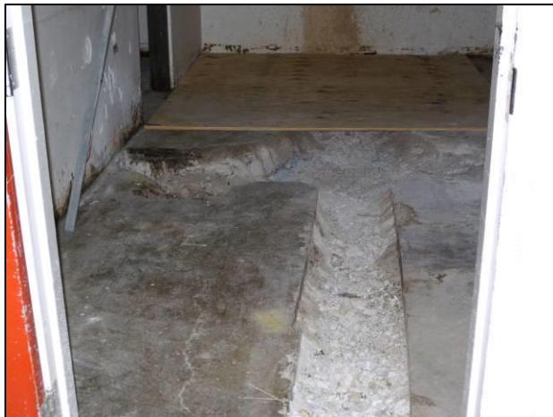
Figure C-2. T Building Room 16 View A
