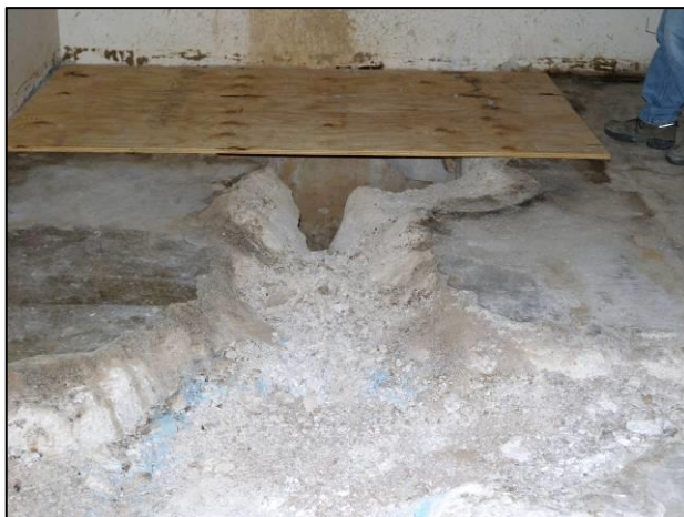
Figure C-4. T Building Room 16 View C
