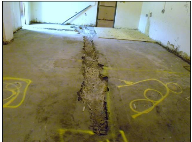
Figure C-9. T Building Room 16 View H
