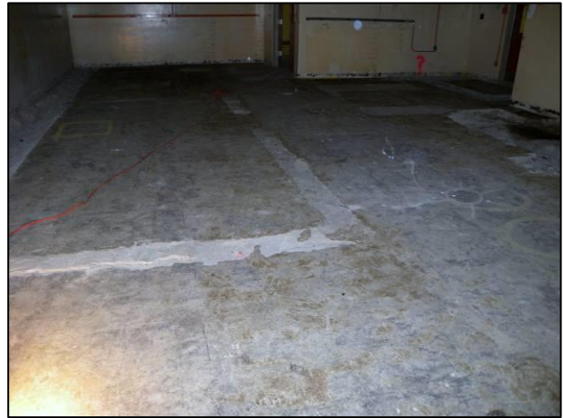
Figure C-13. T Building Room 61 View B
