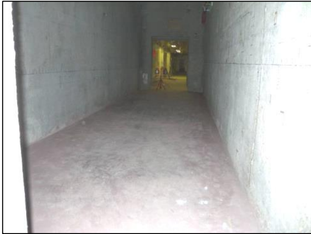
Figure C-36. T Building Room 59 View E
