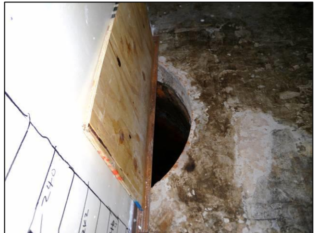
Figure C-19. T Building Room 61 View H
