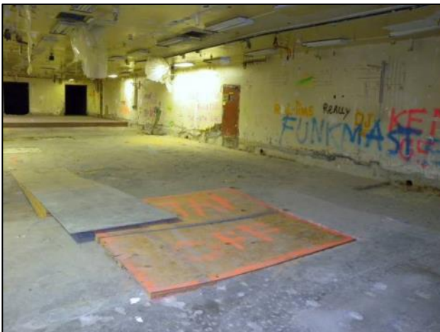
Figure C-46. T Building Rooms 39-44 and 48-50 View I
