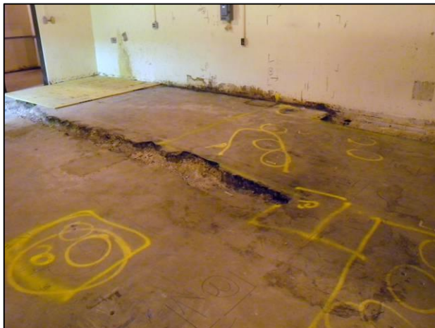
Figure C-10. T Building Room 16 View I
