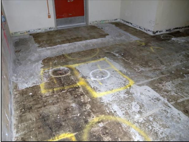
Figure C-16. T Building Room 61 View E
