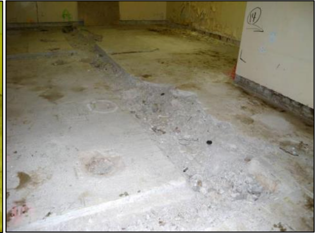
Figure C-25. T Building Room 63 View F
