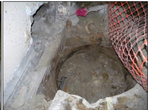
Figure C-27. T Building Room 63 View H
