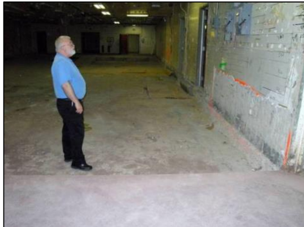
Figure C-39. T Building Rooms 39-44 and 48-50 View B
