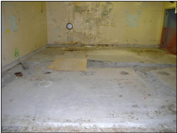
Figure C-21. T Building Room 63 View B
