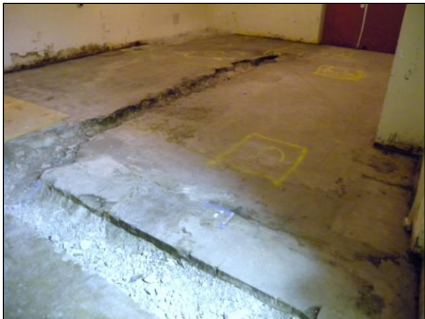
Figure C-3. T Building Room 16 View B
