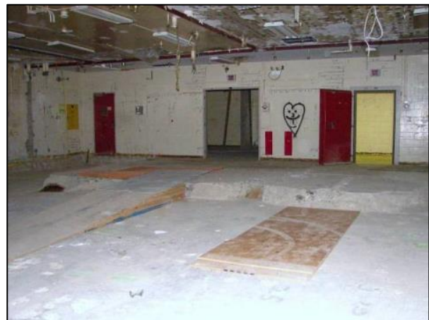
Figure C-41. T Building Rooms 39-44 and 48-50 View D
