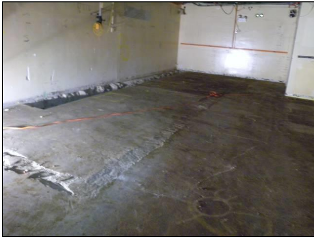
Figure C-12. T Building Room 61 View A
