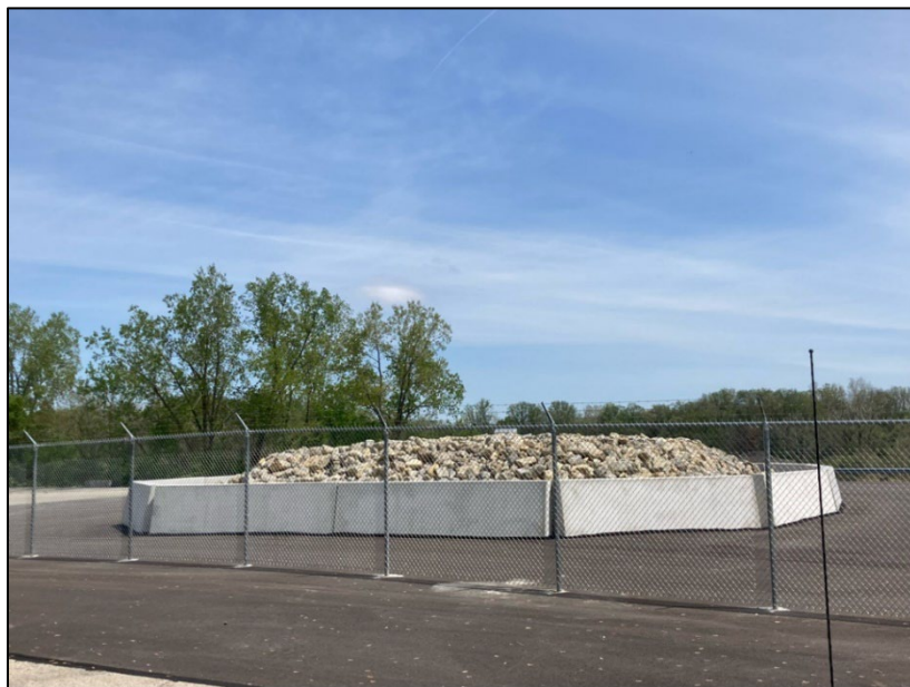
Figure 1. Onsite Low-Level Radioactive Waste Entombment
