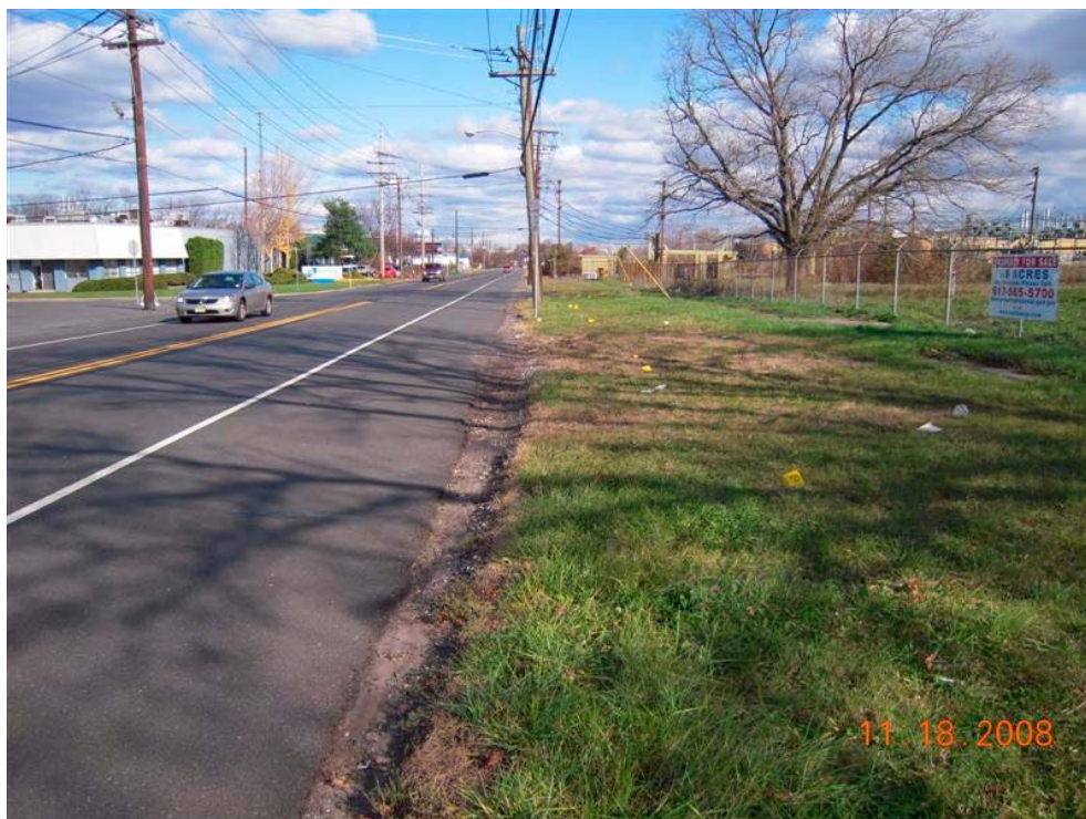
Jersey Avenue, looking north, overhead phone and electric lines, underground gas line marked with yellow flags
