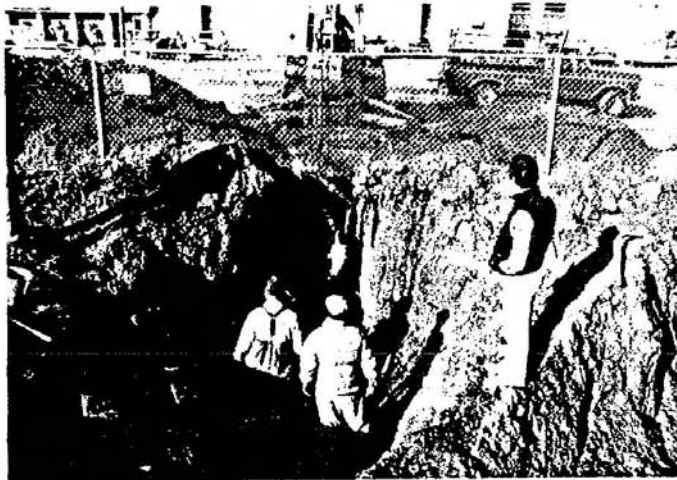
Figure A-22. Preparation of Seal Inlet to City Sewer Main
