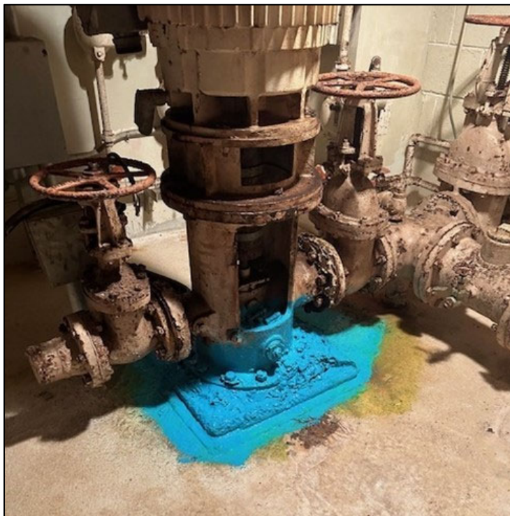
Figure 7. Basement Contamination Area Pump with Fixative Applied, Front View
