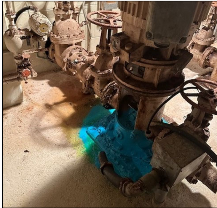
Figure 8. Basement Contamination Area Pump with Fixative Applied, Rear View
