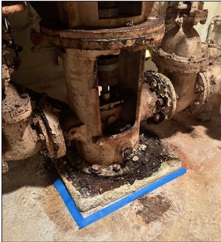
Figure 6. Basement Contamination Area—Offending Pump
