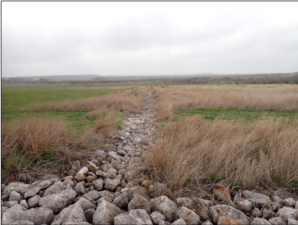
PL-7. Rock Drain on South Corner of Disposal Cell
