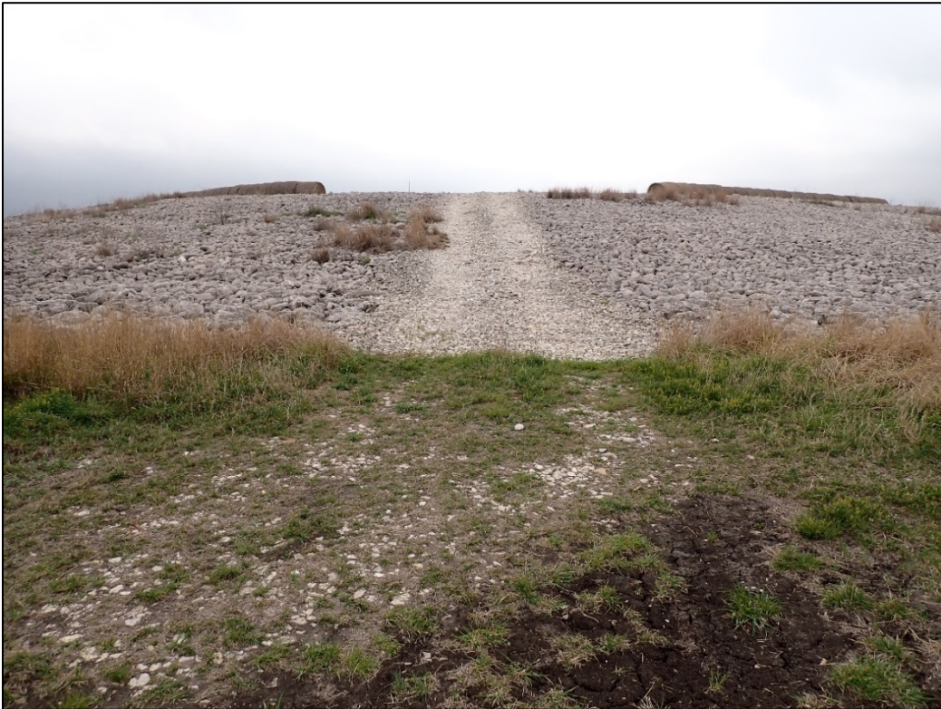
PL-6. Equipment Access Ramp
