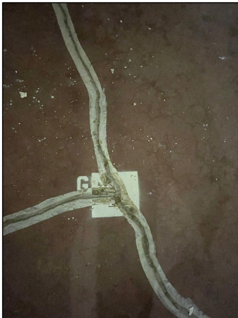
Figure 18. Closeup of Sealed Crack in the Red Concrete (1C-10)
