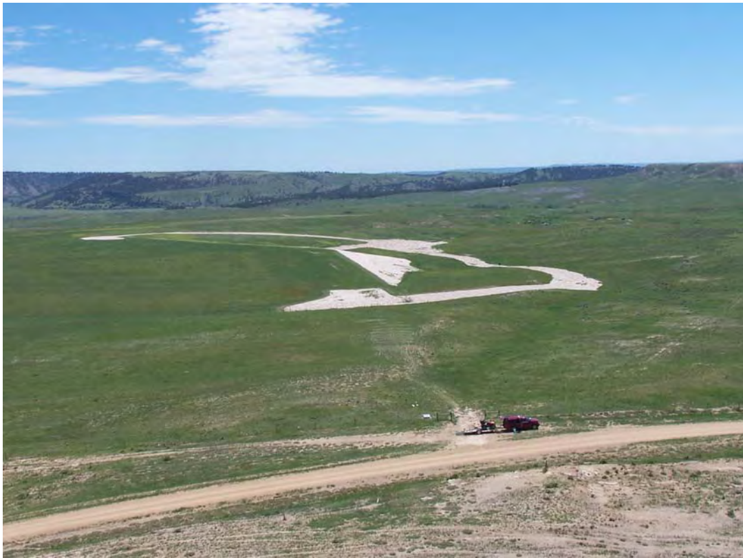
EDG 6/2008. PL-7. Southeast portion of the disposal cell showing the tailings embankment and diversion channels.
