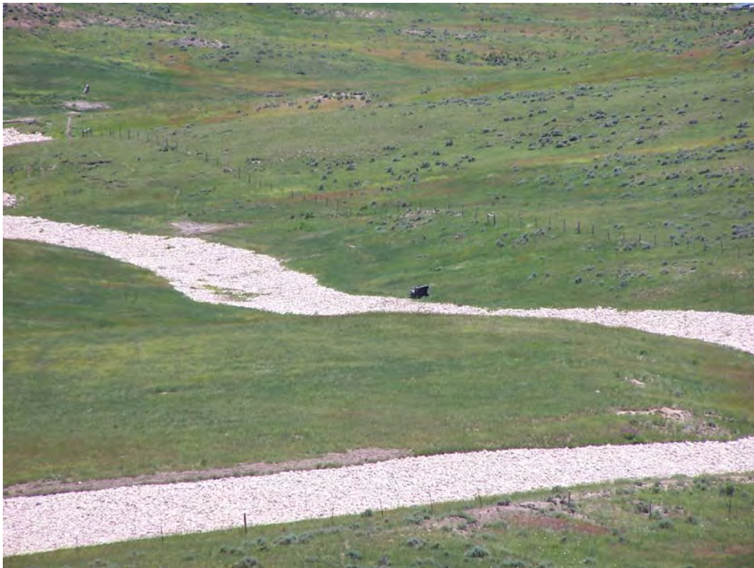
EDG 6/2008. PL-9. West diversion channel.
