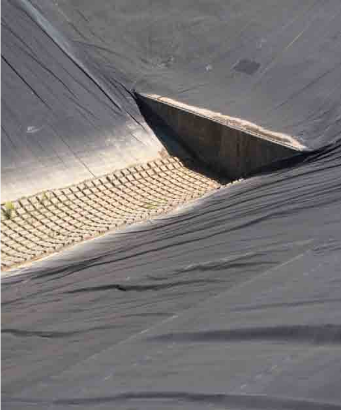
Headwall at NE corner at end of North channel.
