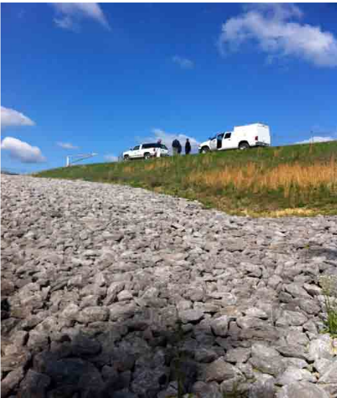
Top of EDB emergency spillway.
