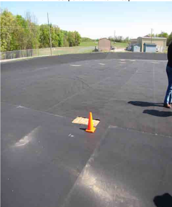
Independent liner inspection liner sample collection in northwest portion of interim cap.
