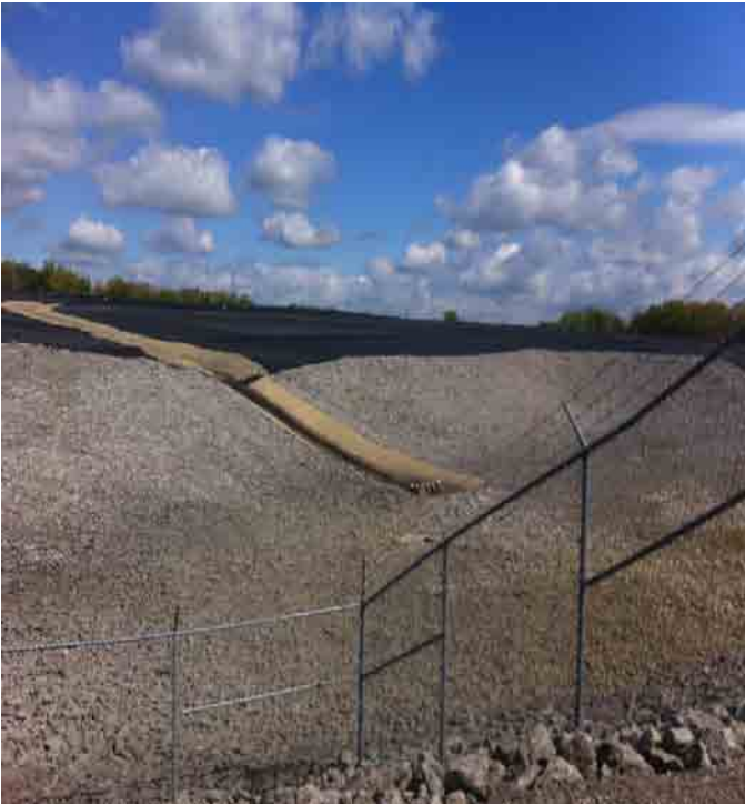
EDB and outfall of Y channel
