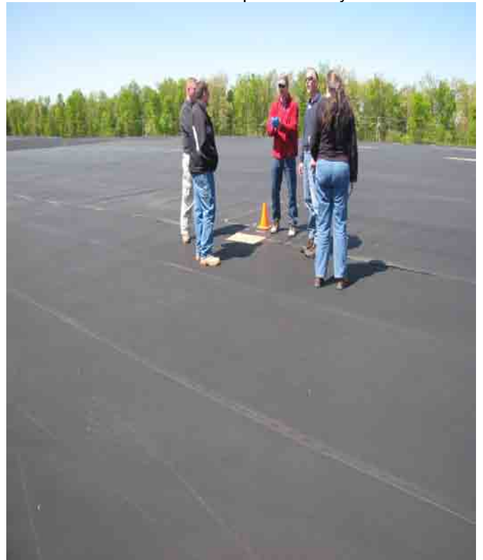
Independent liner inspection; liner sample collection.
