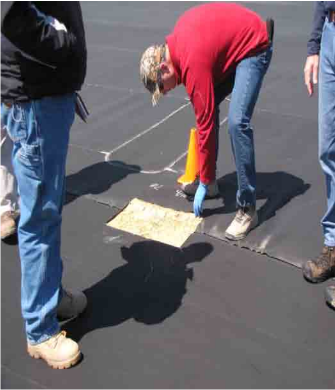
Independent liner inspection; liner sample collection.
