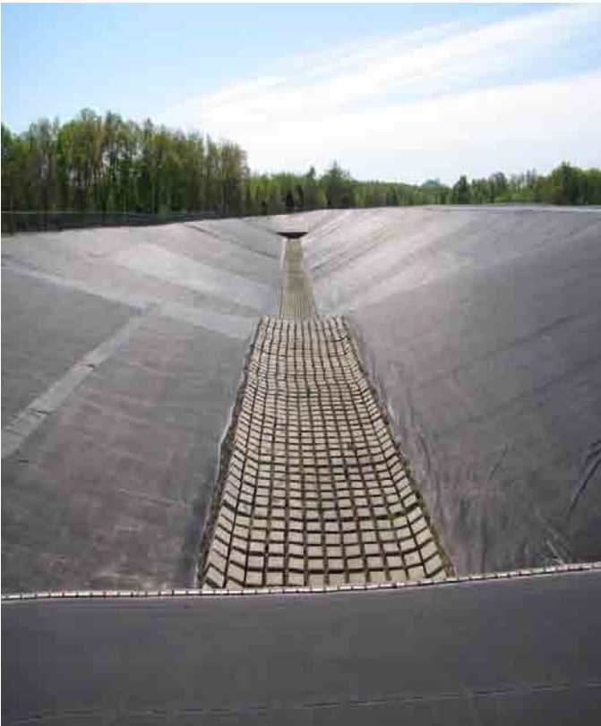
North channel looking east.
