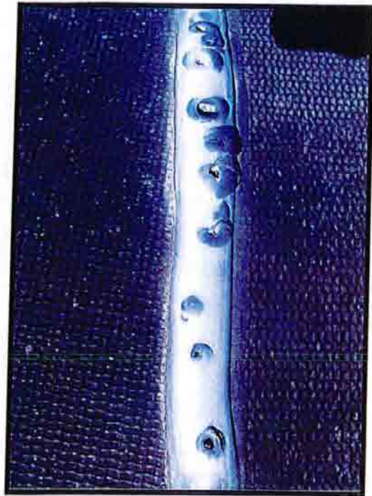
Typical "Bubbling" Failure of Extrusion Weld
