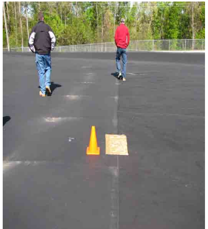
Independent liner inspection liner sample collection in northwest portion of interim cap.
