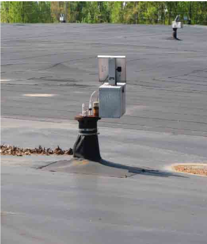
Sump protrusion through interim cap.
