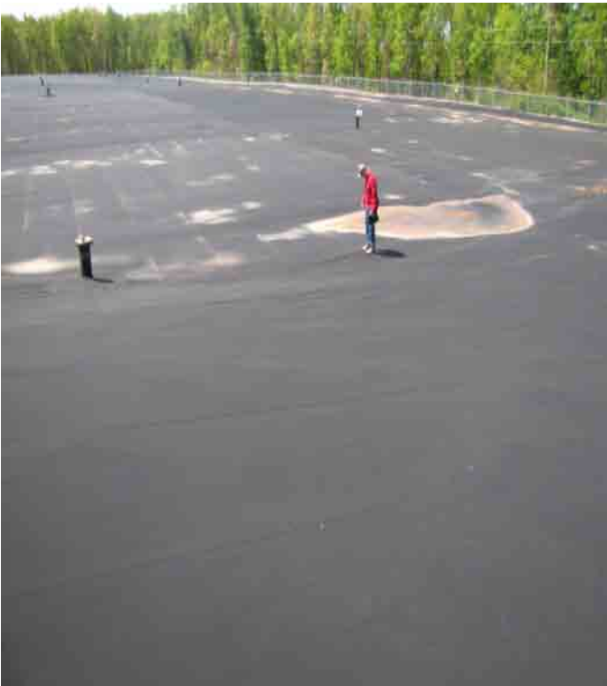
View of interim cap from EMC bunker looking southwest.
