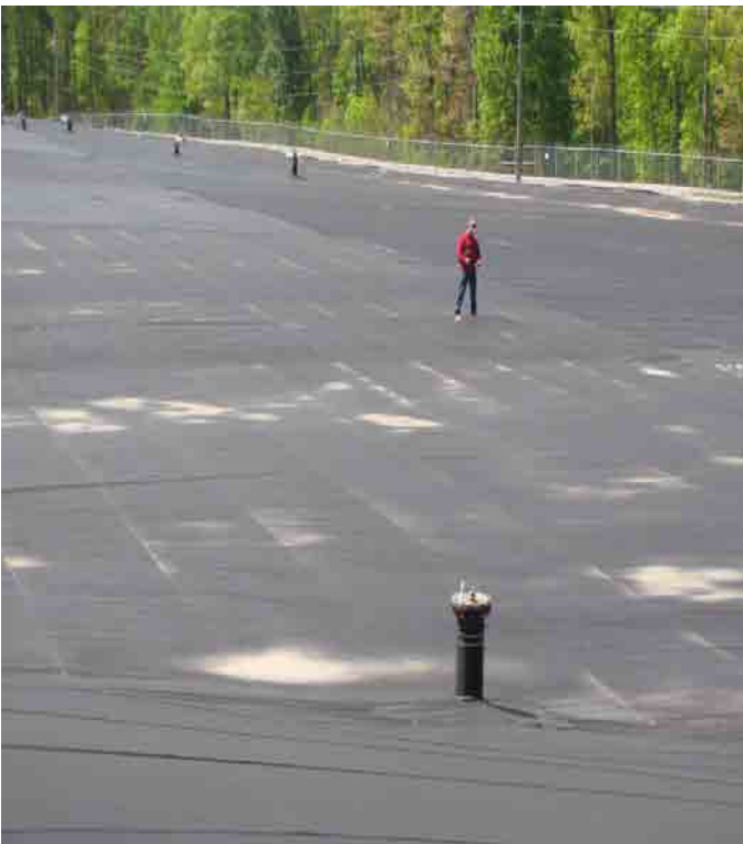
View of interim cap from EMC bunker looking southwest.
