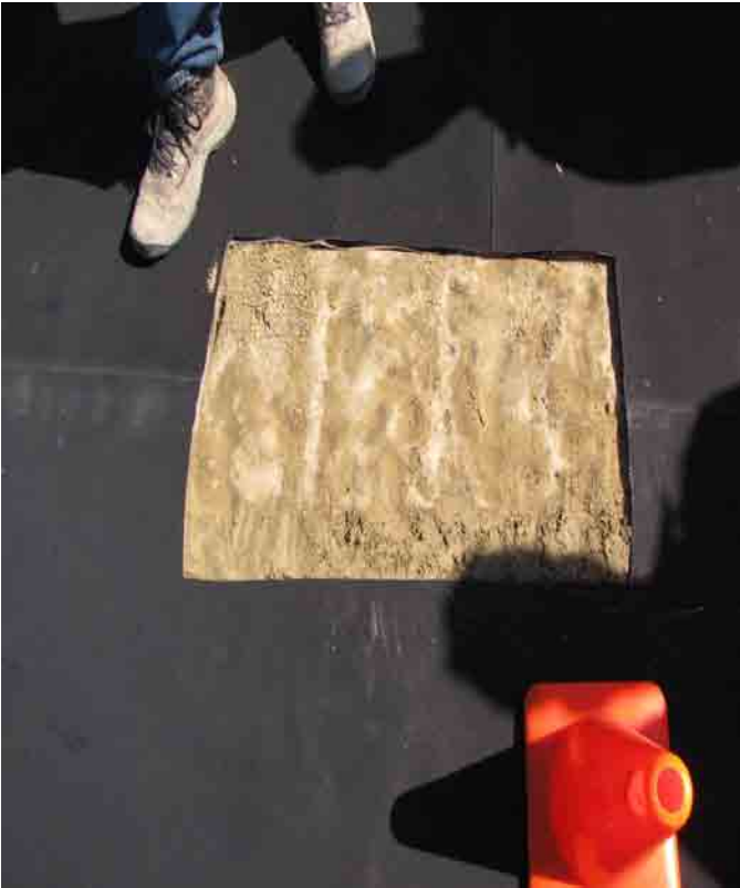
Close-up picture of liner subsurface after collecting liner sample.
