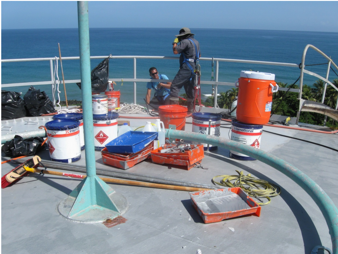
BON 8/2013. PL-3. Top of dome, paint supplies.
