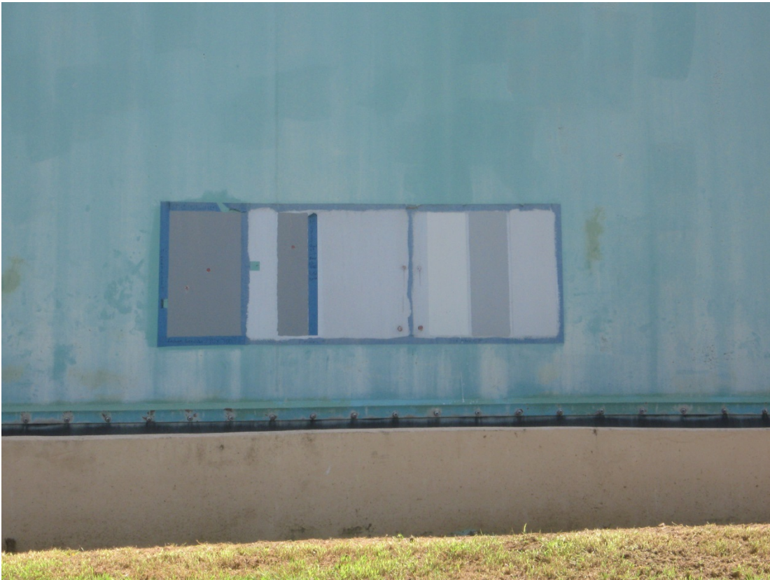
BON 8/2013. PL-1. Test paint – outside surface of containment dome.
