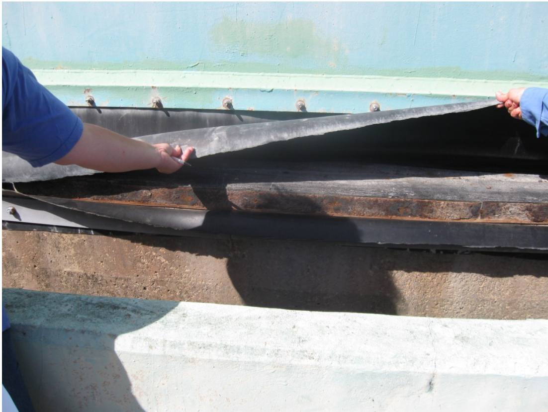
BON 8/2013. PL-5. Repairs to seal around base of dome.
