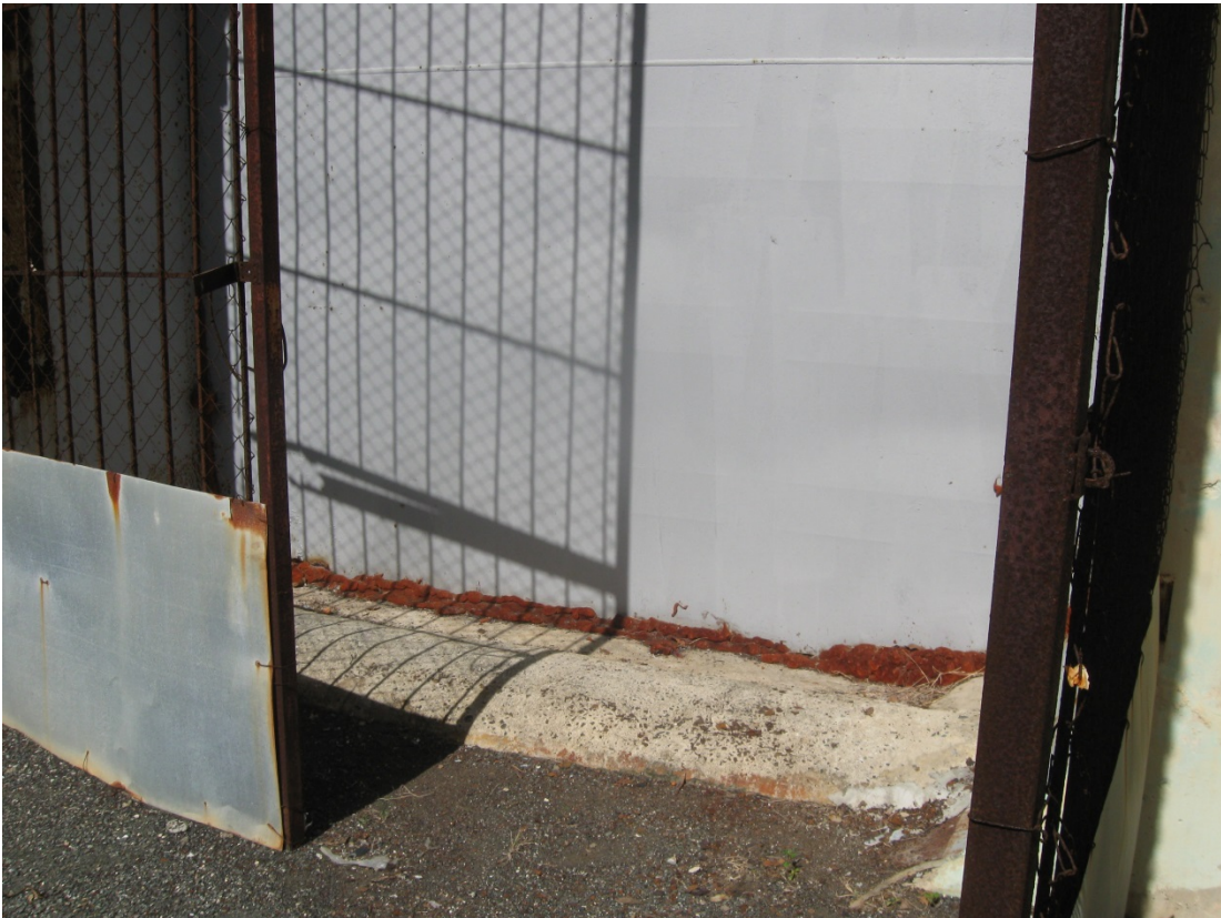
BON 8/2013. PL-10. Freight door, east side of containment building.
