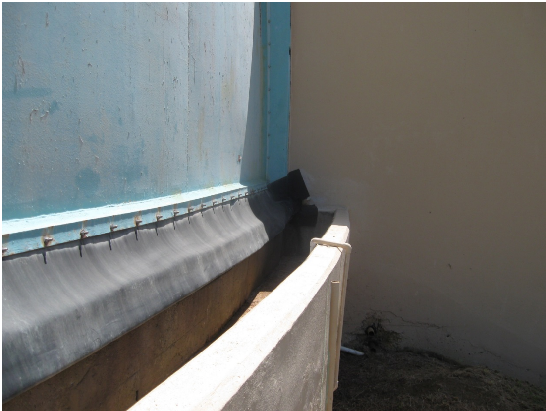
BON 8/2013. PL-6. Flashing repair along base of dome.
