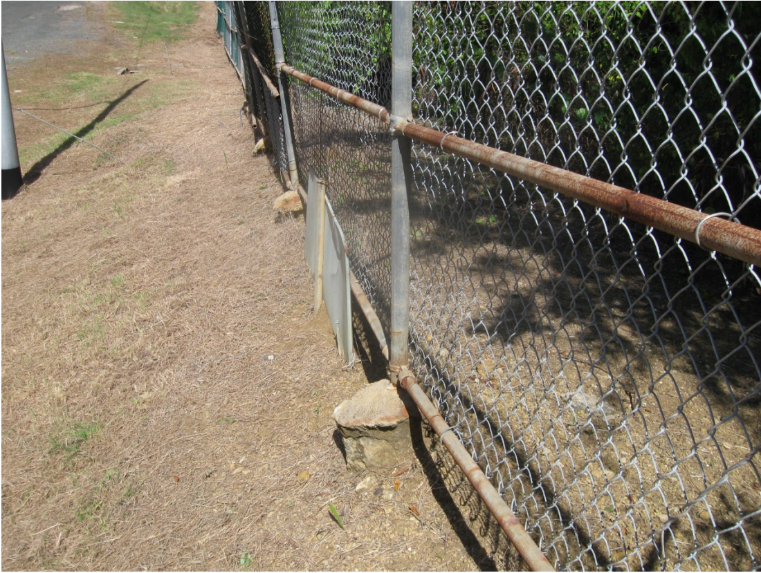
BON 8/2013. PL-11. Looking west down north fence line.
