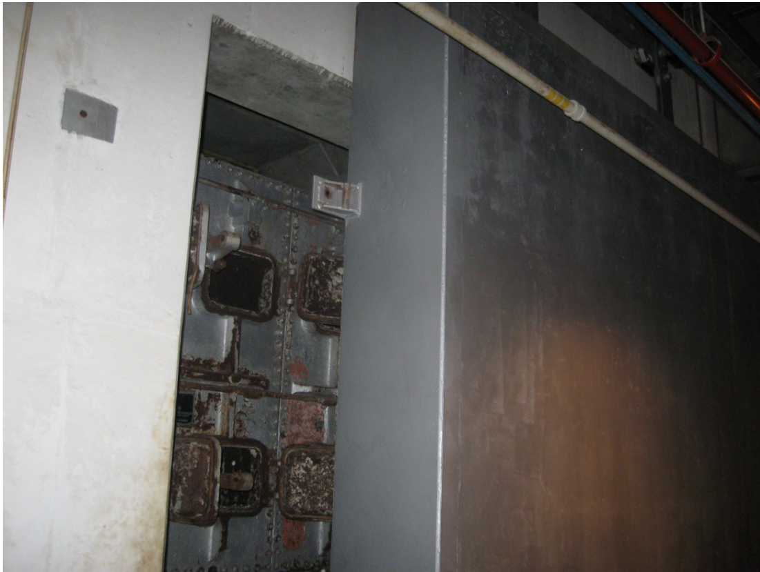
BON 8/2013. PL-7. Repainted surface to address underlying lead paint.
