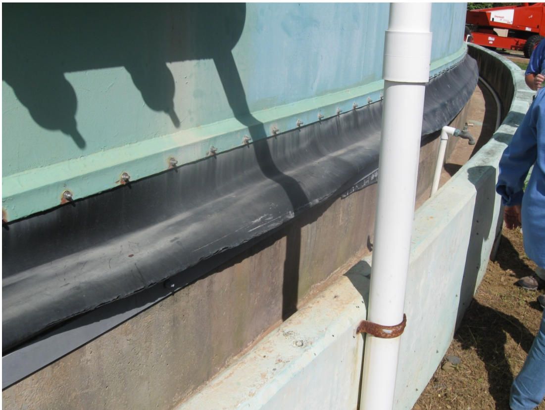
BON 8/2013. PL-4. Repairs to seal around base of dome.
