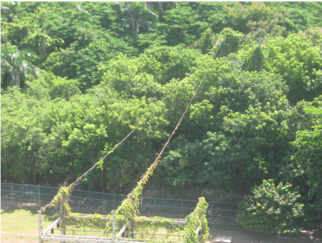
BON 8/2013. PL-14. Top of dome, looking northeast.
