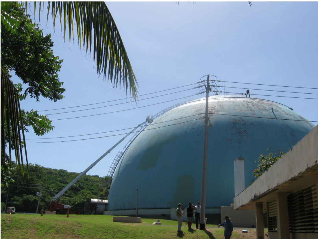
BON 8/2013. PL-2. Extended bucket lift to top of containment dome.
