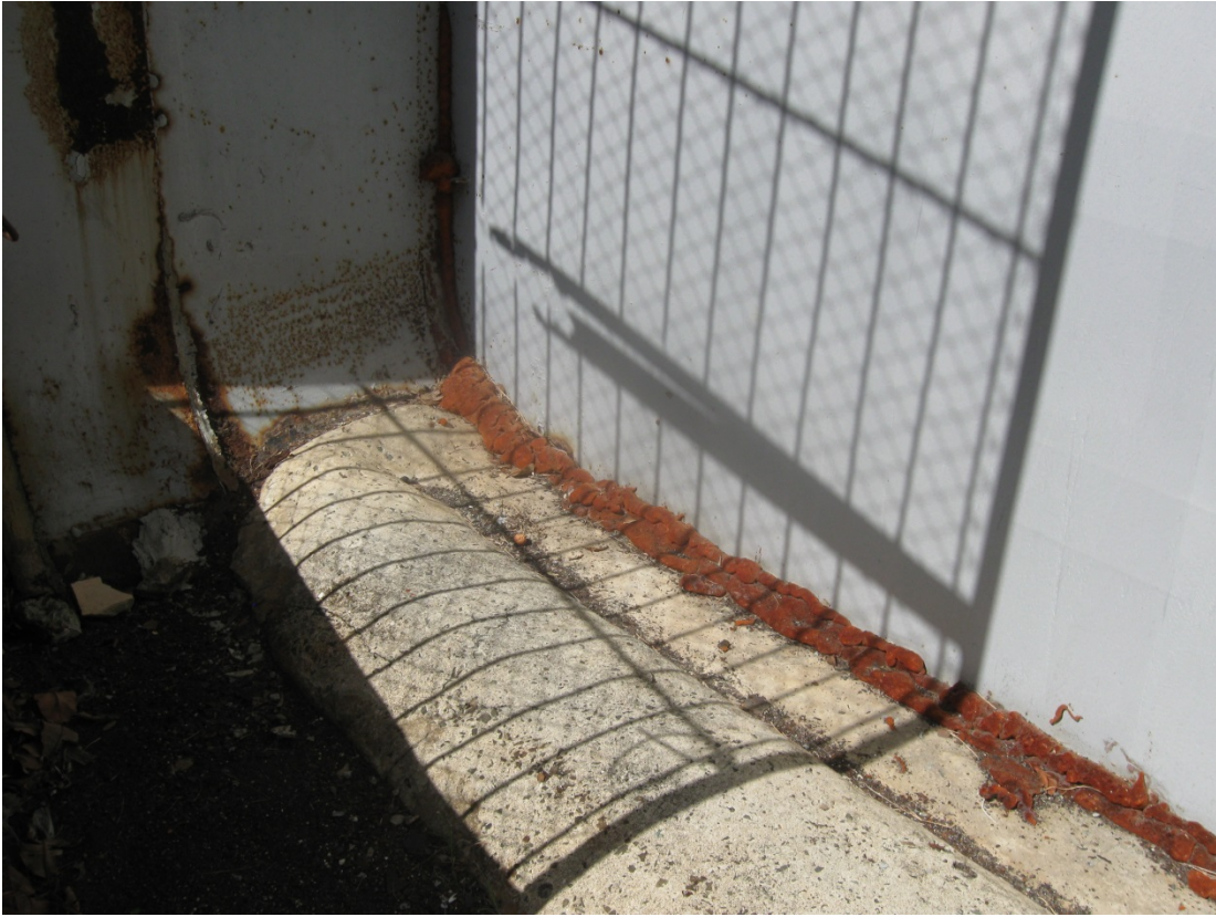
BON 8/2013. PL-9. Freight door, east side of containment building.
