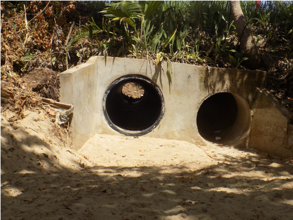
PL-13. Drain culverts
