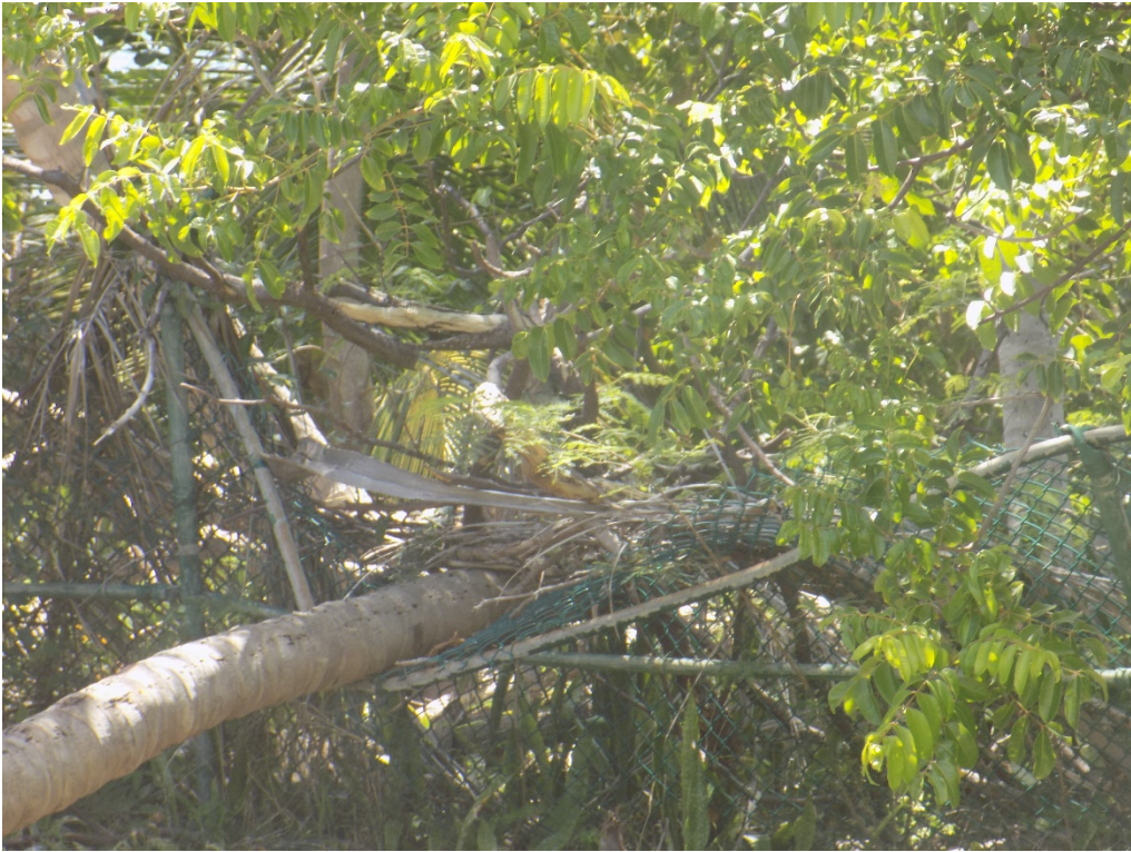
PL-6. Downed tree on security fence
