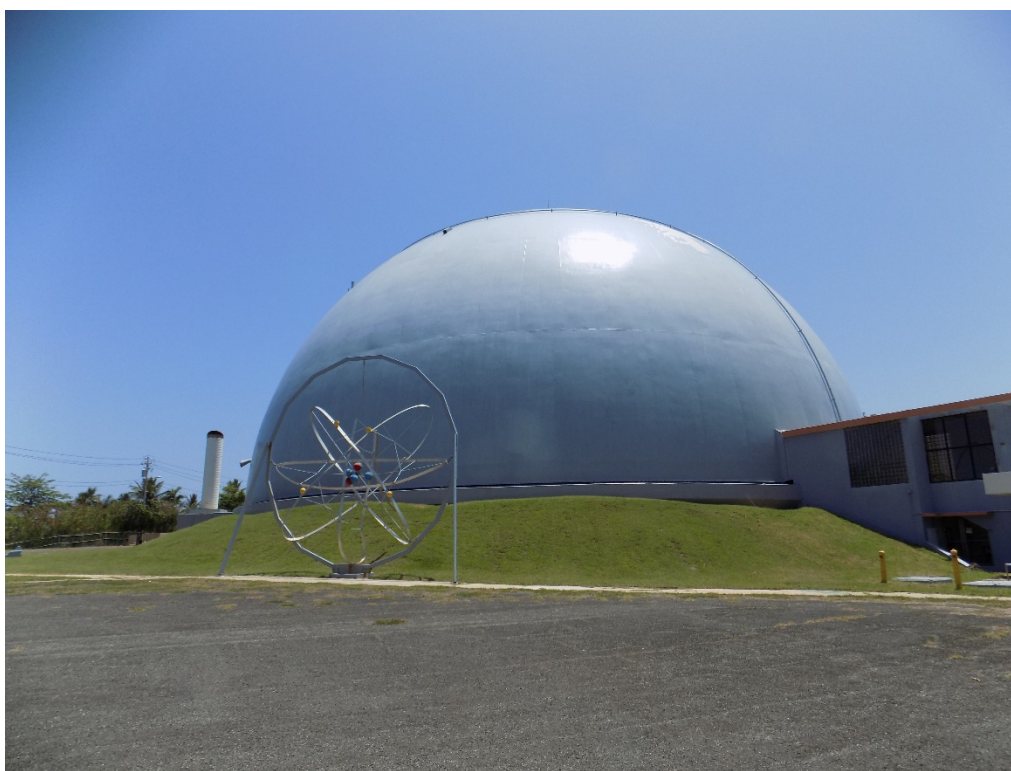
PL-1. Containment dome
