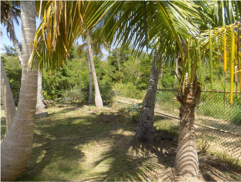
PL-8. Downed tree on security fence
