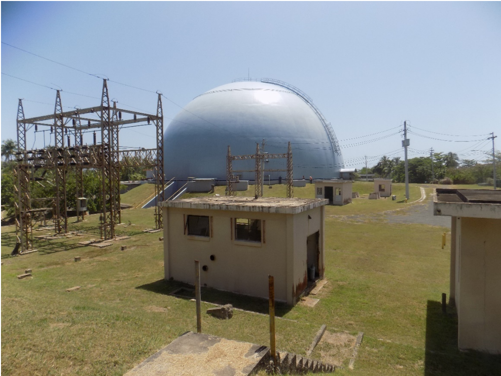
PL-11. Containment dome
