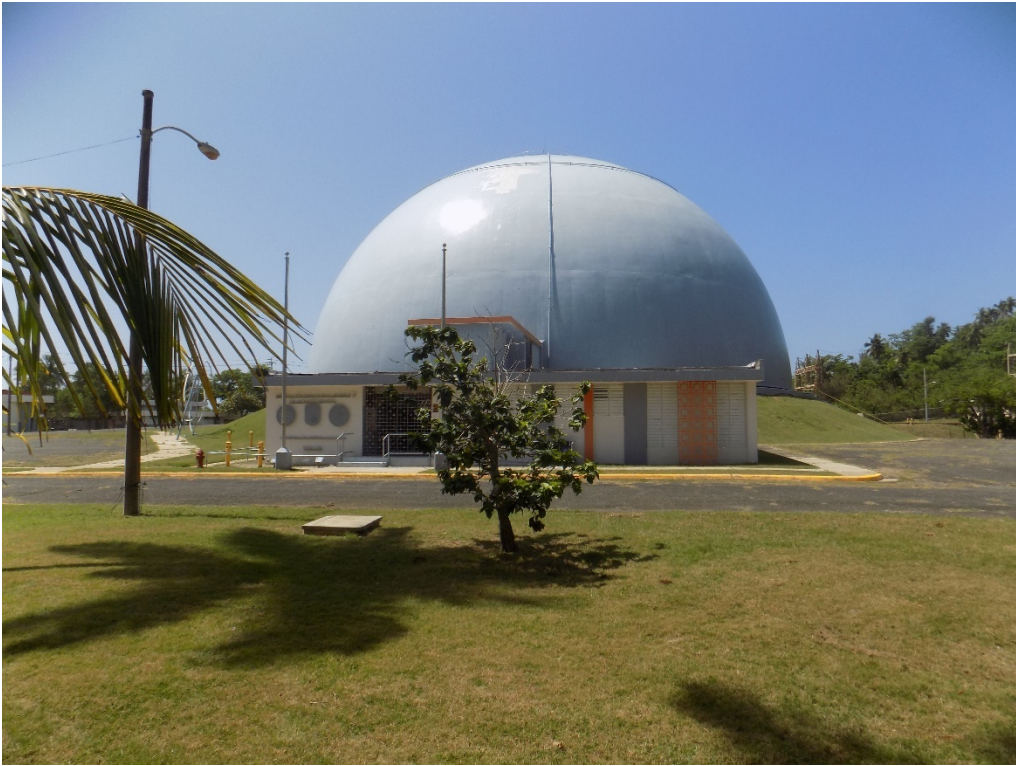
PL-12. Containment dome
