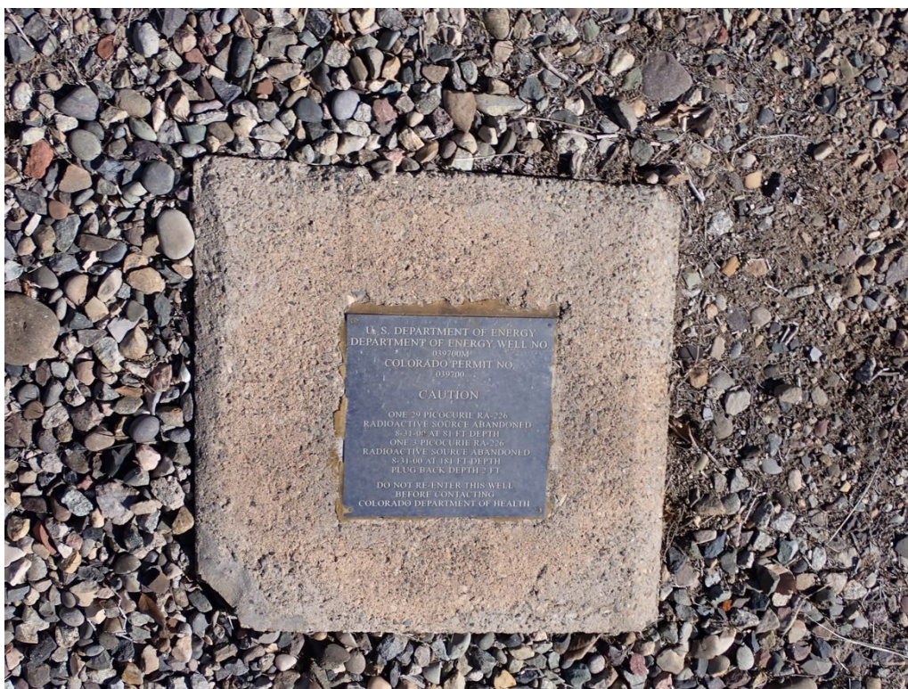
PL-8. Decommissioned Well Containing Radium Foil
