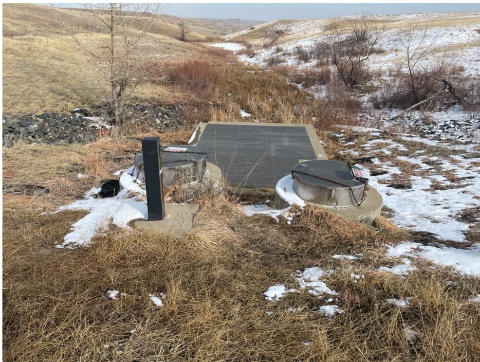
Figure 6. Looking East-Northeast at the Present Landfill Treatment System, Which Was Functioning Properly. Small amounts of Bio-growth were removed from the North and South Manhole Outlet Pipes, treatment unit outlet pipe, and system outfall using a mechanical pipe cleaner as part of routine preventative maintenance.
