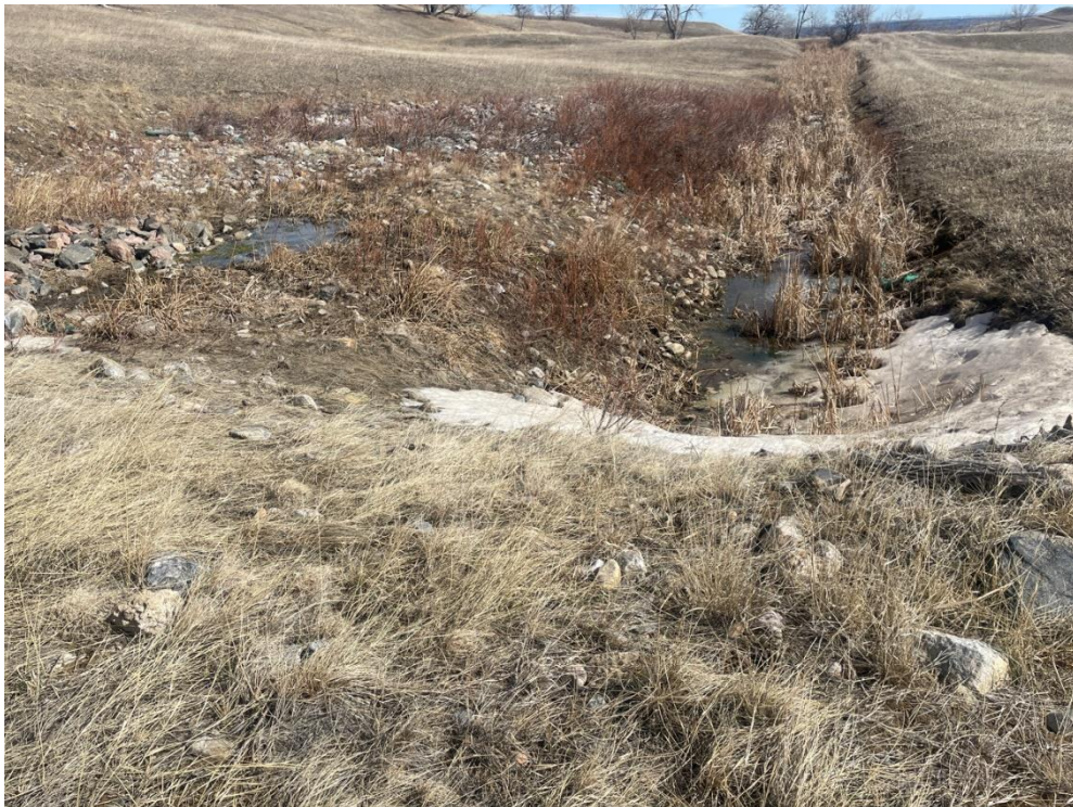
Figure 9. Looking East at the SID, Which Receives Groundwater from the ESSD Outfall and an Interceptor Drain on the Eastern Hillside and Had a Flow of 1–2 gpm
