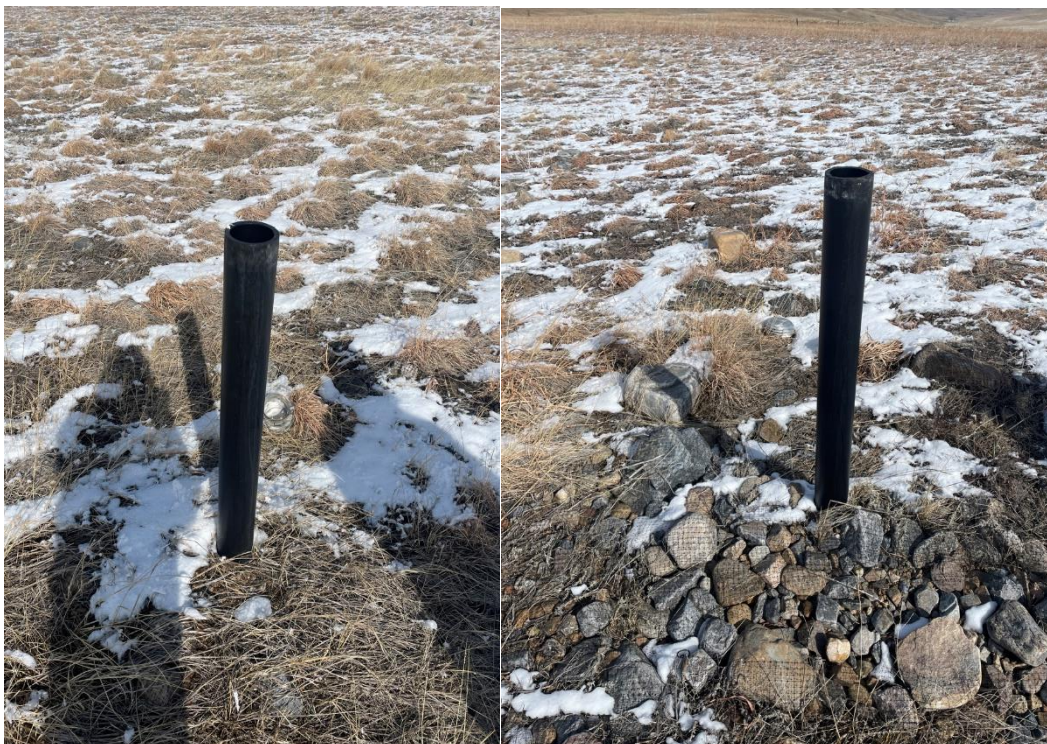
Figure 4. Looking at two Barometric Gas Vents, where the Vent Caps Needed to Be Reattached
