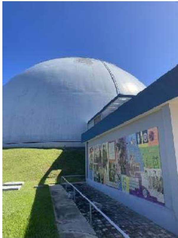
PL-2. Paint on Dome Damaged
