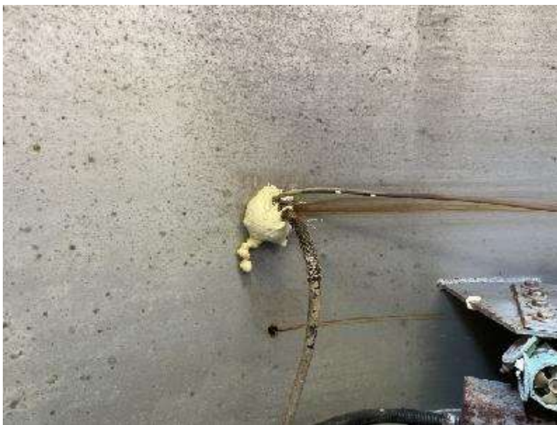
PL-1. Hole in Airlock 2 Sealed
