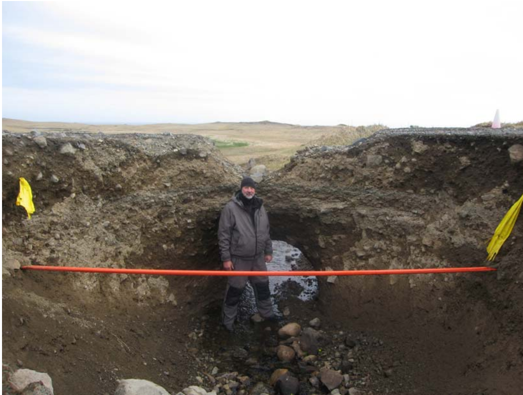
Figure 8. Infantry Road Washout near MM 8
