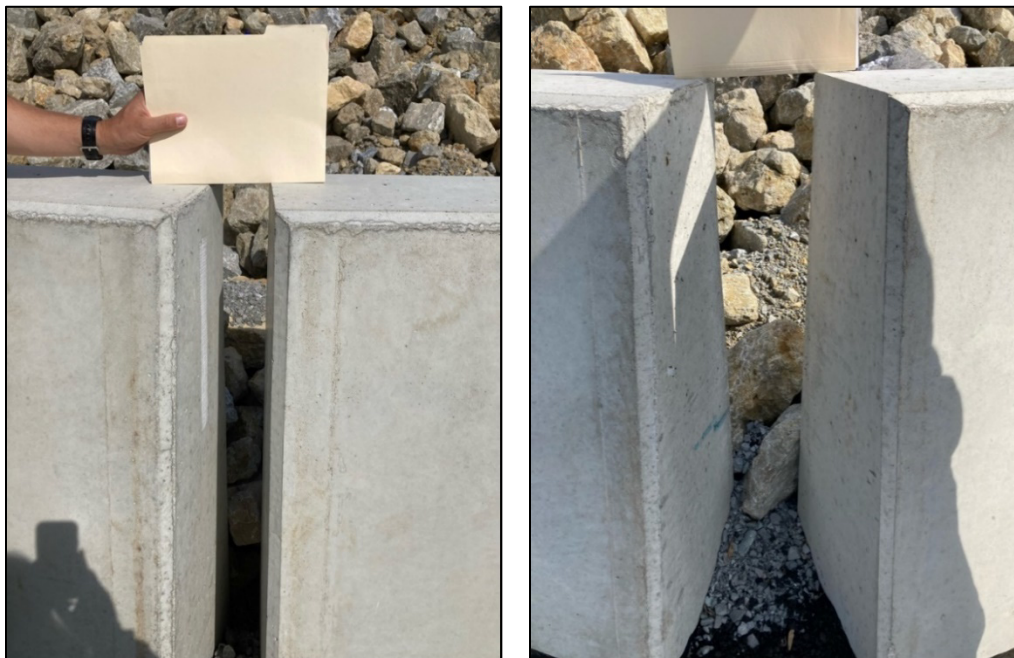
Figure 3. Examples of Spacing Between Protective Jersey Barriers Observed in 2024 and 2025
