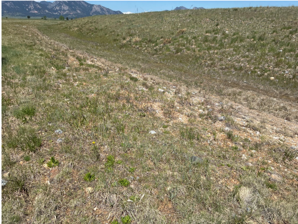
Figure 1. Looking West-Northwest at the Southern Vegetation-lined Perimeter Channel, Which Was in Good Condition.
