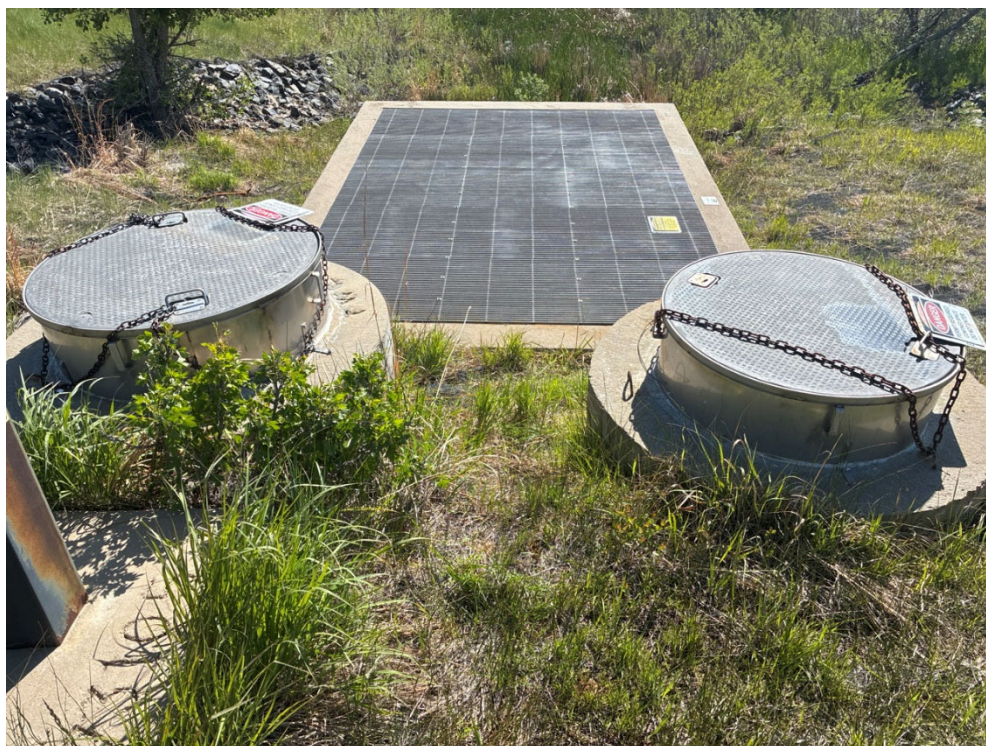
Figure 6. Looking East at the Present Landfill Treatment System, Which Was Functioning Properly. Small amounts of Bio-growth were removed from the North and South Manhole Outlet Pipes, treatment unit outlet pipe, and system outfall using a mechanical pipe cleaner as part of routine preventative maintenance.
