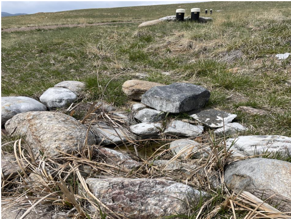
Figure 8. Looking Northwest at the ESSED, Which Had a Flow of Less than 1 gpm. Approximately 1 inch of sediment was observed at the outfall but was not disrupting flow.
