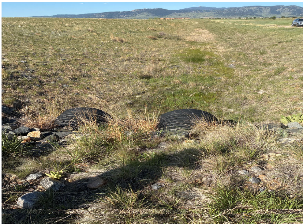
Figure 4. Looking Southwest at Culverts in the Northern Vegetation-lined Perimeter Channel, Which Were in Good Condition and Functioning Properly
