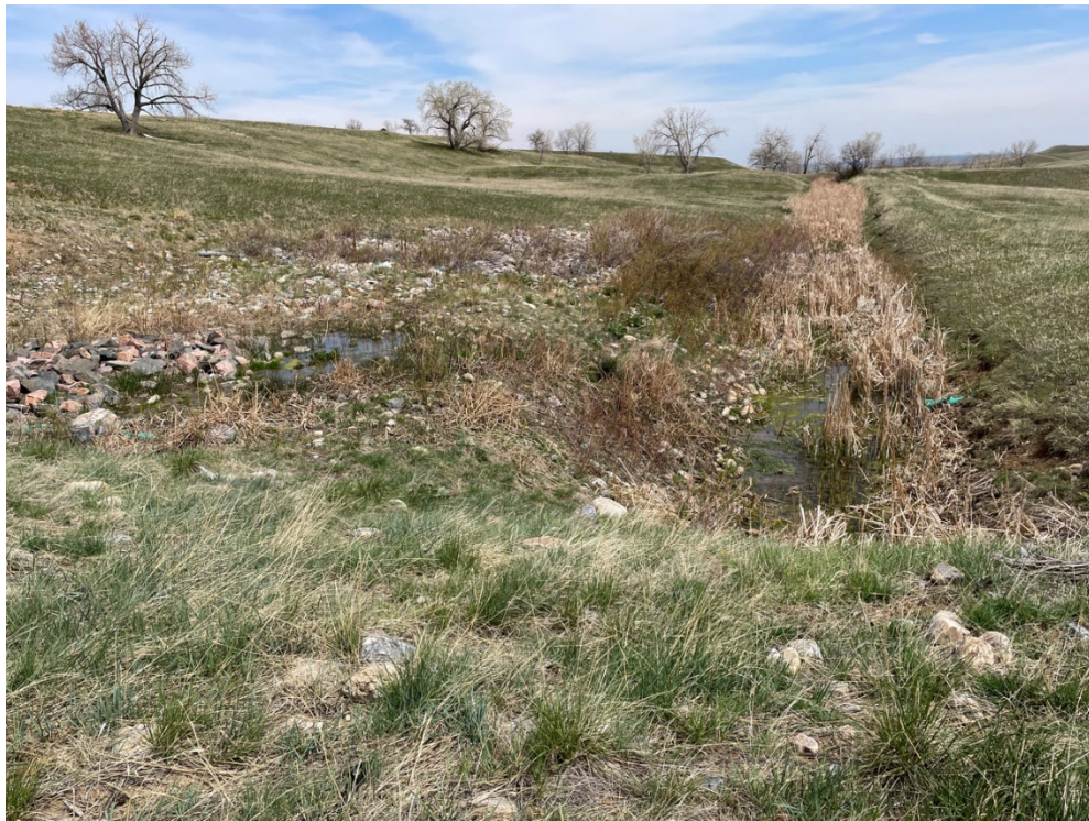
Figure 10. View Looking East at the SID, Which Receives Groundwater from the ESSD Outfall and an Interceptor Drain on the Eastern Hillside and Had a Flow Rate of Approximately 2–3 gpm
