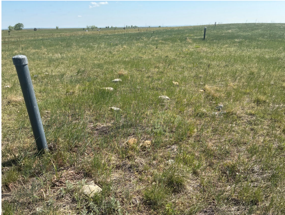
Figure 3. Looking East-Northeast at the Settlement Monuments and Barometric Gas Vents on the Cover, Which Were in Good Condition.
