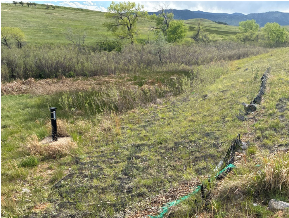
Figure 8. View Looking West at the Seep 8 Location, Which Had a Flow Rate of Approximately 2–3 gpm
