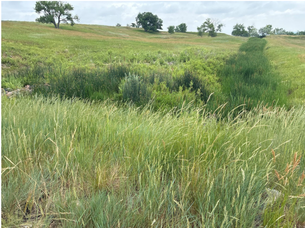
Figure 11. View Looking East at the SID, Which Receives Groundwater from the ESSD Outfall and an Interceptor Drain on the Eastern Hillside and Had a Flow Rate of Approximately 1–2 gpm
