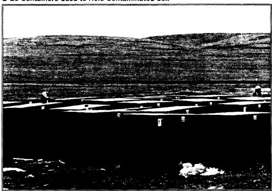
Figure 2-4 B-25 Containers Used to Hold Contaminated Soil
