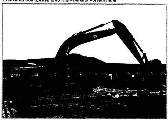
Figure 6-6 Excavated Soil Spread onto High-Density Polyethylene
