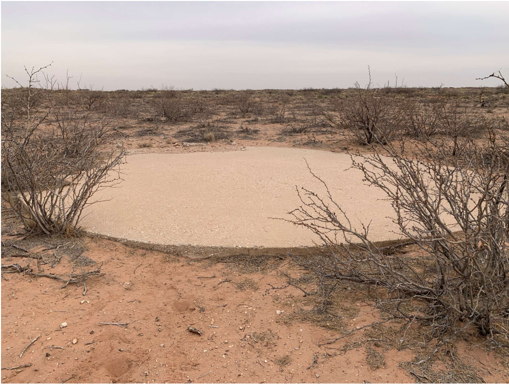
Photograph A-3. View Looking South at the Concrete Cap that Covers the Project Gnome Emplacement Shaft
