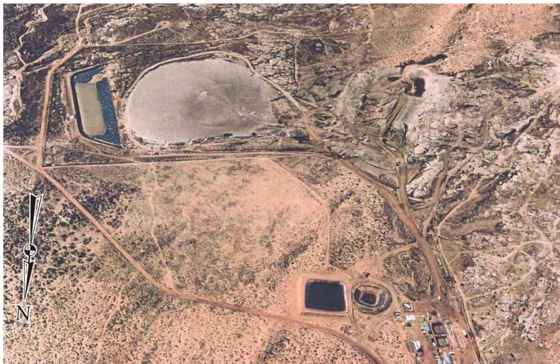
Figure 2–5. Contaminated Excavation and Haul from the Heap-Leach Area Prior to New Tailings Pile and Evaporation Pond Excavation (March 1993)
