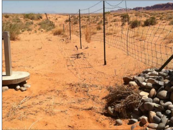
Erosion at well 0734 and nearby fencing.
