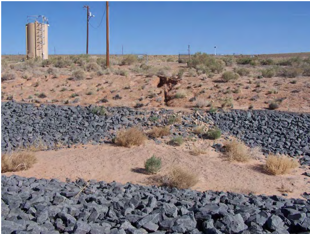
TUB 4/2008. PL-4. Gully erosion and sediment deposition in the diversion channel near distillate tank.
