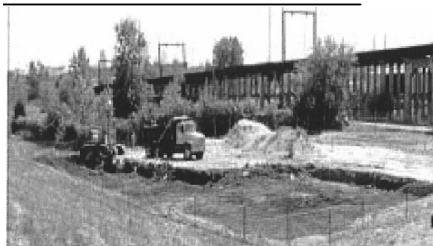
Crews remove material from the Plant 7 East site in St. Louis.
