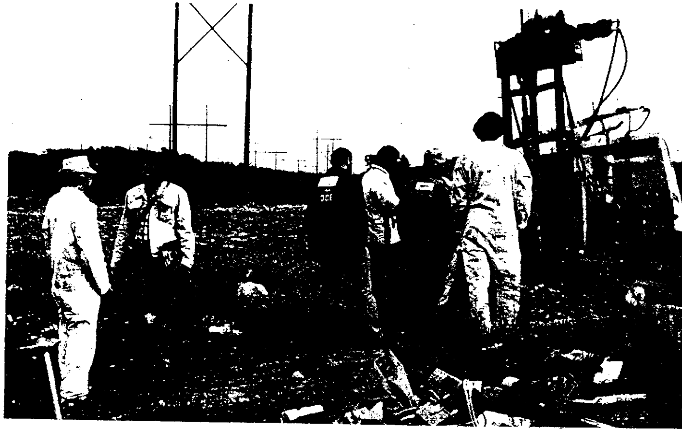
DRILLING FOR HAZARDS: State and federal investigators drill for core sample of dump site near Norton/Attleboro town line.
