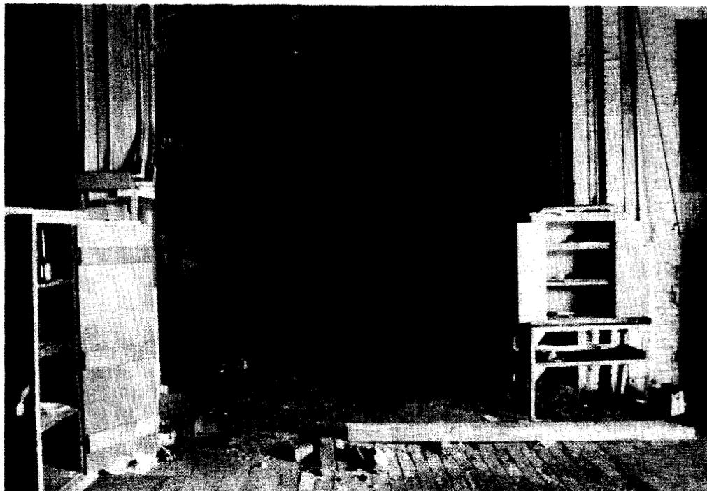
**Fig. 23. View of brick facing on column B2 (right side of photo behind cabinet). Chips of the brick facing material contained 900 pCi/g  $^{238}\text{U}$ .**
