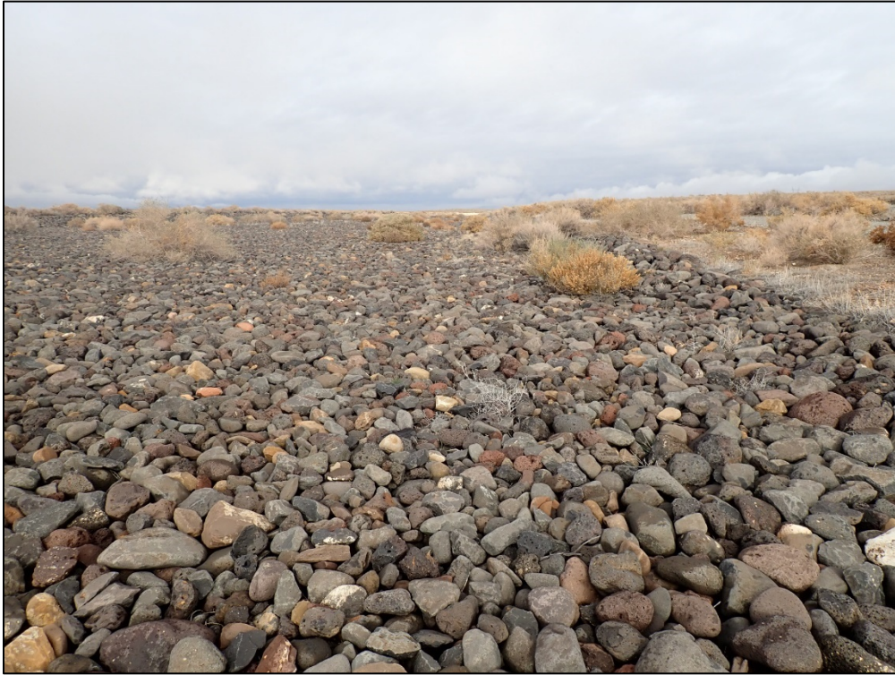
PL-9. South Diversion Channel
