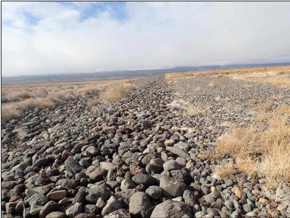
PL-8. Disposal Cell Top and Side Slope
