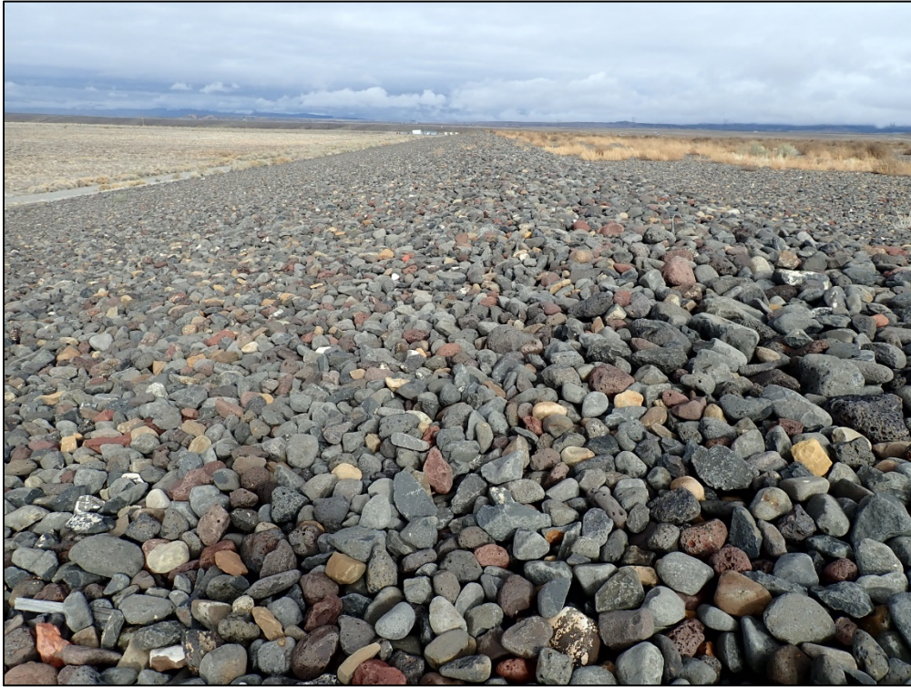
PL-7. West Side Slope Disposal Cell
