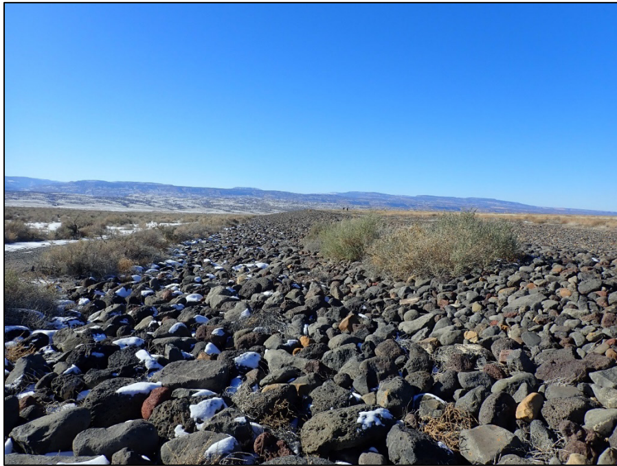
PL-8. South Side Slope of Disposal Cell
