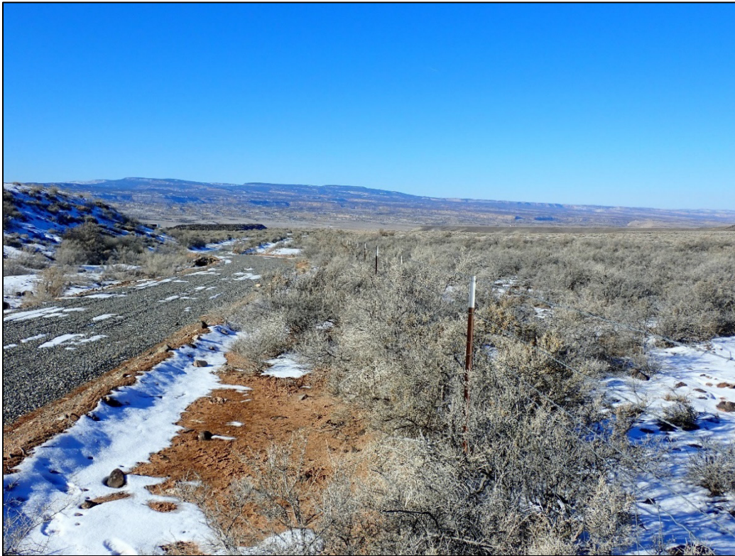
PL-3. North Perimeter Fence
